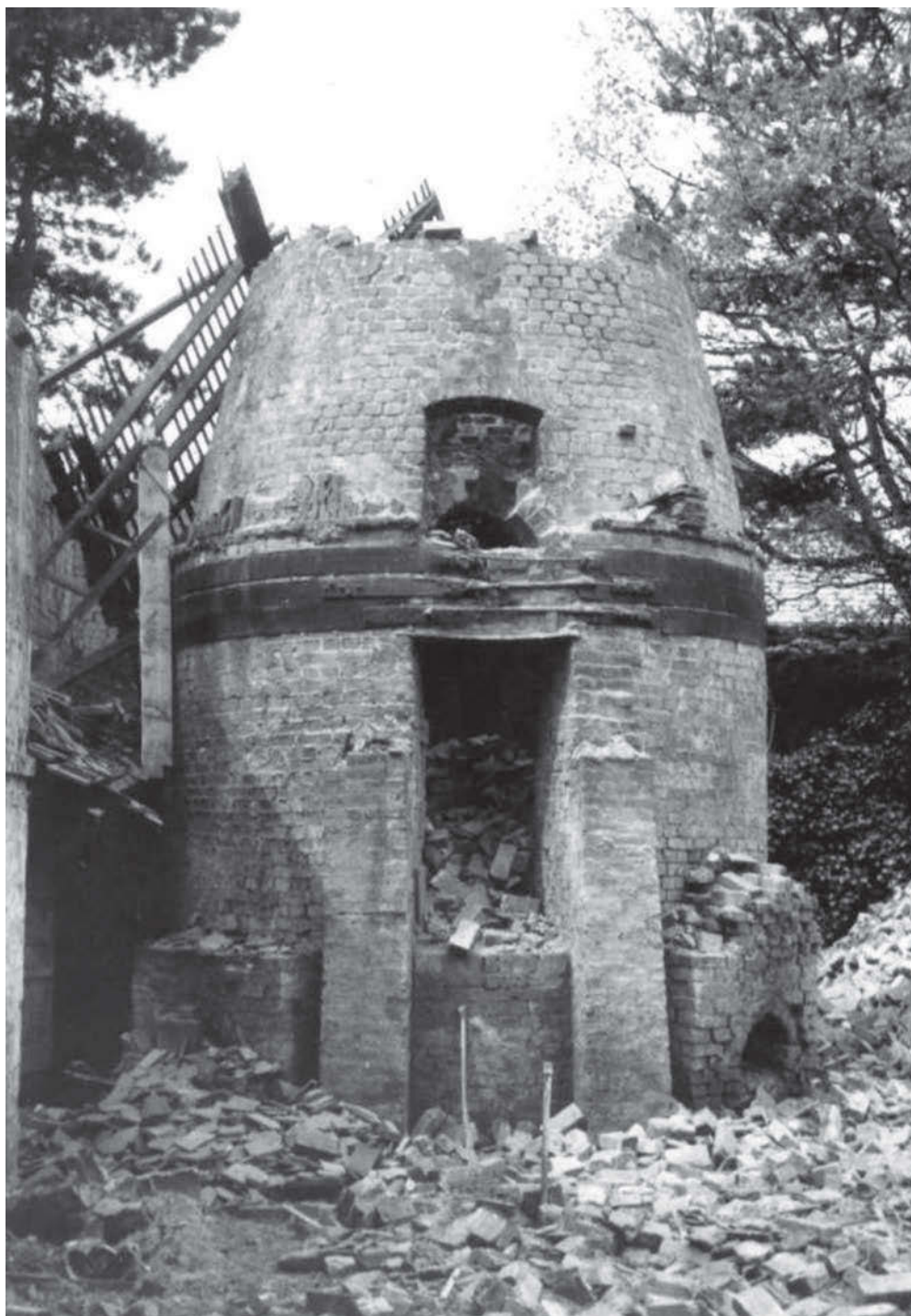
Fig. 5. Photograph of the bottle kiln during demolition in 1971 viewed from the east (courtesy of East Grinstead Museum Collection).
