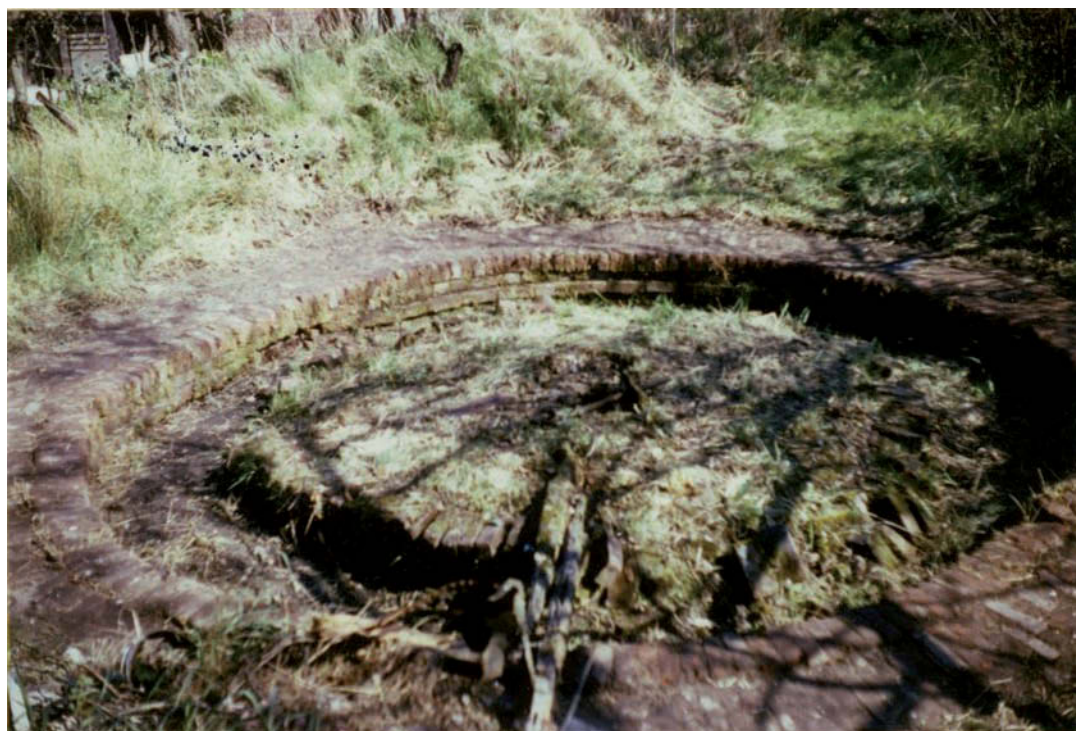
Fig. 9. Photograph of the 'horse gin' from the East Grinstead Pottery showing the inner and outer brick structures around a trough that held unprocessed clay (courtesy of East Grinstead Museum Collection).
