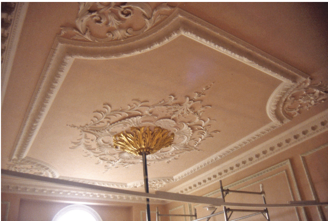
Fig. 45. The restored ceiling in the Stairs Hall.
