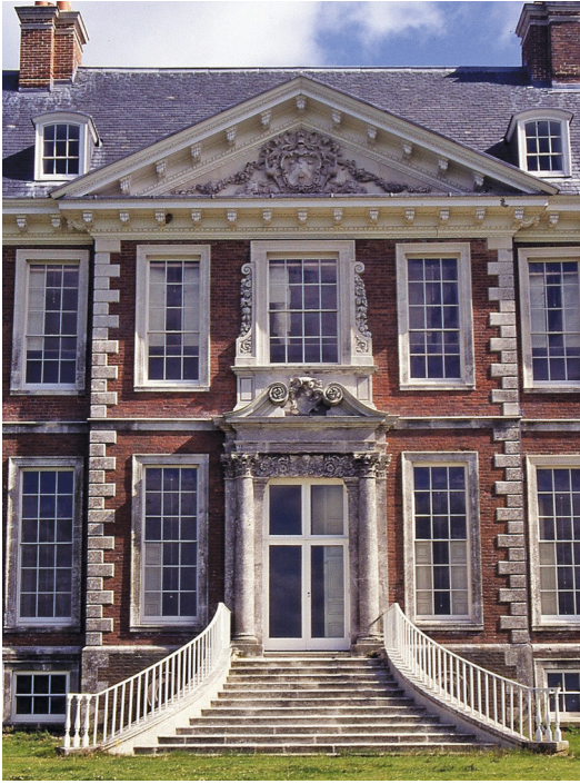
Fig. 13. Detail of the south front, after restoration.
