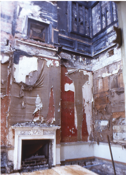
Fig. 27. The Small Drawing Room and part of the bolection panelling in the Prince Regent's Bedroom above it, after the fire.
