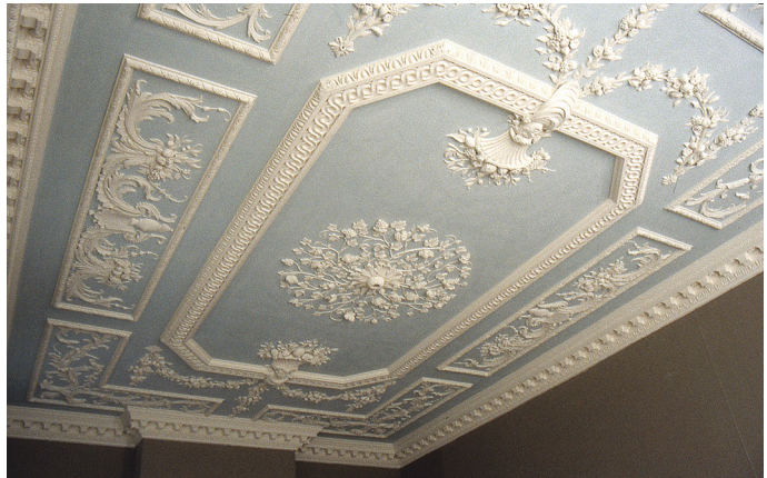
Fig. 43. The restored ceiling in the Red Drawing Room, prior to gilding.
