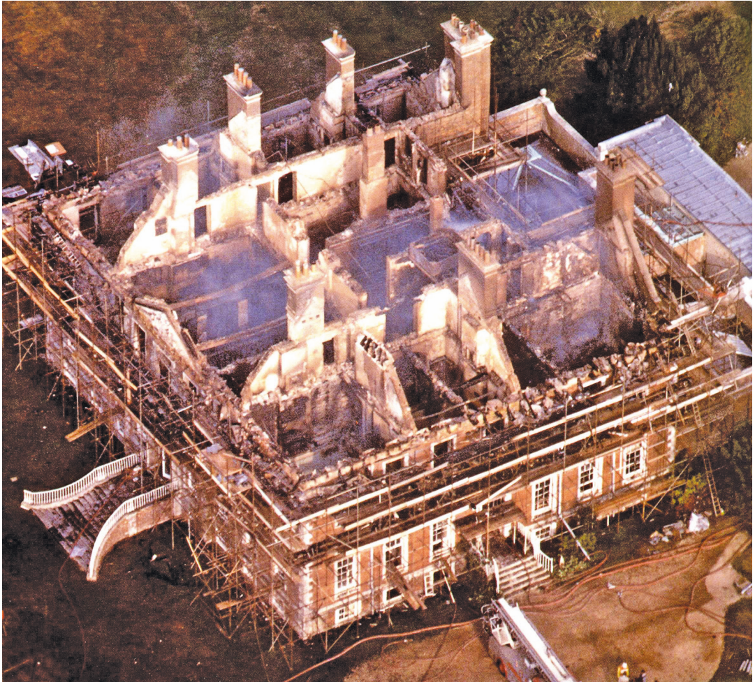
Fig. 1. The house after the fire in August 1989. Photograph by courtesy of Portsmouth Publishing and Printing Ltd.
