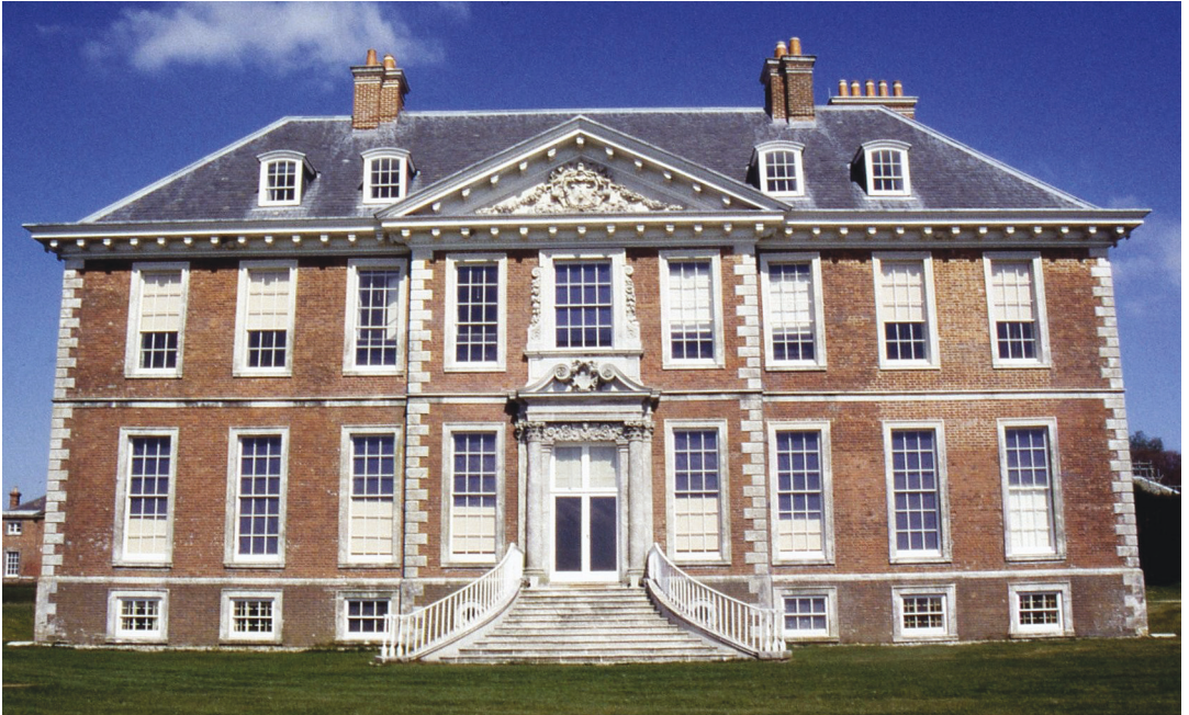
Fig. 11. The south front, after restoration.
