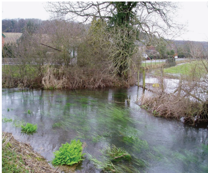
Fig. 13. Winter flood conditions at the junction of the East and West Ems at Walderton Bridge, 100m from the pumping station. (D. Dunkin.)
