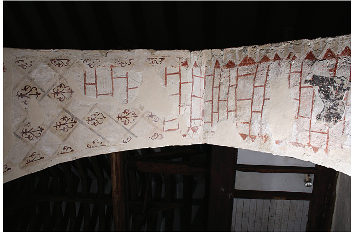
Fig. 15. Soffit of E. arch of S. nave wall, with masonry pattern [B] overlaid with later patterning [E].
