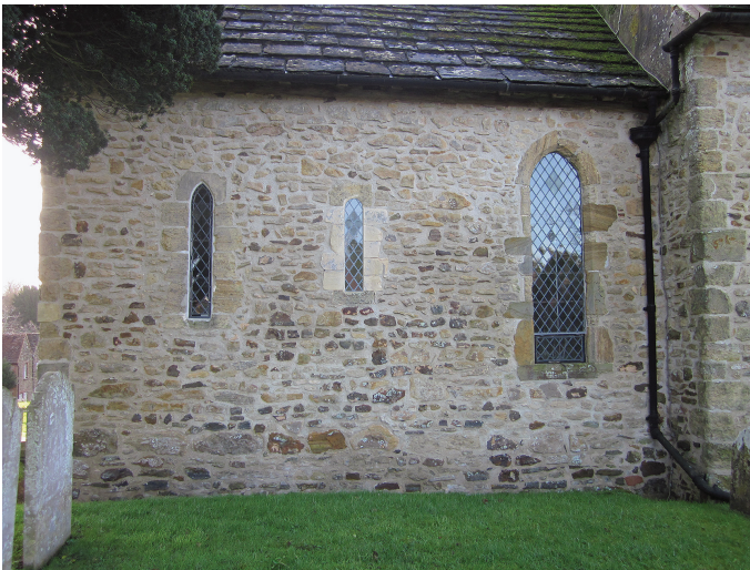
Fig. 8. On the north wall of the chancel there are three windows. The smaller central window is of Norman character and probably replaces an earlier Anglo-Saxon window. There are traces of this earlier window where Pulborough Stone remains in use, but most of the window is now built of Caen Stone.
