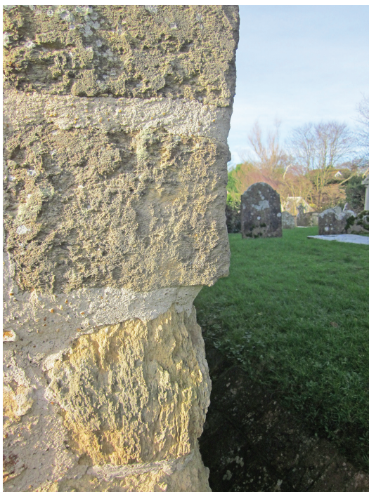
Fig. 5. Stones 4 (top only), 5, 6, and 7 of the north-east chancel quoin are of Pulborough Stone, here sufficiently enlarged to read something of their Anglo-Saxon orientations as BVFL , BVFR (the most obvious), BH , BH .
