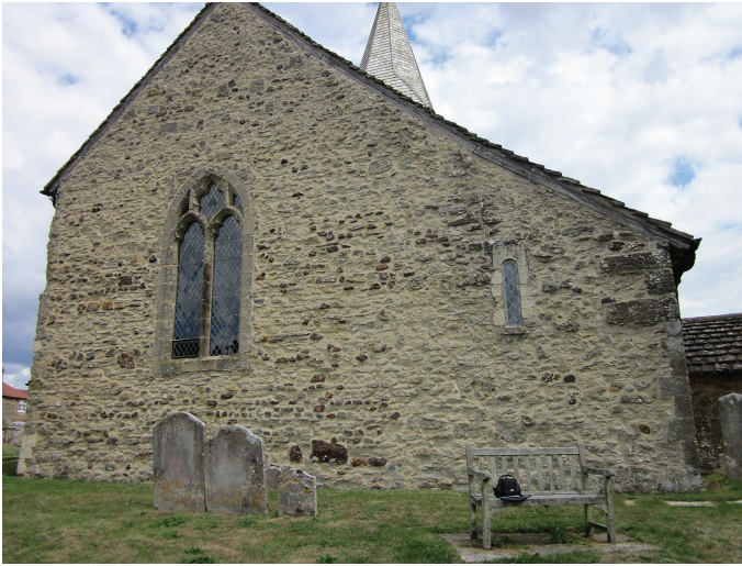
Fig. 7. The west faces of the nave and south aisle at West Chiltington. Only the top three quoin stones of the south-west nave quoin remain. The darker stones in the Hythe Beds walling are mainly of Folkestone iron-rich sandstone. The aisle west window is largely created in Caen Stone in Norman style, and the darker patch of iron-rich sandstones above and to the north of the window marks the position of the one-time gallery doorway.
