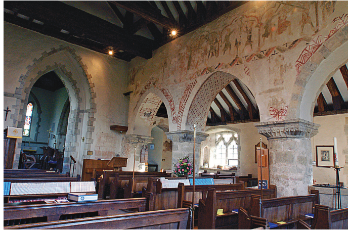
Fig. 19. Nave interior from NW towards chancel arch.
