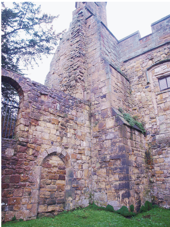
Fig. 15. Remains of St John's gate-chapel, from the north-east.
