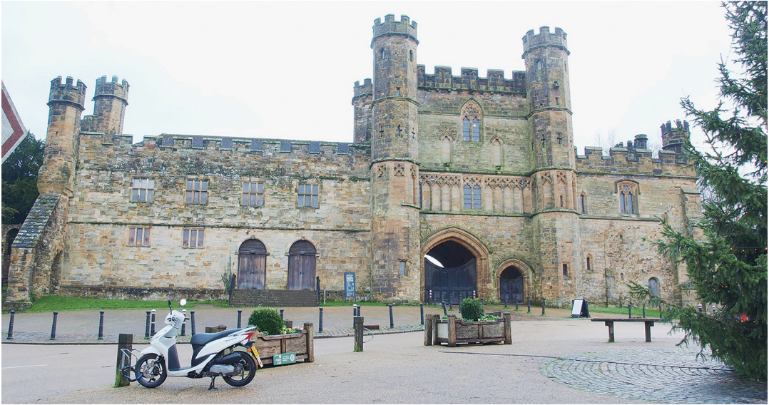
Fig. 2. General view of the Great Gatehouse from the north.
