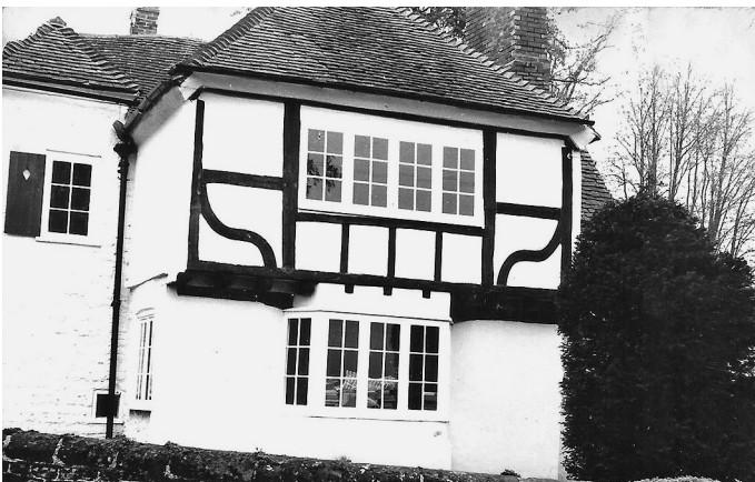
Fig. 3. The cross wing after renovation showing the ogee braces (WDOAM).
