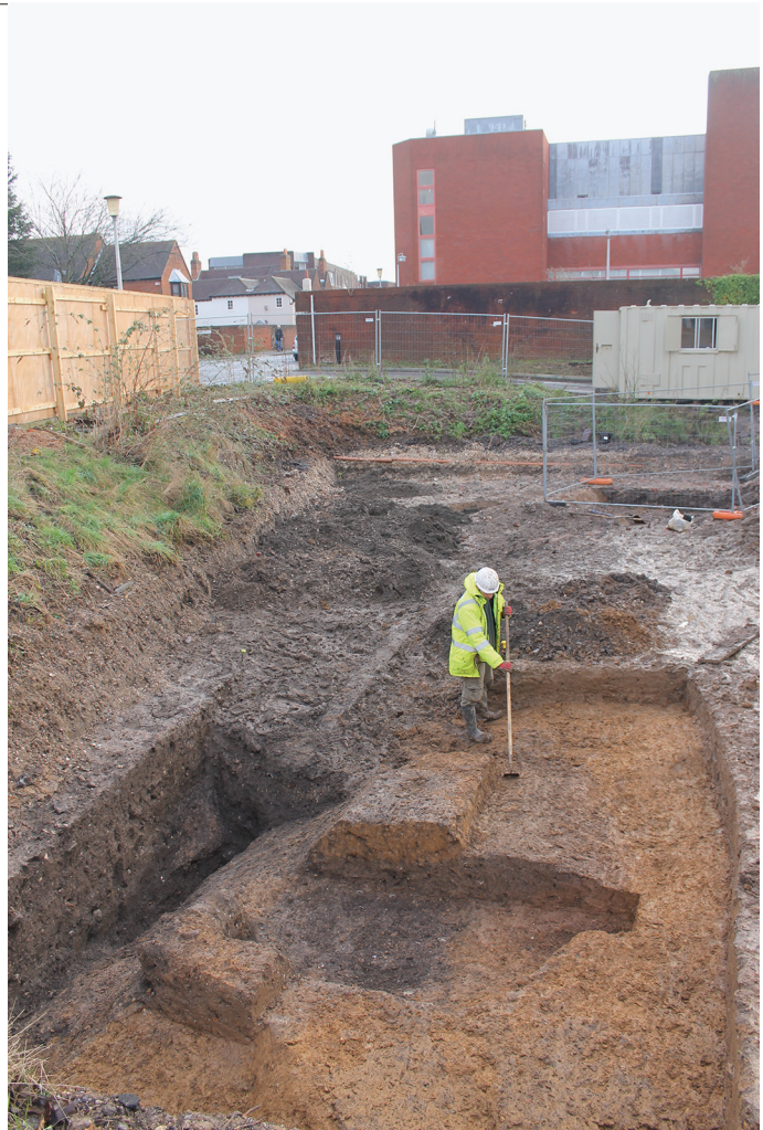
Fig. 9. The sewer ditch [6/006] facing east.
