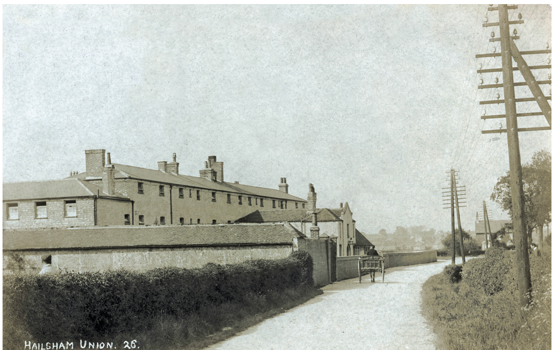
Fig. 1. Hailsham Union Central Workhouse, built in 1836 (by permission of Peter Higginbotham Collection/Mary Evans Picture Library)
