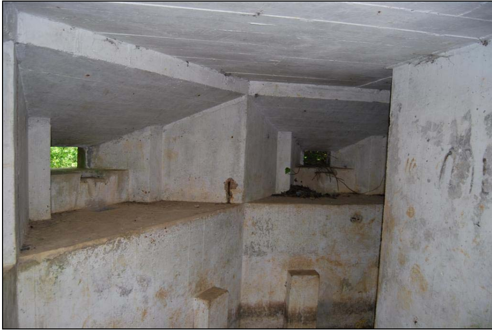
Plate 3: Internal View of Loopholes
