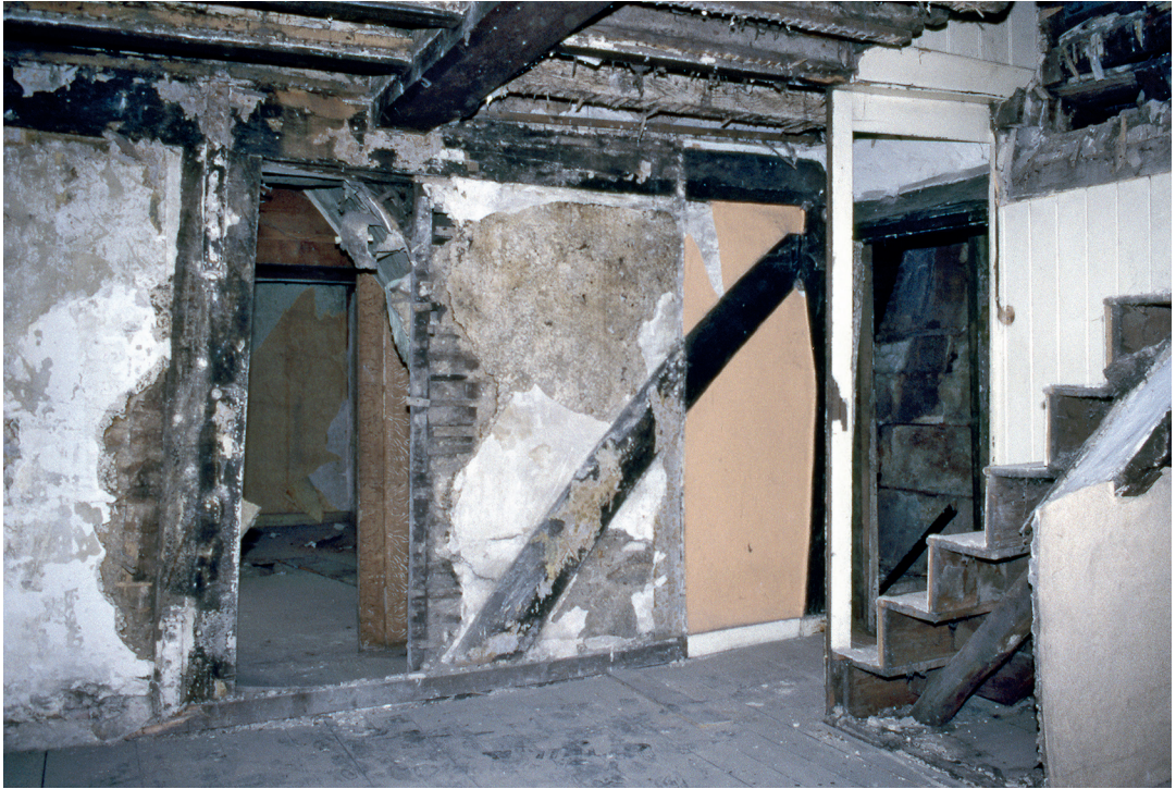
Fig. 10. Truss B-B: foot-brace to post B1 (right) and central stud (left).
