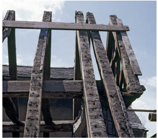
Fig. 24. Detail of projecting gable head.
