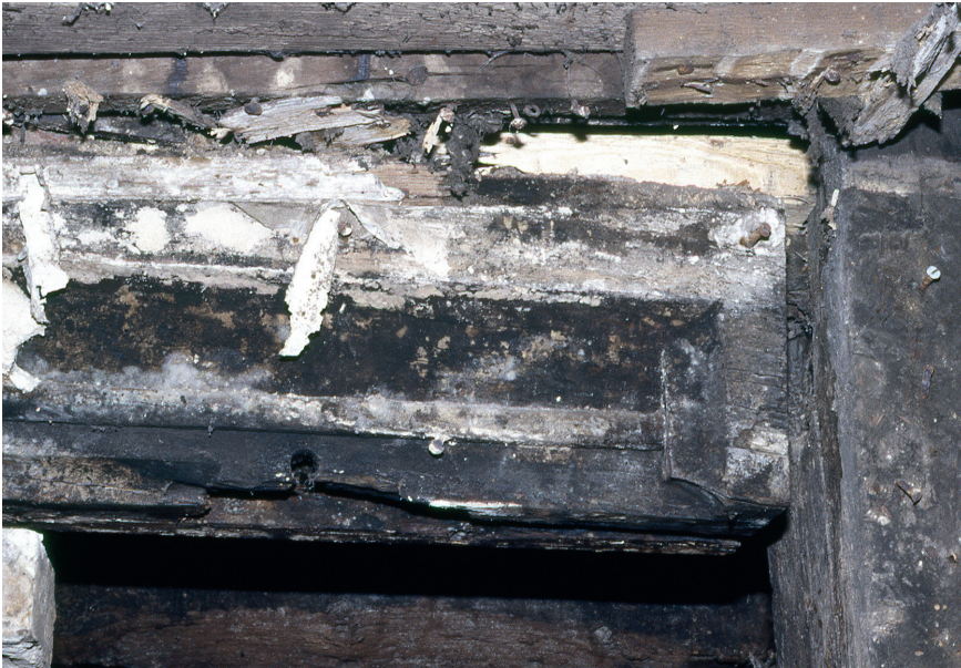
Fig. 14. Crossbeam truss B-B with principal post B1 to right.
