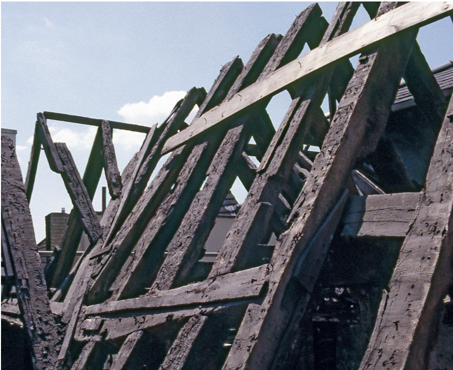
Fig. 26. Intersection of roof with that over main range (left). Note butted side-purlin to north (right) of principal rafter and butt purlin interrupting the common rafters to the south (left).
