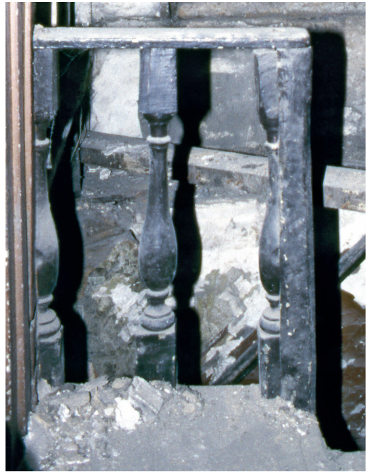
Fig. 23. Balustrade to first-floor landing.
