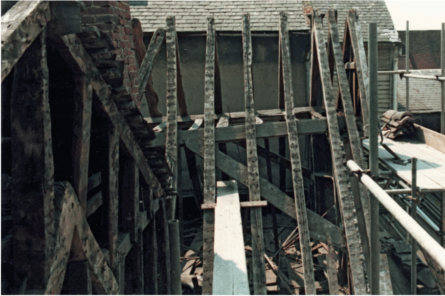
Fig. 25. North end of roof viewed from east.
