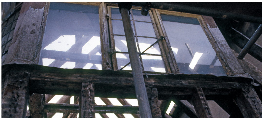
Fig. 22. Garret window at head of bay window.
