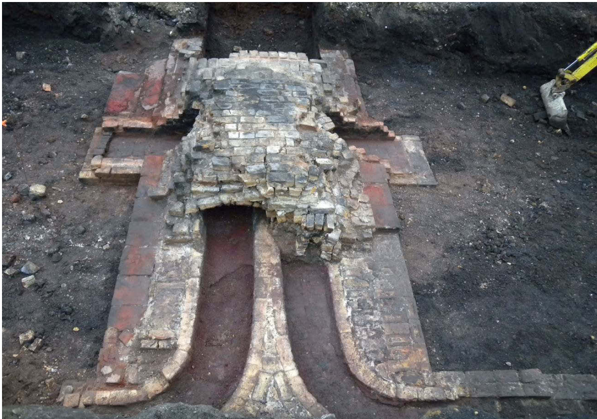
Trench 2 Structure [31], looking south-east (above) and north (below), showing parallel flues and brick floored chamber
