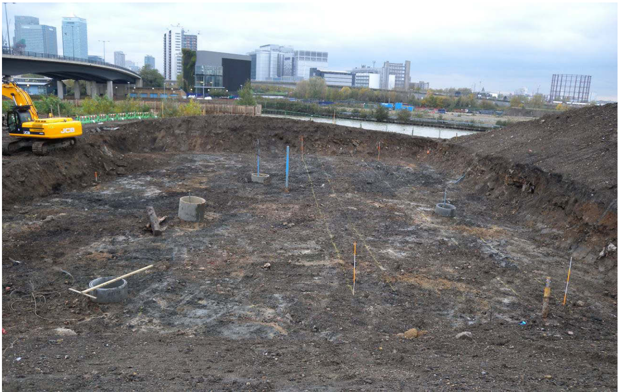
Area at Limmo Peninsula reduced from 107m ATD (7m OD) to 105m ATD (5m OD), looking west
