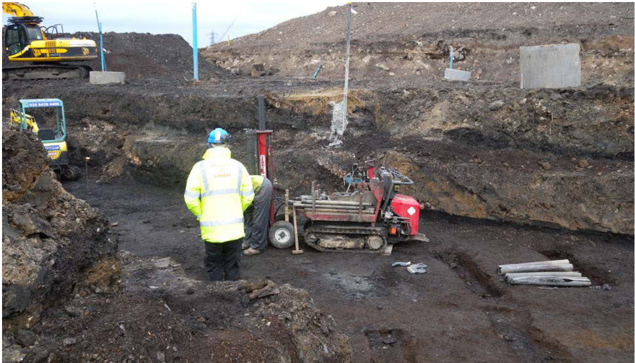
Trench 2 with terrier rig in operation, looking north-west
