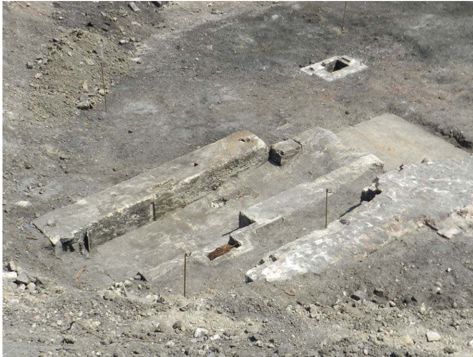
Photo 5 Concrete structure [98] - possible the base for a machine with a large wheel or drum. Drain [111] is in the background and wall [95] (the wall separating the machine and erecting shops) is at right. (Looking east)
