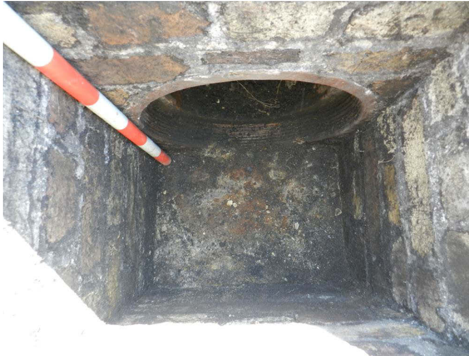
Photo 7 Drain [111]. (South-west at top of picture).
