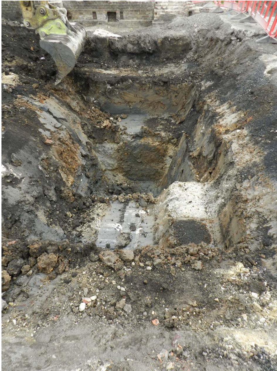
Photo 8 The stepped sondage. (Looking north-east)
