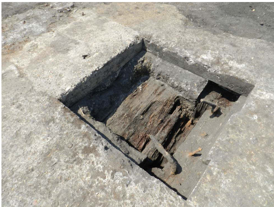
Photo 6 Concrete and timber structure [104/114] A possible hoist or crane base. (Looking north)
