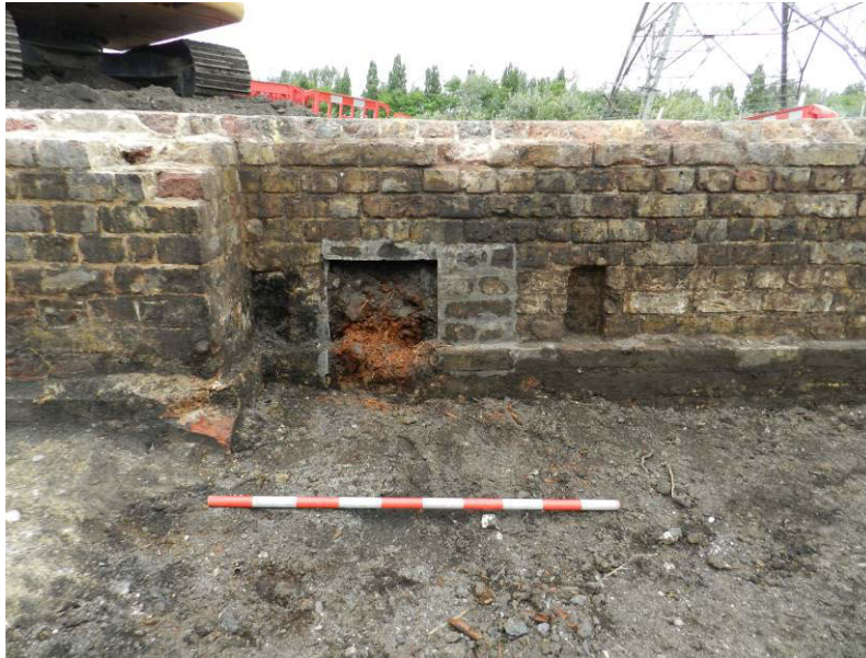
Photo 3 Recess for a possible floor. A portion of rotten timber remains in situ. (Looking north east)
