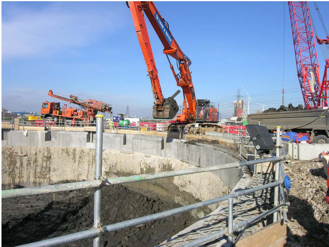
Photo 1 Main Shaft excavation
