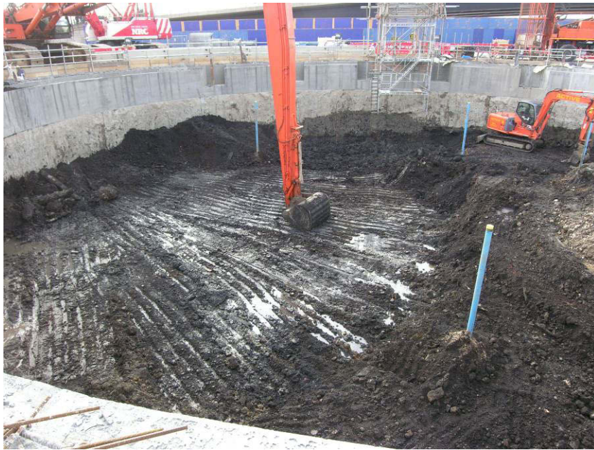
Photo 2 Main Shaft. Sterile estuarine alluvium between 102.0m ATD and 100.5m ATD below 19th-century clinker dumps. Looking east
