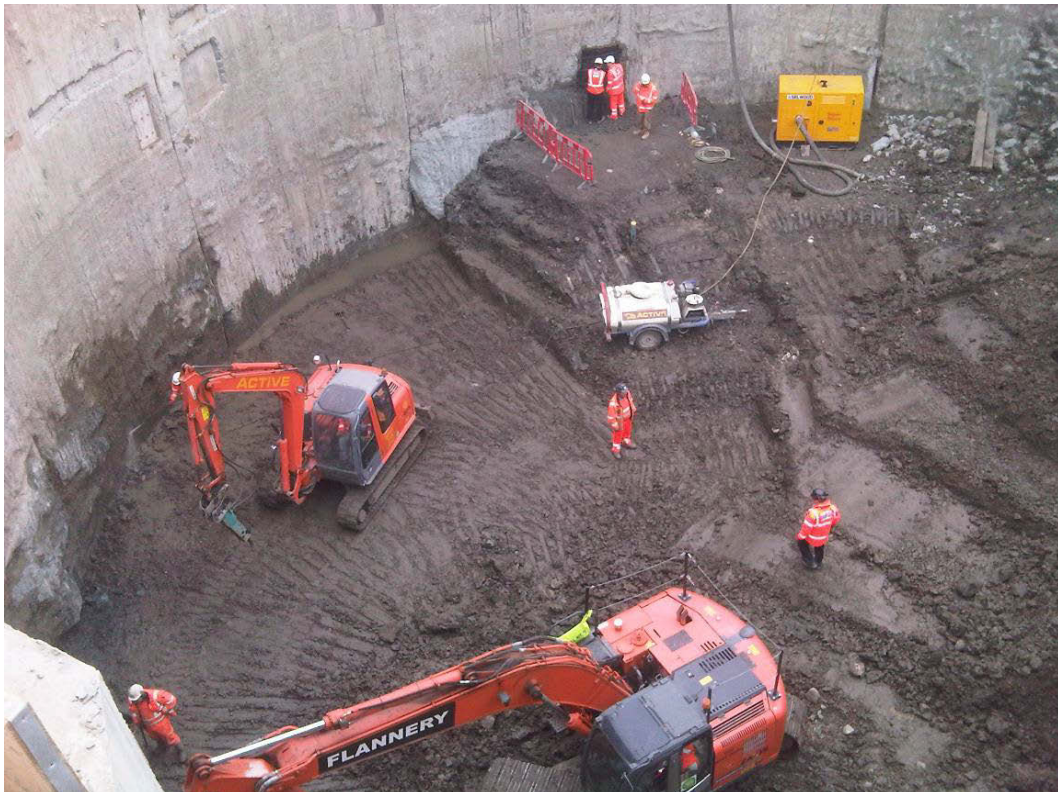
Photo 5 Main Shaft. Excavating the London Clay
