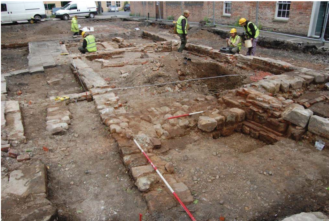
Ford Street/Friar Gate car park. 'Queen Anne House' and medieval foundations, E facing
