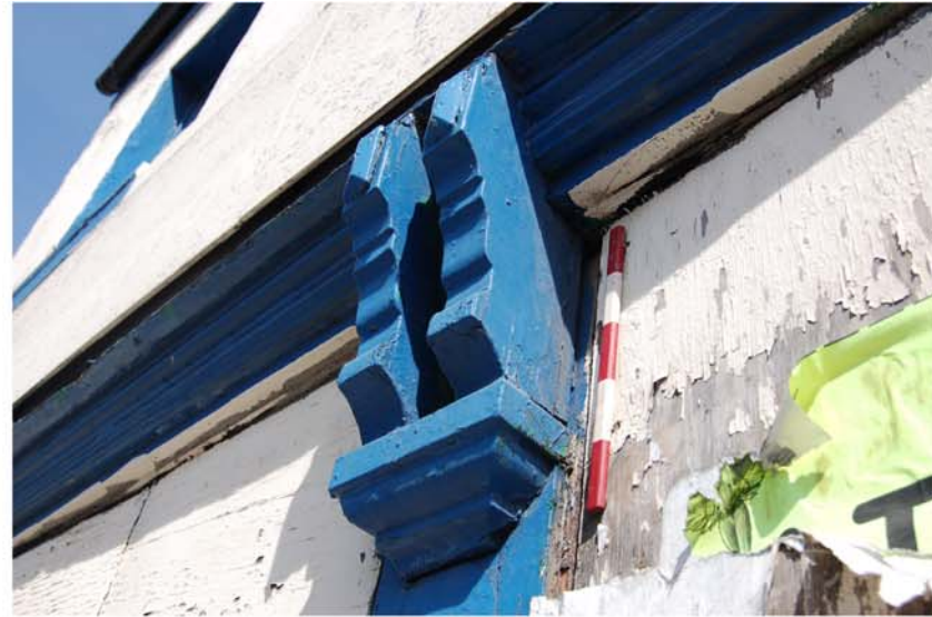
Plate 2: 5 Agard Street, cornice bracket from the southeast
