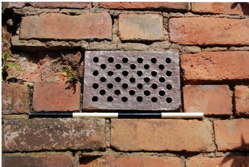
Plate 19: Wall between 71 King Street and the Seven Stars, air vent from the south
