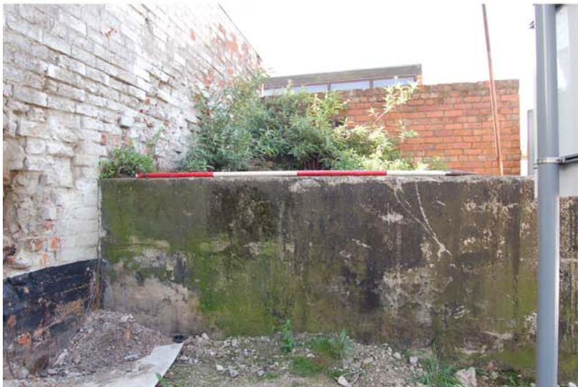
Plate 3: 5 Agard Street, concrete structure at the west end of the building
