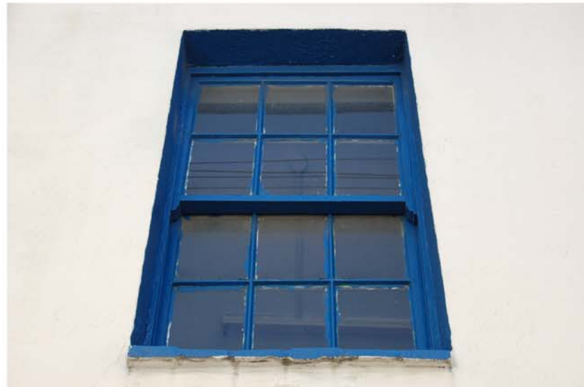
Plate 4: 5 Agard Street, first-floor window from the north
