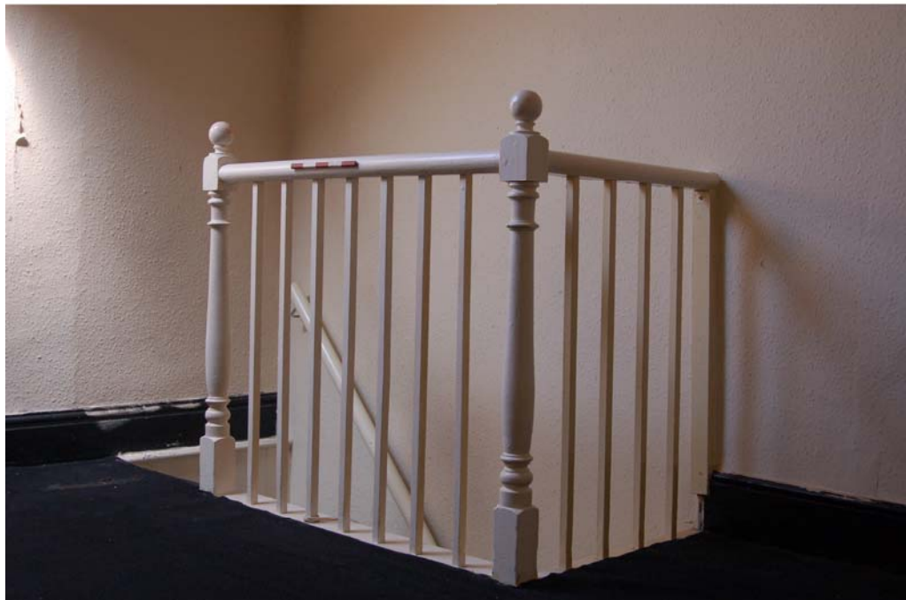
Plate 17: 35 Ford Street, S2, balustrade from the southeast
