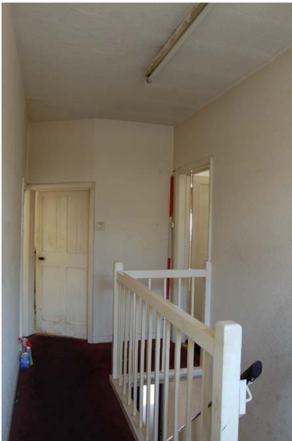
Plate 7: 5 Agard Street, F1 landing from the southwest
