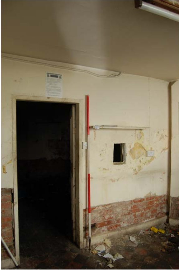
Plate 5: 5 Agard Street, G2, south wall from the northeast showing observation loop
