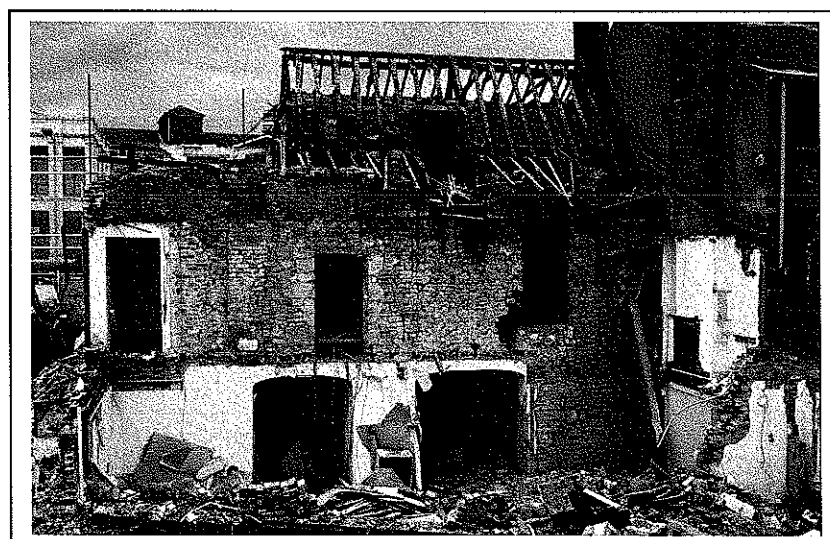
Plate 18 Early ironstone walls and timber roof incorporated in number 53 Bridge Street. Observed during demolition.
