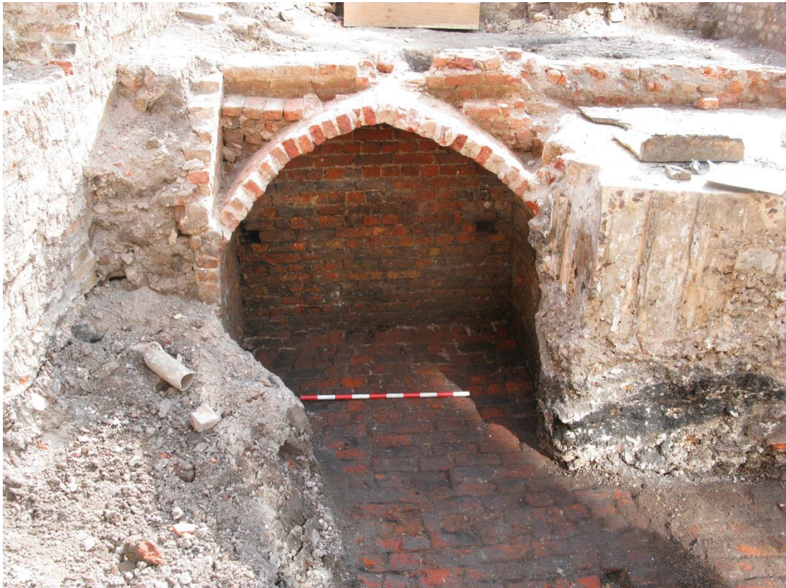
Photo 3 View of internal arch-roofed alcove [88], looking east
