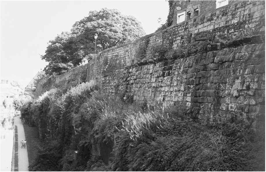
III IV.13 Massive masonry and elaborate cornice of fortress curtain wall
