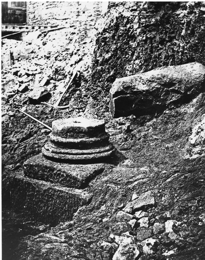
III VIII.7 Close-up of column base and fallen column drum found on Feathers Hotel site 1863.
