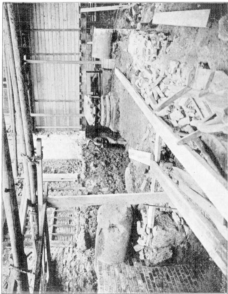
View of Excavations Looking East.
