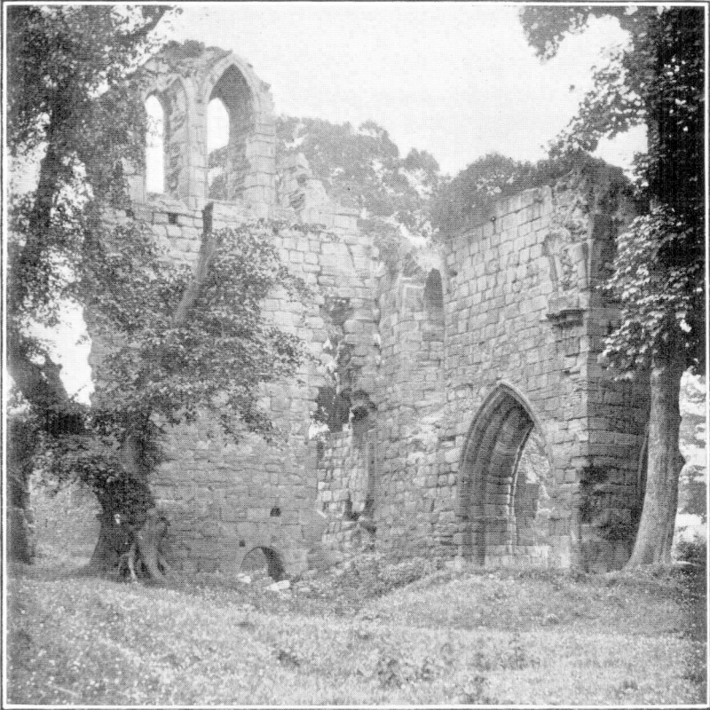
South Transept, looking south-west
