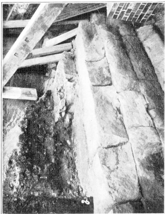
Fig. 6.—Roman Wall (portion at north end) showing at b the coursing of the rubble work
