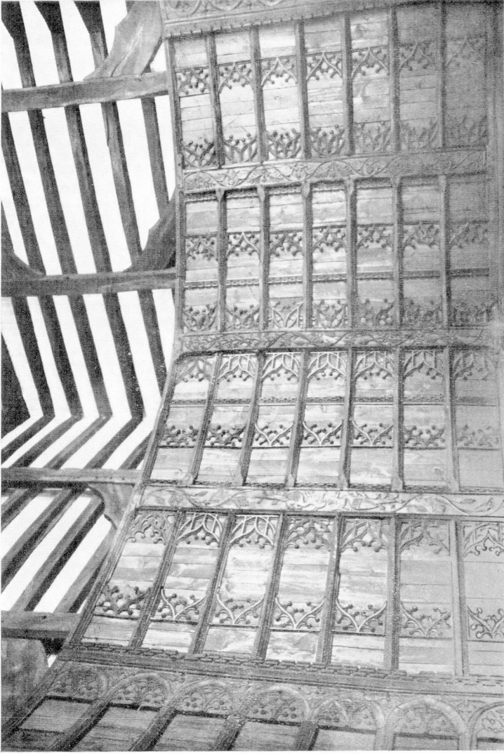
BANGOR-ON-DEE SANCTUARY ROOF.
