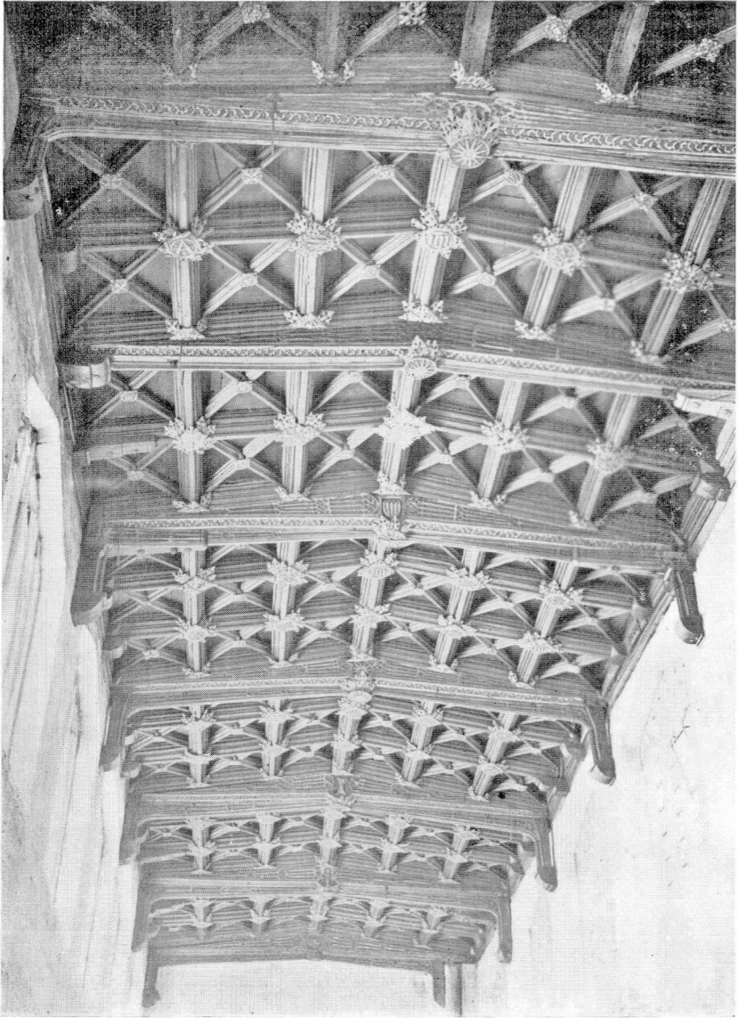
WITTON, NORTHWICH, NAVE ROOF.
