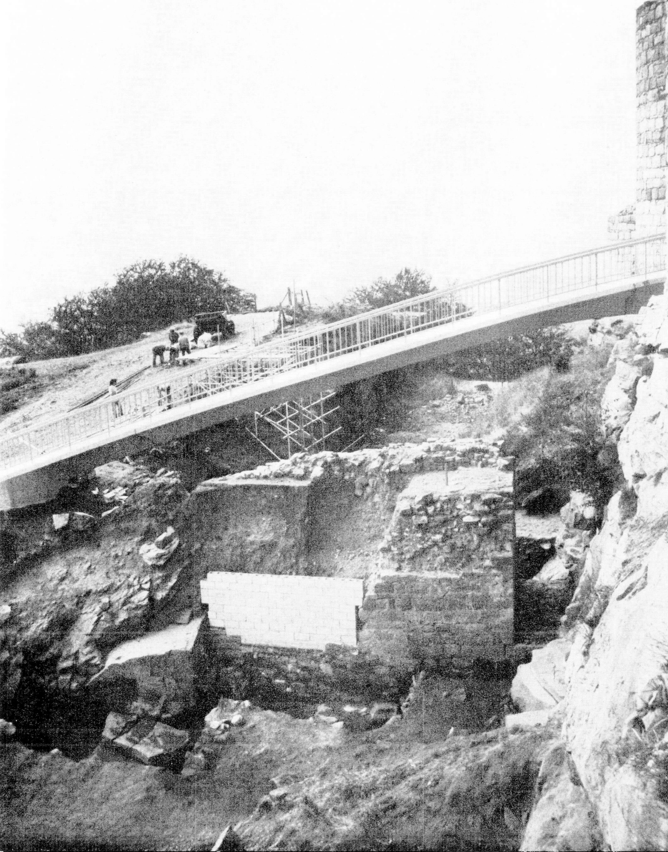
Plate II — Causeway from the east
