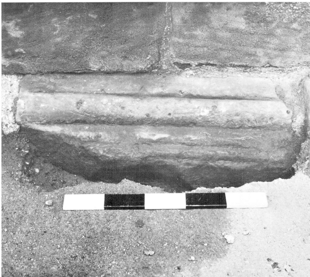
Plate 3 — Damaged cornice fragment, originally from the Roman wall and reused in the footings of the City Wall (Point B on Fig. 1). (Half metre scale).
