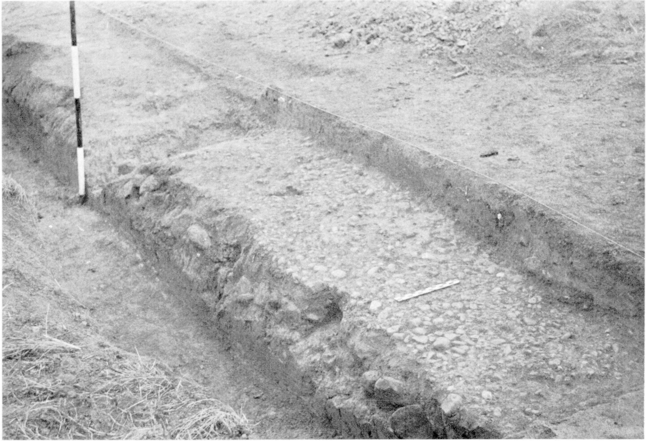
Plate 2 — The pebble surface of Road II on the sandstone blocks (imperial scale).
