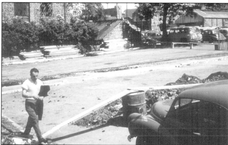
13 The opening of one of many small trenches in the Crook Street area, 1963-5. The building to the left is Matthew Henry's Chapel.
