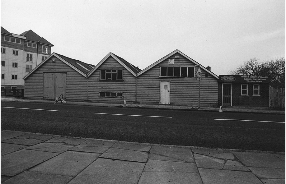
III. III.11: The New Crane Street frontage of Tilston's Boat Yard
