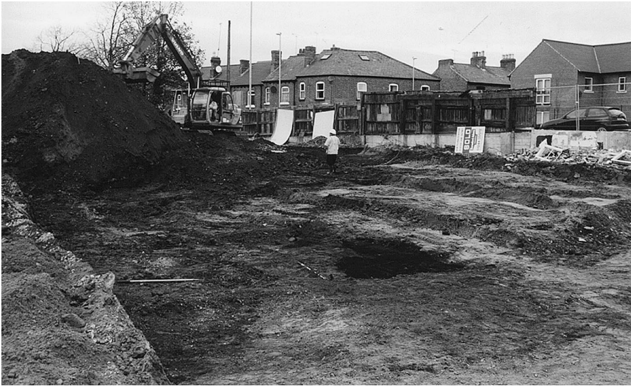
III. III.9: The build-up of debris over the wharf/slipway
