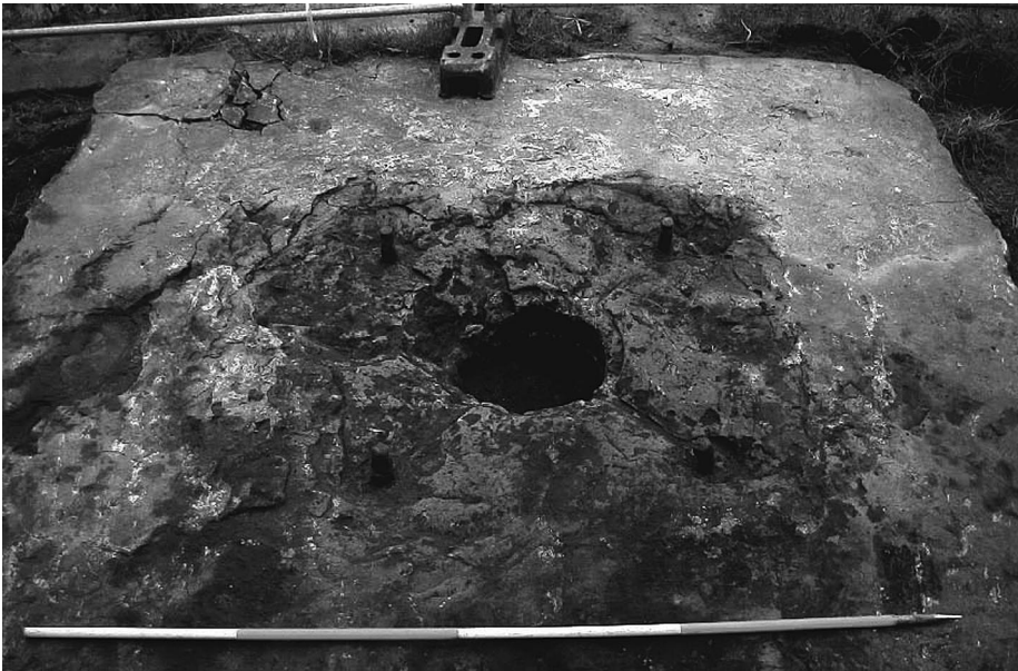
III. V.2: Detail of concrete crane base showing central pivot-hole and crane fixing bolts
