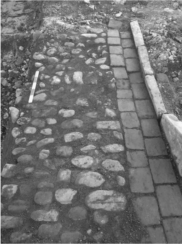
III IV.15 Phase 3 cobbled surface and kerbs of Fosbrook Street, viewed from the north
