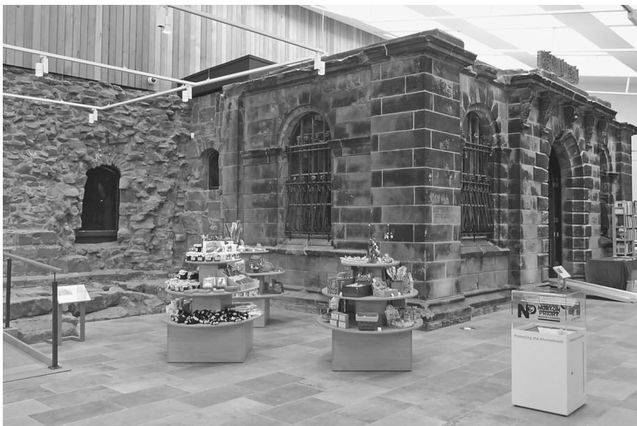
Ill VII.9 The museum atrium, showing the Victorian porch and part of the undercroft, with the foundations of the Abbot's Tower to the left
