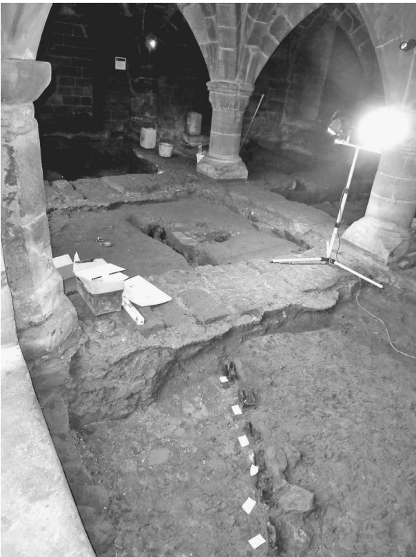
above: III VII.6 The Victorian tiled floor in the southern bay of the twelfth-century undercroft prior to excavation. ©The Norton Priory Museum Trust
