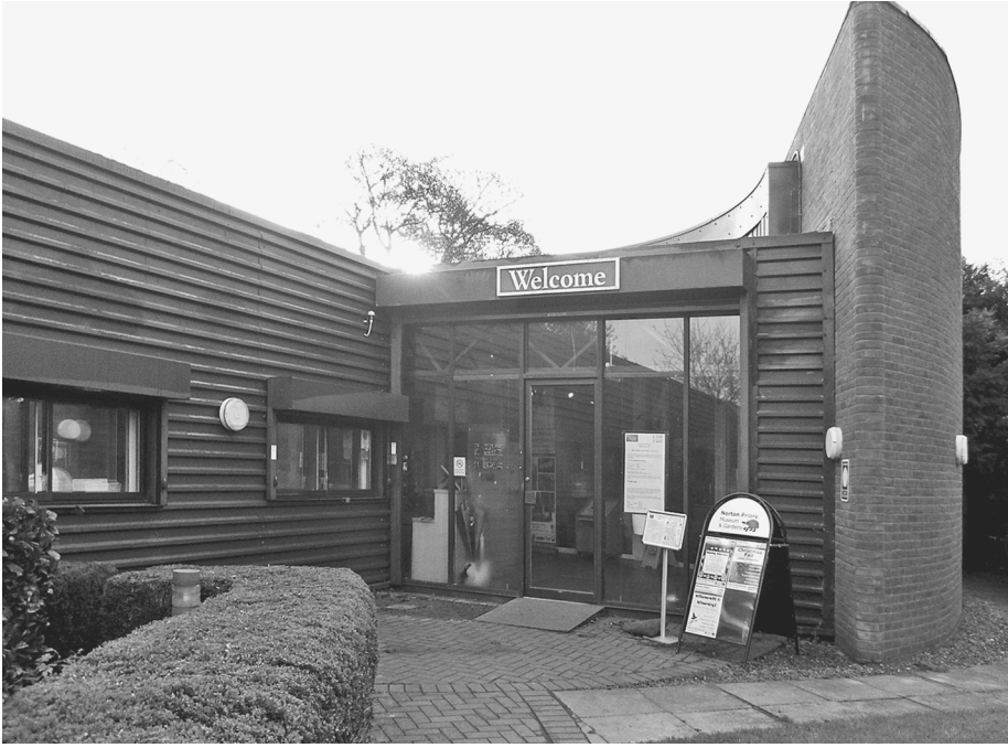
III VII.1 The entrance to Norton Priory Museum built in 1982, seen here just prior to the start of the project in 2014. © The Norton Priory Museum Trust
