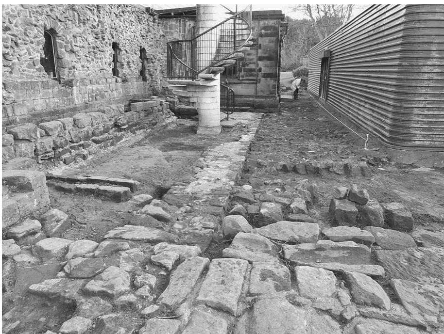
III VII.4 The excavation in the area that was to become the new atrium, between the west wall of the undercroft and the old museum, showing the line of the terraces on either side of the porch that can be seen in photographs of the Victorian house. ©The Norton Priory Museum Trust
