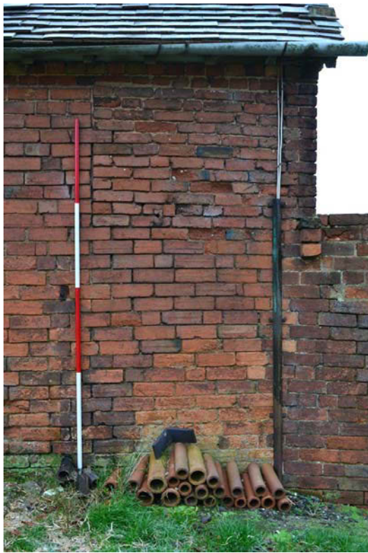
Plate 5: Brickwork joints from the north
