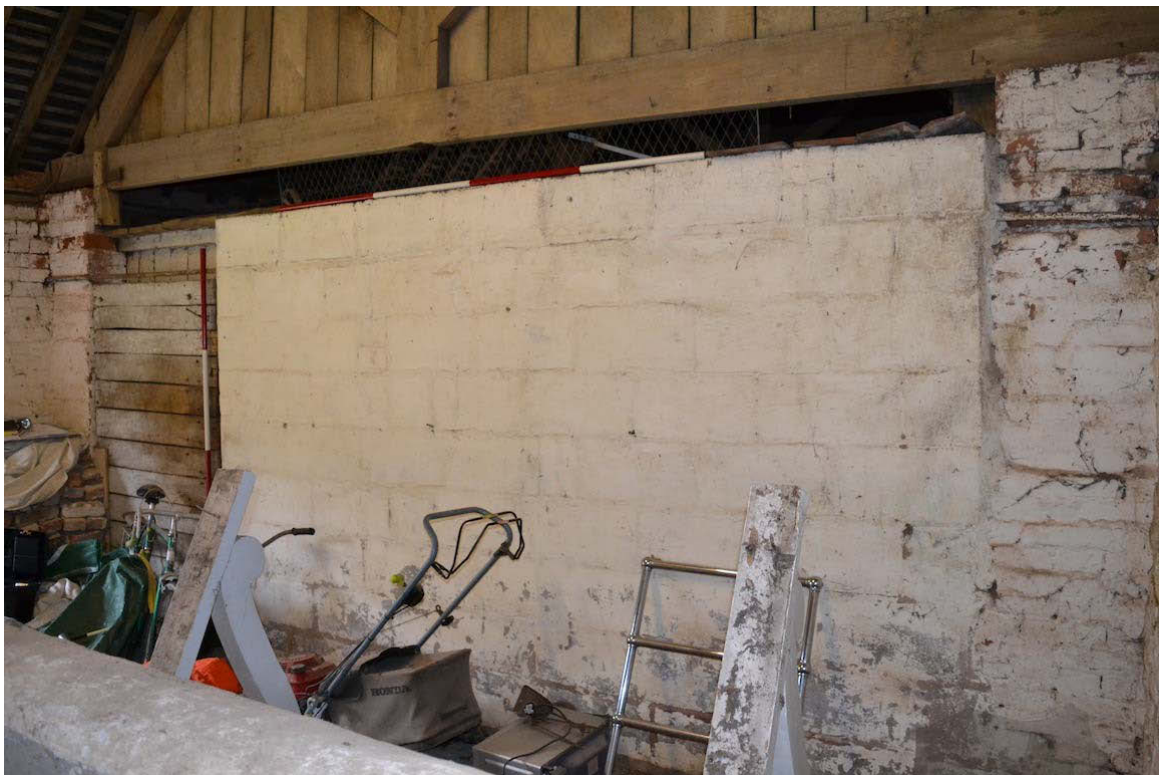
Plate 17: G2, eastern partition from the south east
