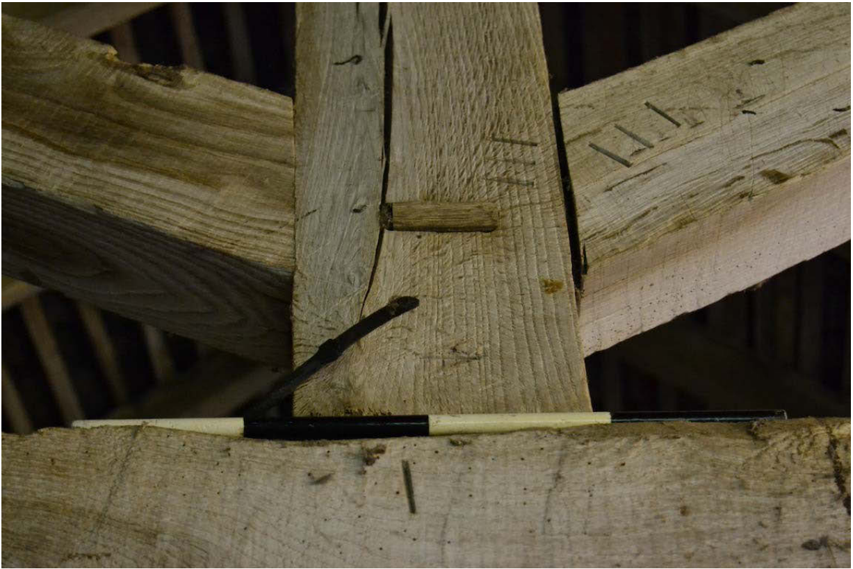
Plate 26: G4, central roof truss, junction of tie beam and king post
