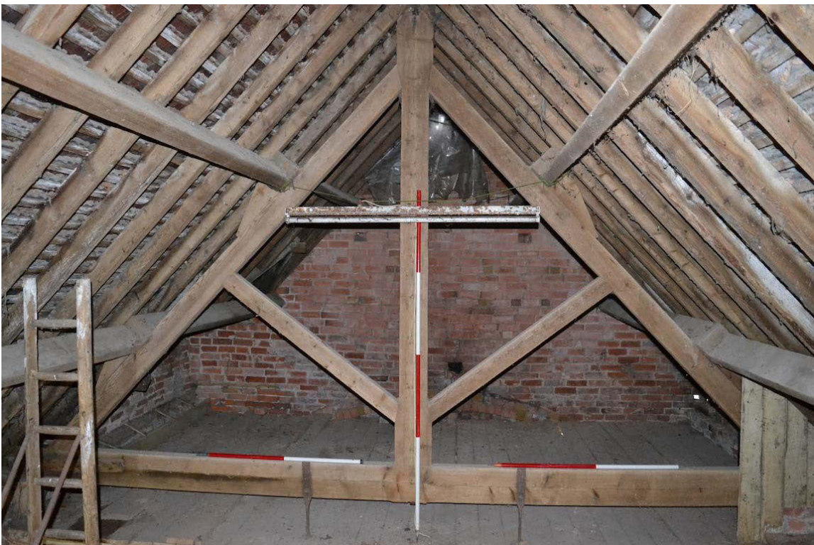
Plate 29: F1, roof truss from the west
