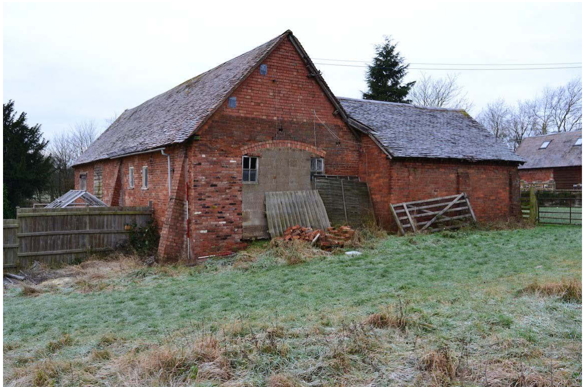
Plate 8: The building from the south east
