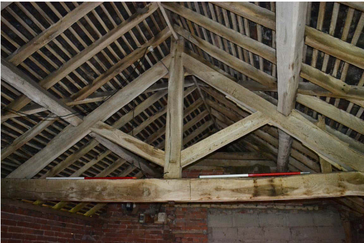
Plate 23: G4, central roof truss from the north
