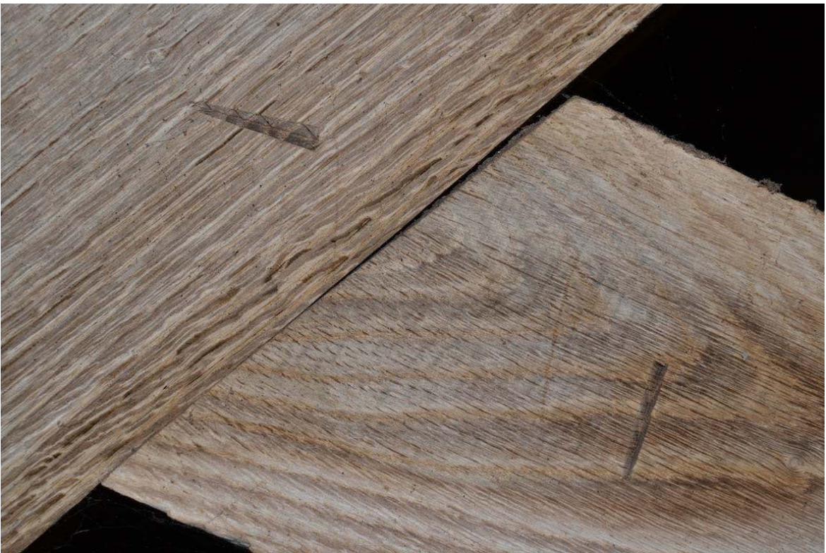
Plate 25: G4, central roof truss, junction of eastern principal and raking strut
