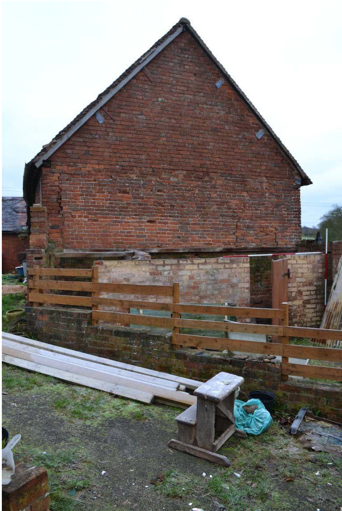
Plate 9: The building from the west
