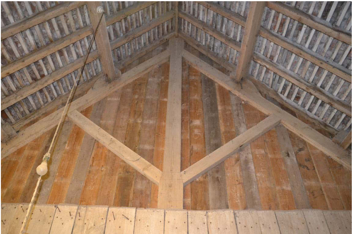
Plate 15: G1, roof truss from the west
