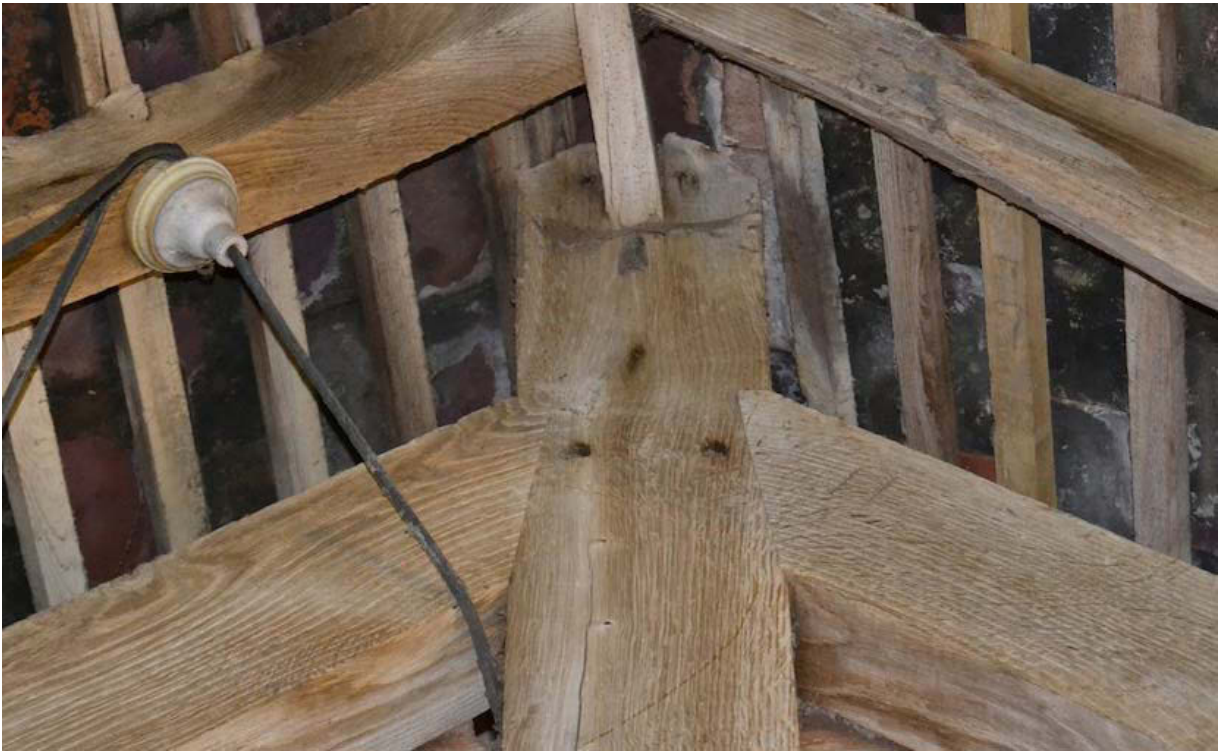
Plate 27: G4, central roof truss, head of the king post
