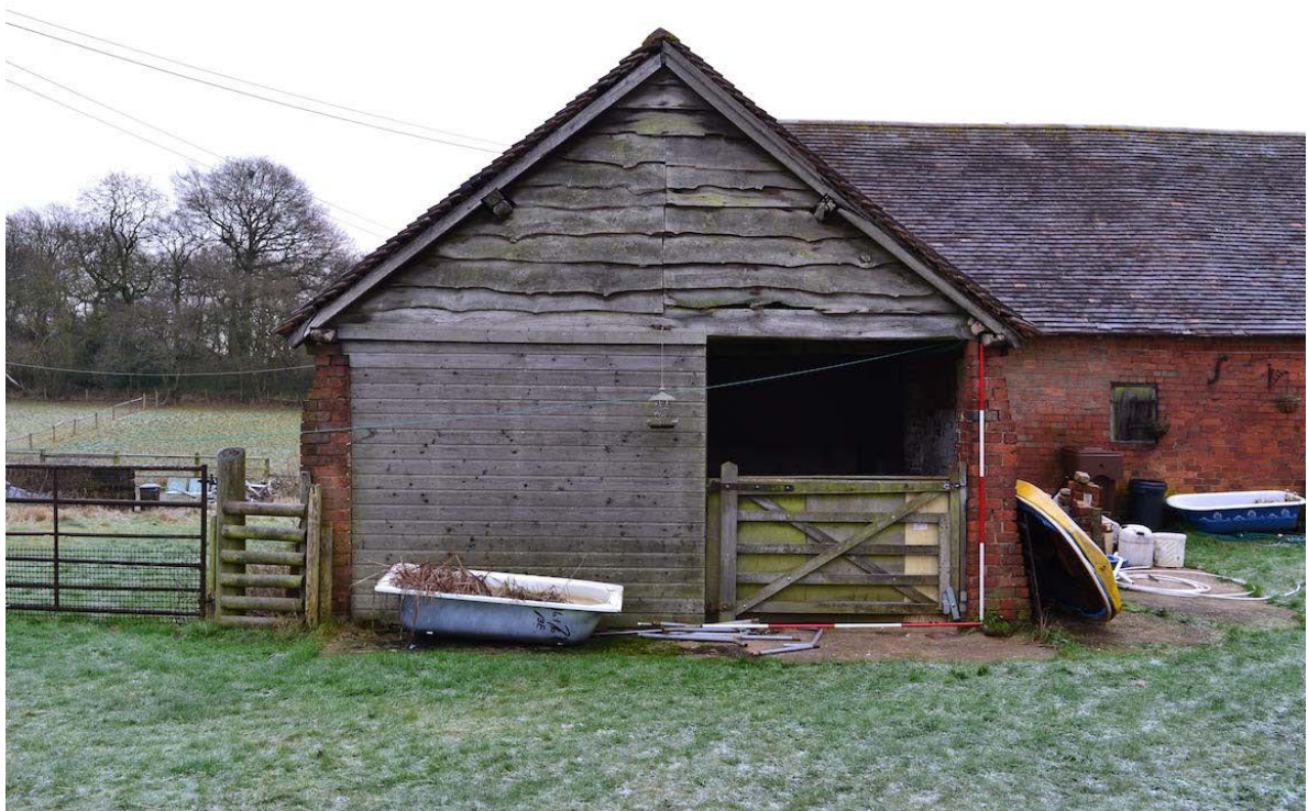
Plate 6: Cart shed from the north
