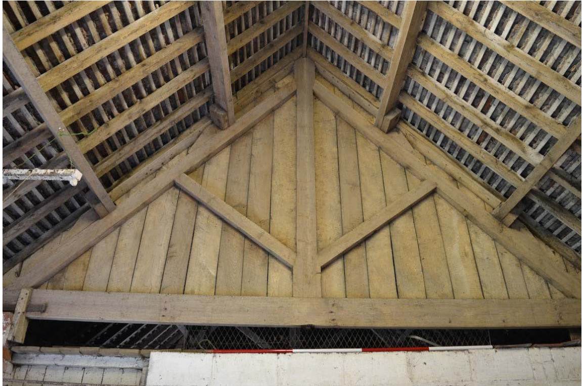
Plate 18: G2, roof truss from the west
