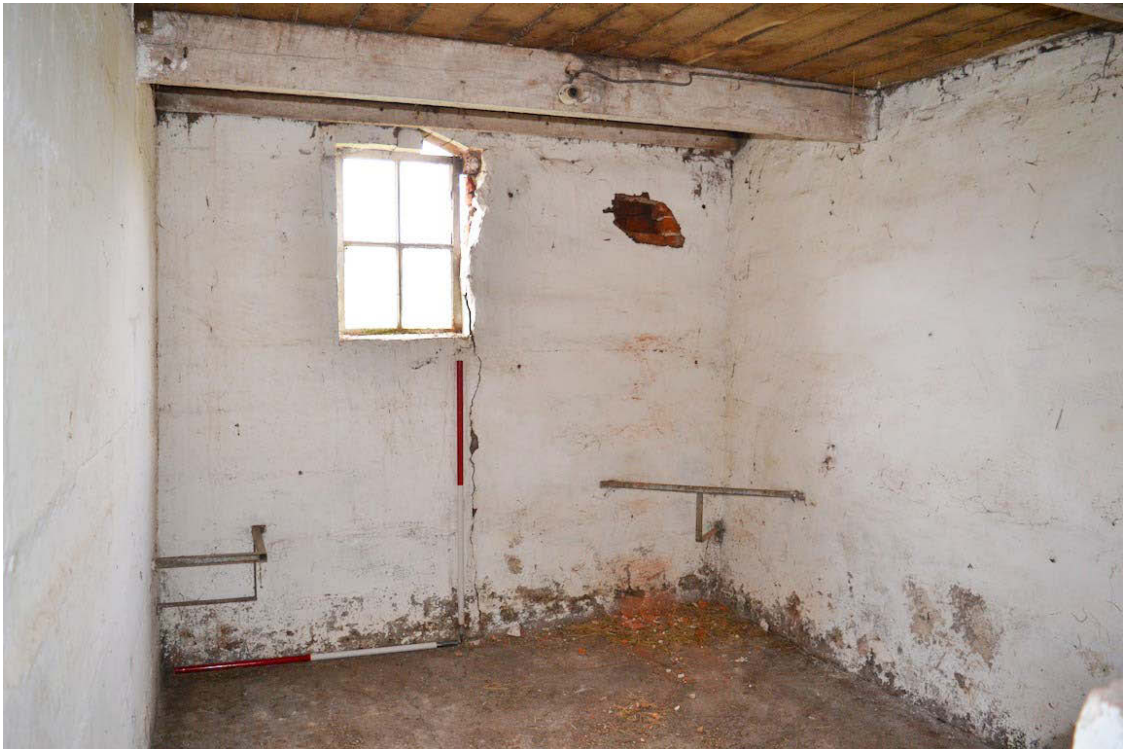
Plate 20: G3, south side of blocked cart entrance from the north west
