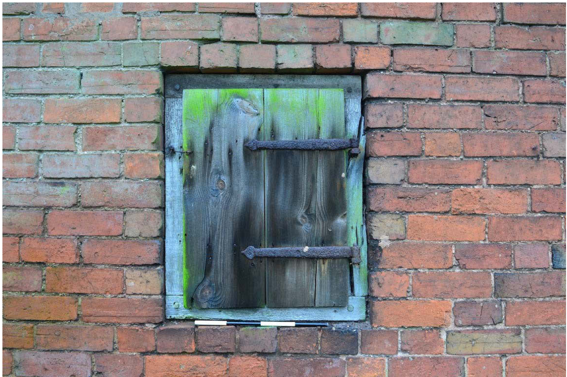
Plate 4: Eastern window from the north
