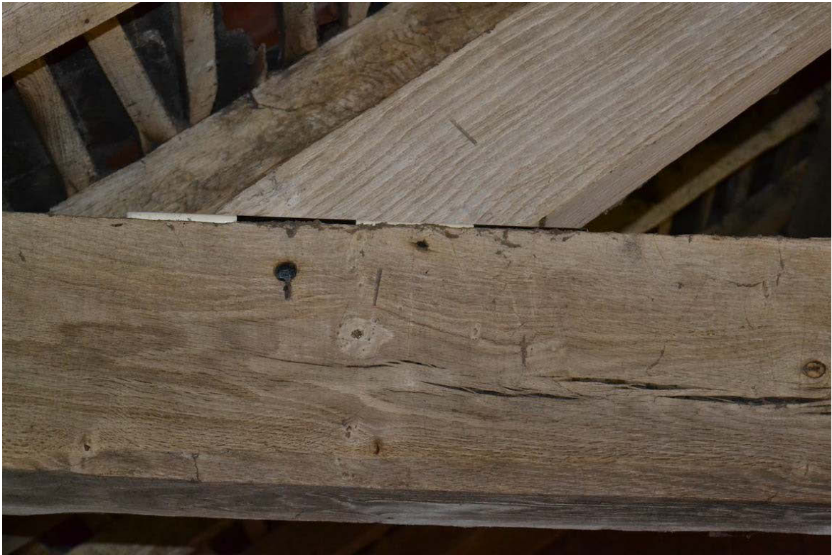
Plate 24: G4, central roof truss, junction of tie beam and eastern principal
