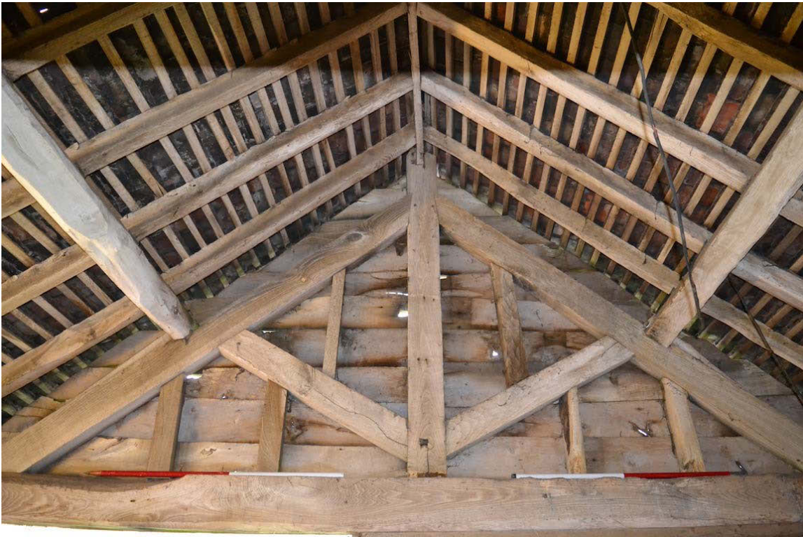
Plate 28: G4, north roof truss from the south
