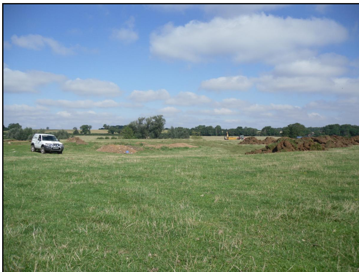
Figure 3. Photograph looking north-west showing the area of Quarry 2 being part filled by topsoil from the road areas.
