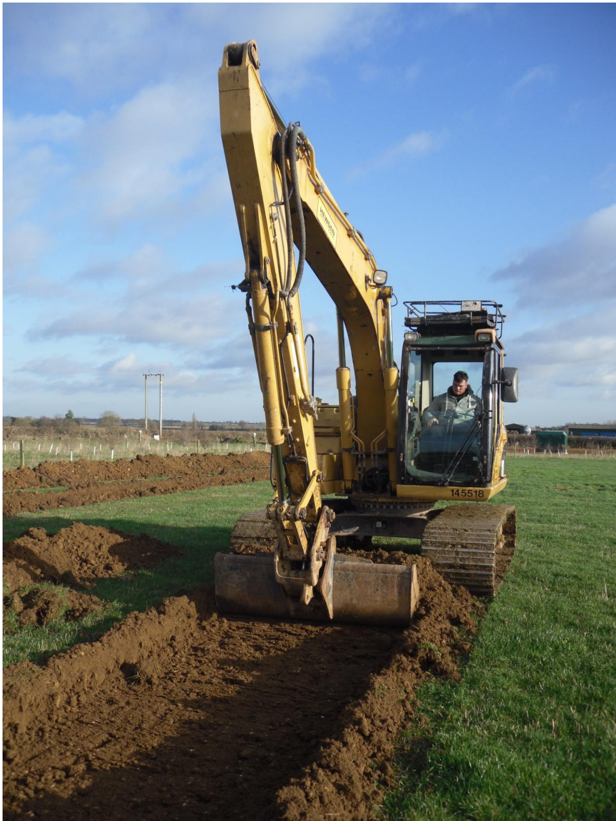
Figure 6. 360° excavator cutting trench 2. Looking northeast.
