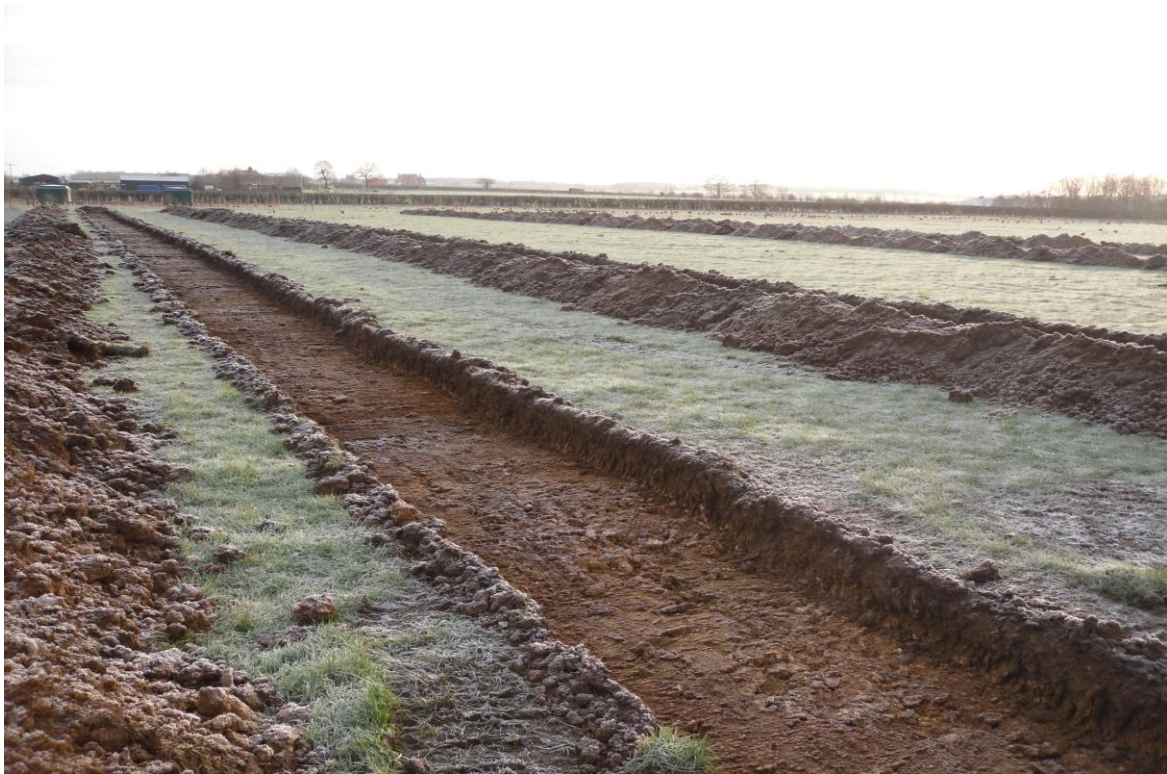
Figure 7. General view of trenches looking southeast from trench 1.
