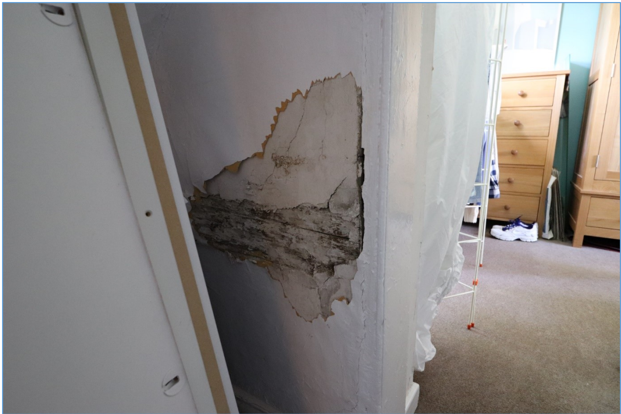
Plate 34. Detail of the exposed beam in the northern wall of Bedroom 2.
