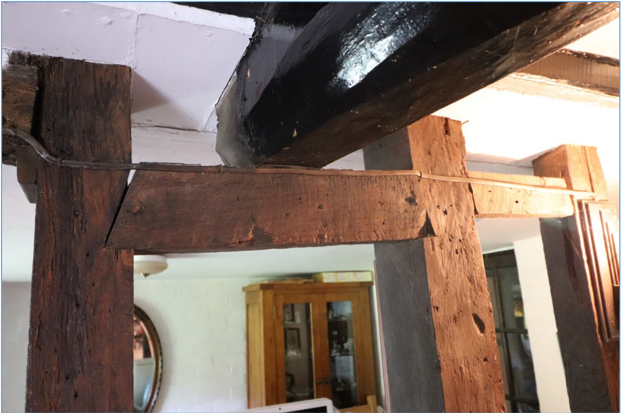
Plate 17. Detail of the bridging beam and the northern wall of the dining room.
