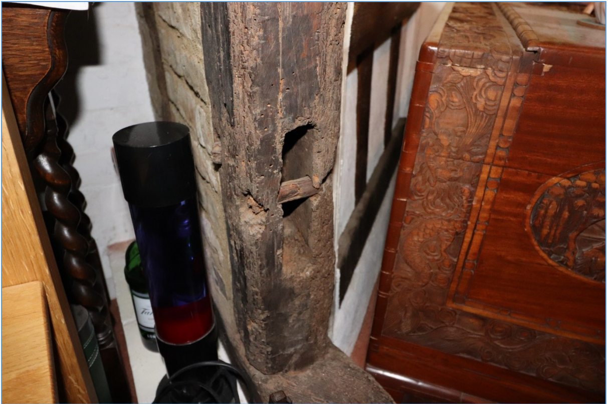
Plate 19. Detail of the empty pegged joint in the north wall of the dining room.
