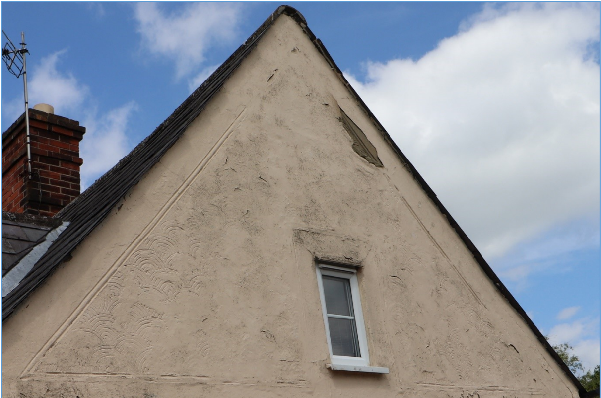
Plate 5. Detail of the southern gable, showing the decorative plasterwork beneath the paint, looking north-east.
