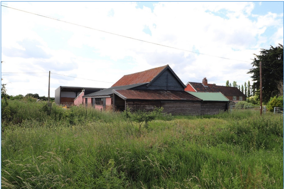
Figure 9. General view of the barn complex from the south-east, showing the eastern lean-to against the eastern gable of the main barn.
