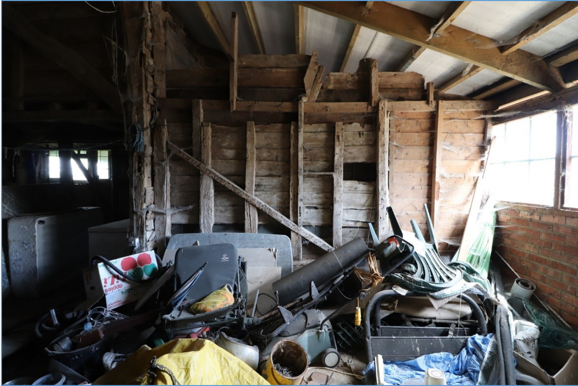
Figure 34. The eastern elevation of the central bay of the southern lean-to, looking east, showing surviving timber-framing from the original porch of the main barn.
