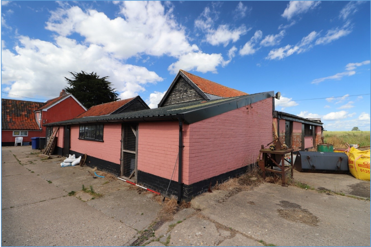
Figure 45. The south-western infill, looking north-east.
