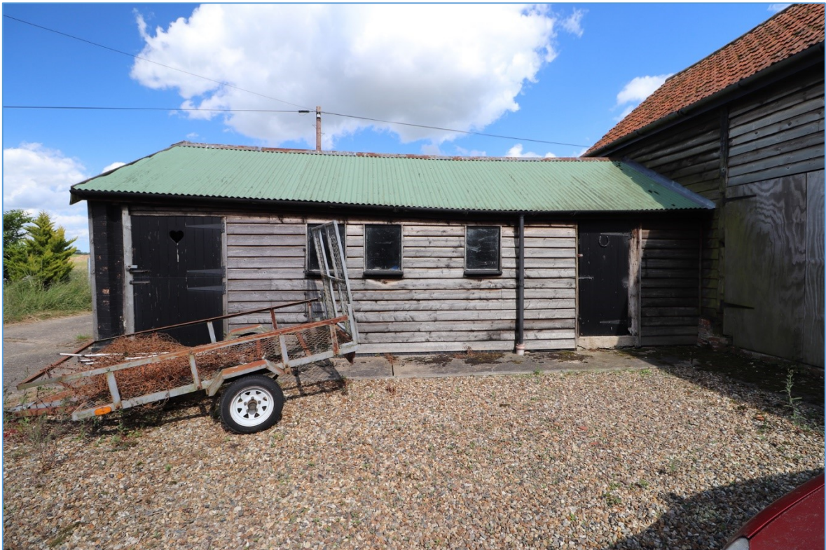
Figure 41. The western elevation of the northern extension, looking east.
