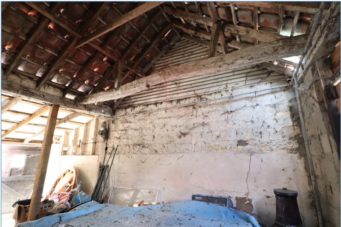
Figure 50. The northern wall of the south-western infill, looking north, showing the remnants of the smaller barn.
