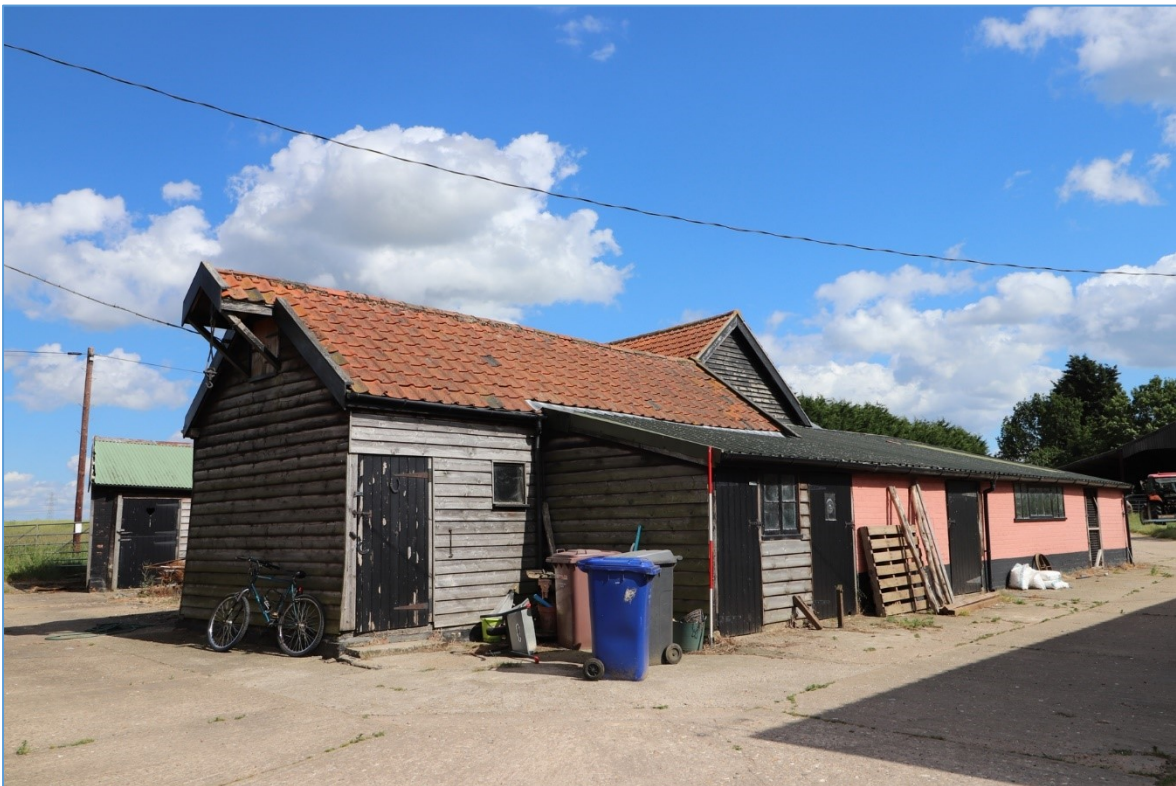
Figure 11. General view of the barn complex from the north-west, showing the tiled roof of the north-south barn and later extensions.
