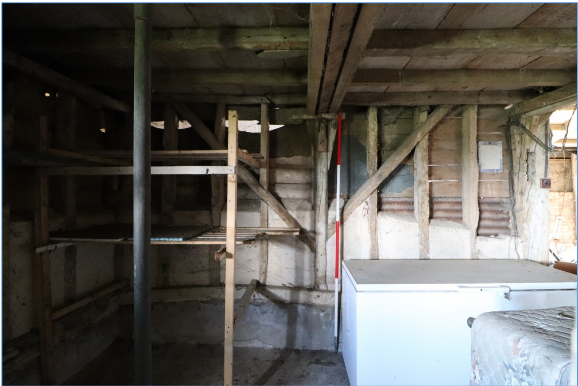
Figure 25..The southern elevation of the eastern bay, looking south, showing the surviving timber framing with render infill.
