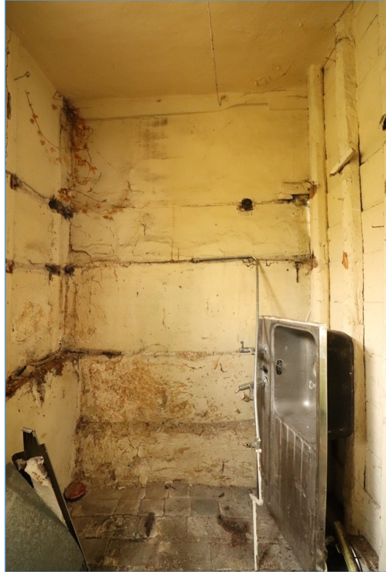
Plate 17. Interior of the northern cell of the extension, looking east.
