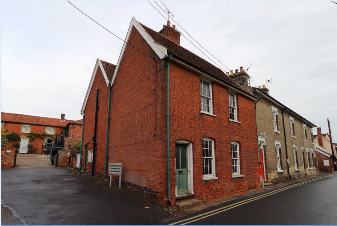
Plate 2. The property from the south-west, showing southern façade, western gable and double-pitch apex roof.
