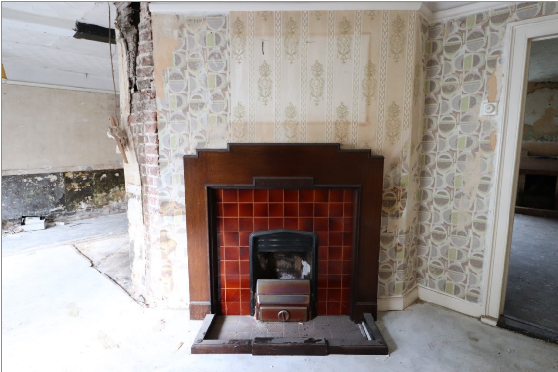
Plate 9. Detail of the open eastern fireplace, looking north-west.
