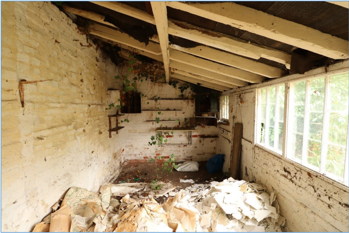
Plate 27. Interior of the outbuilding, looking east.
