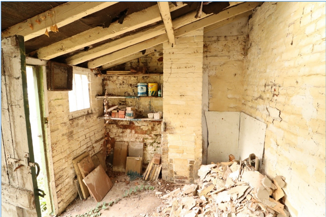
Plate 28. Interior of the outbuilding, looking west.
