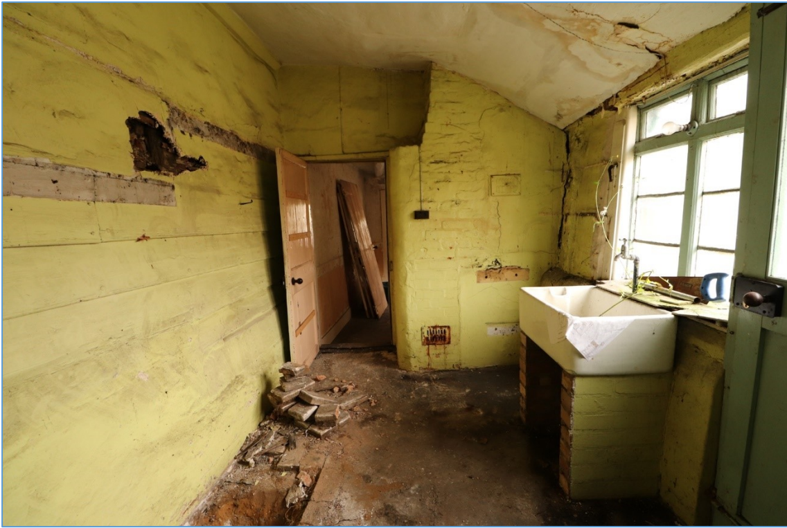
Plate 14. The interior of the north-eastern extension, looking south, showing encased chimneystack and connecting door to the main body of the property.
