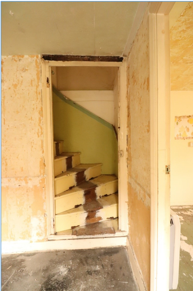
Plate 13. The entrance to the stairs, looking south.
