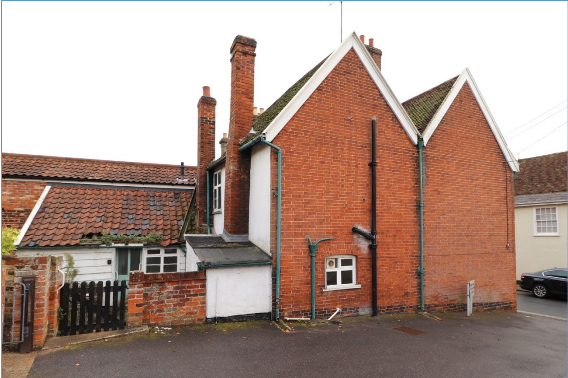
Plate 3. The property from the west, showing western gable, rear chimneystacks and extensions.
