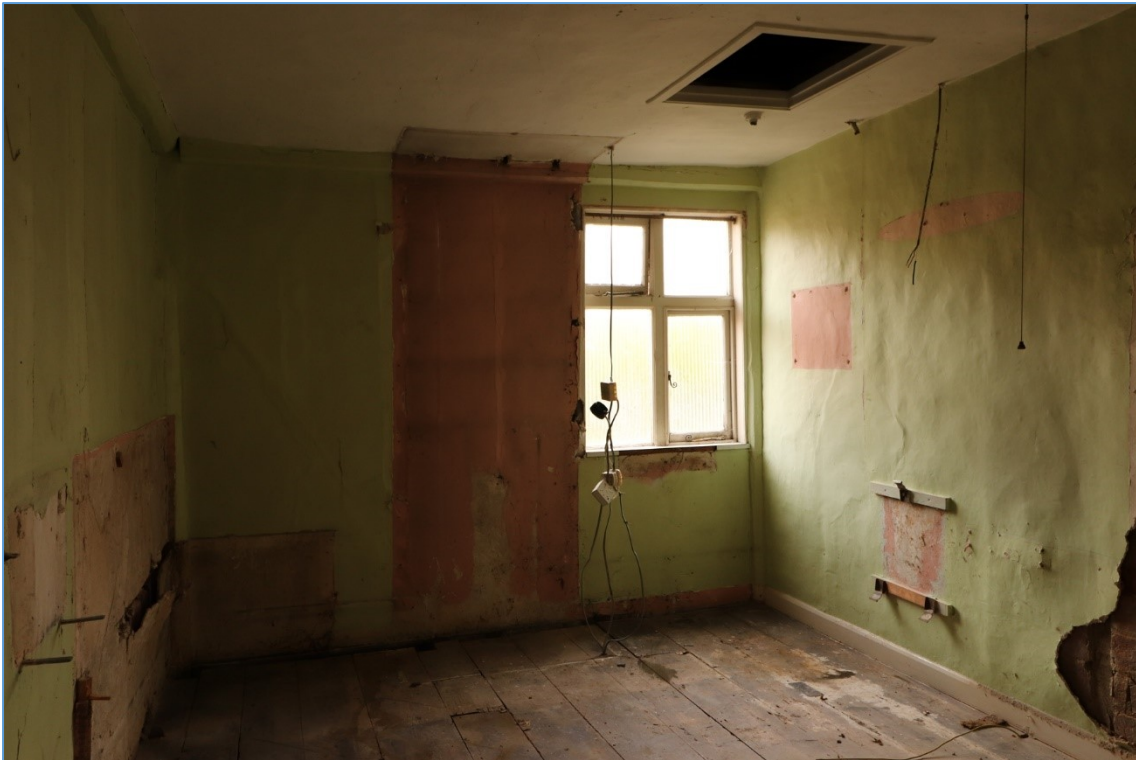
Plate 20. The north-western first-floor former bathroom, looking north.
