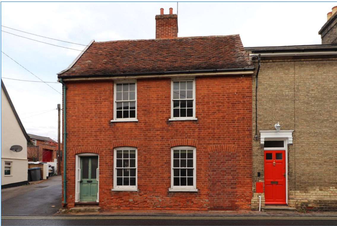
Plate 1. The southern façade of the property, showing extant windows and door, and blocked former door.
