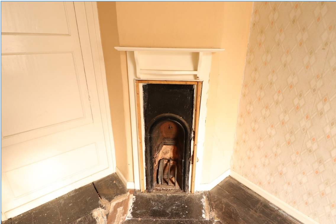
Plate 23. Detail of extant plain fireplace in the south-western first-floor bedroom, looking north-east.
