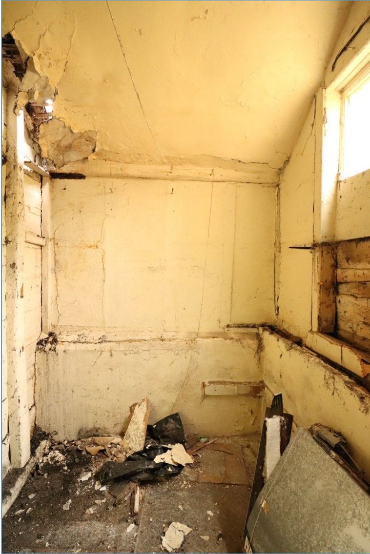
Plate 16. Interior of the northern cell of the extension, looking west.
