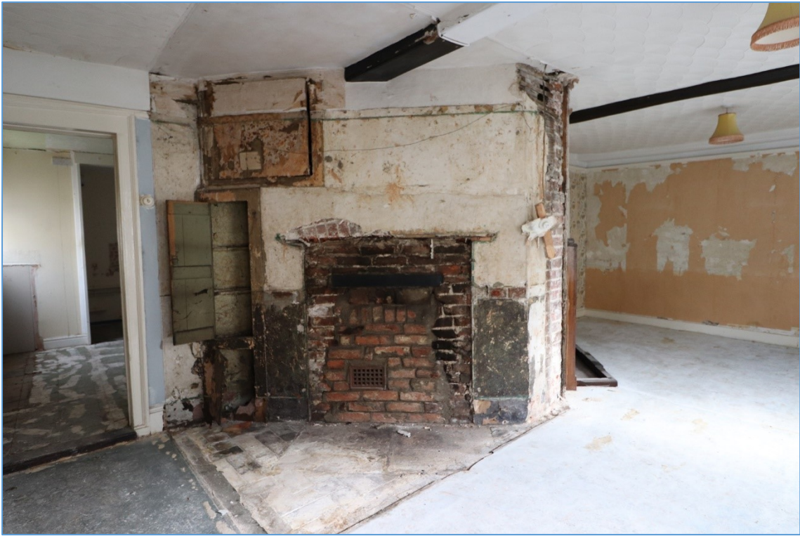
Plate 8. Detail of the blocked western fireplace, looking north-east.
