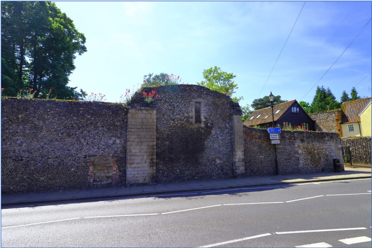
Figure 86: The postern gate on Mustow Street viewed from the north.
