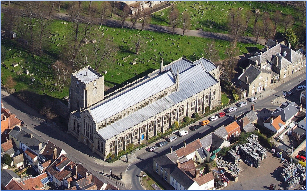
Figure 84: Aerial photograph of St Mary's church from the south-west, showing its relationship with the south-western boundary of the precinct. (© Mike Page, reproduced with permission)
