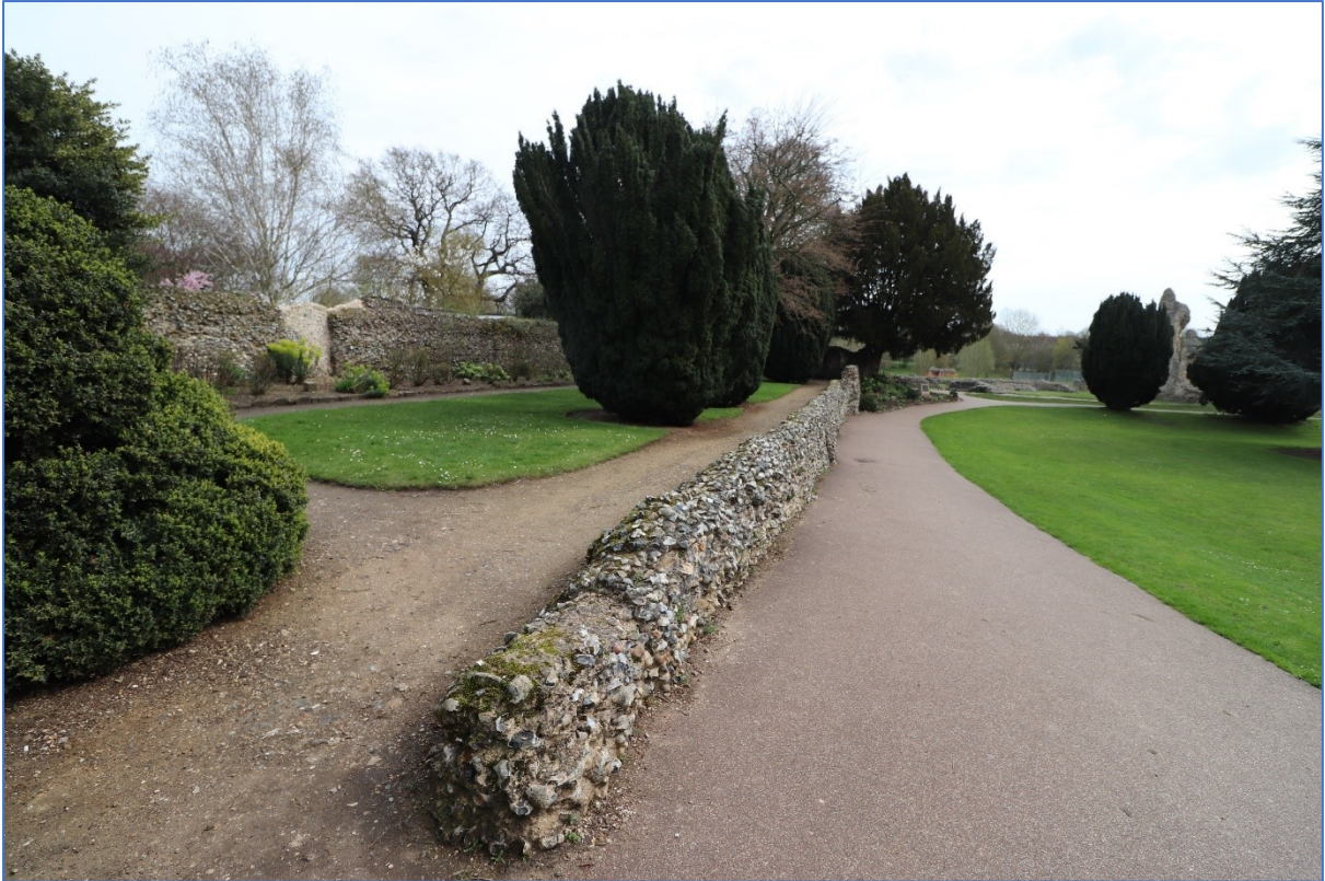
Figure 117: Looking eastwards across the ruins of the refectory, still largely full of rubble. Contrast the ground levels inside the building (left) and outside in the cloister (right).
