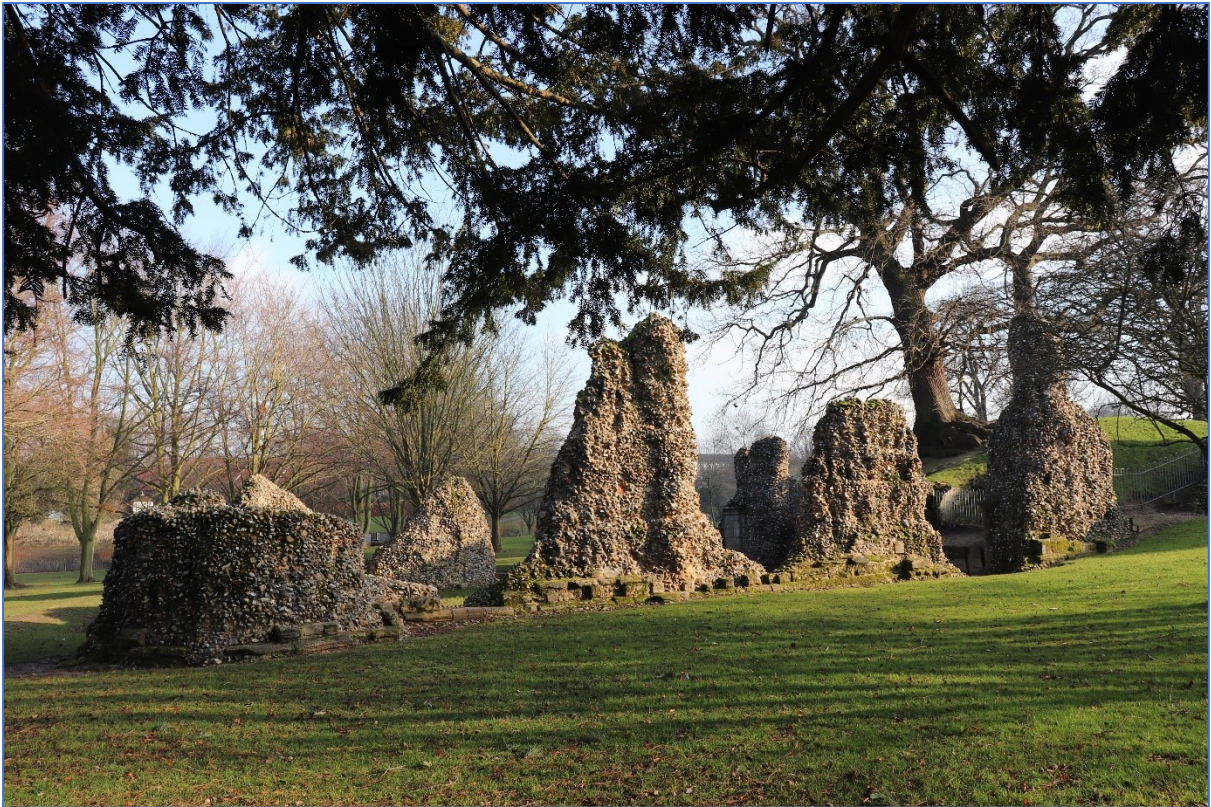
Figure 123: The exterior of the upstanding remains of the Abbot's Palace, known as the Queen's Chamber, looking south-east.
