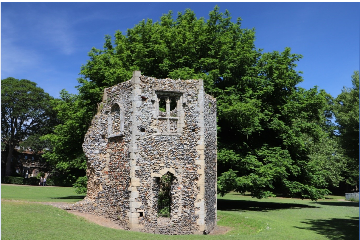
Figure 126: The ruins of the dovecote in the Abbot's Garden, looking north.
