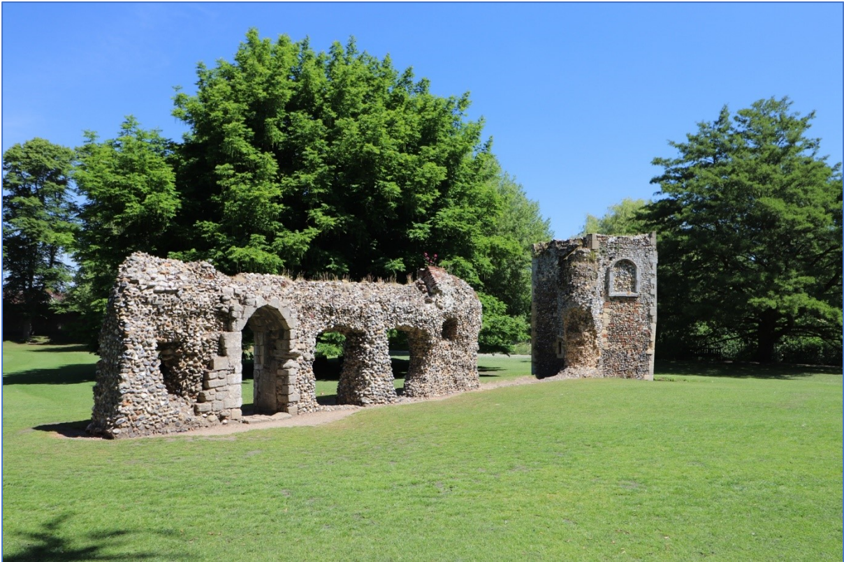
Figure 125: The view eastwards across the area of the Abbot's Garden, with dividing wall and dovecote.
