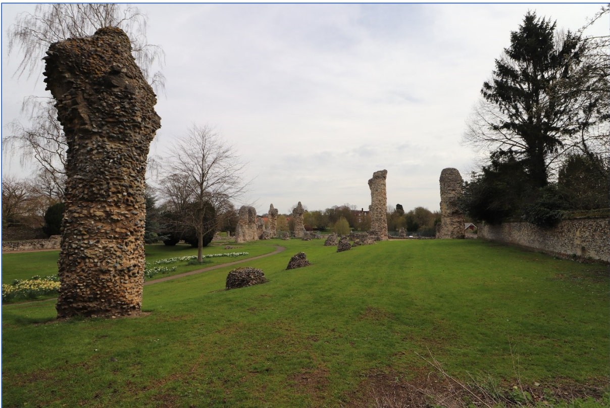
Figure 106: Looking eastwards along the abbey church, with ground level dropping to the cloister.
