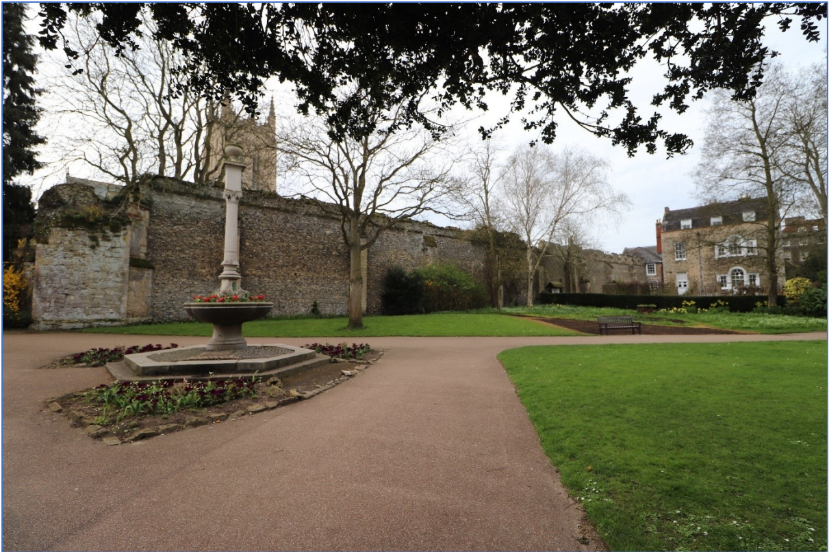
Figure 127: View of the dividing wall at the southern side of the Great Court, looking south-west.
