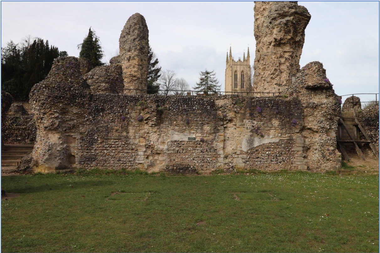
Figure 96: The western wall of the crypt, looking west, showing the wall scars of the former arcading and the locations of the northern and southern staircases into the crypt.
