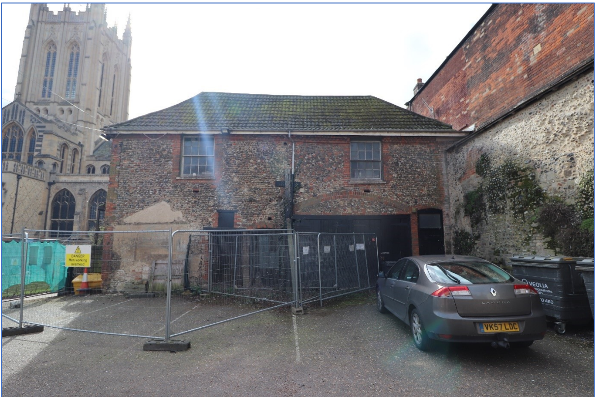
Figure 146: The stable-block and cart-lodge associated with Abbey House, looking south. The wall to the west (right) preserves the medieval precinct wall.
