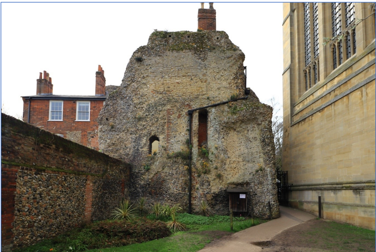
Figure 110: The site of the former northern octagon, looking south, showing the wall scars, openings and stair turret where it would have joined the west front.
