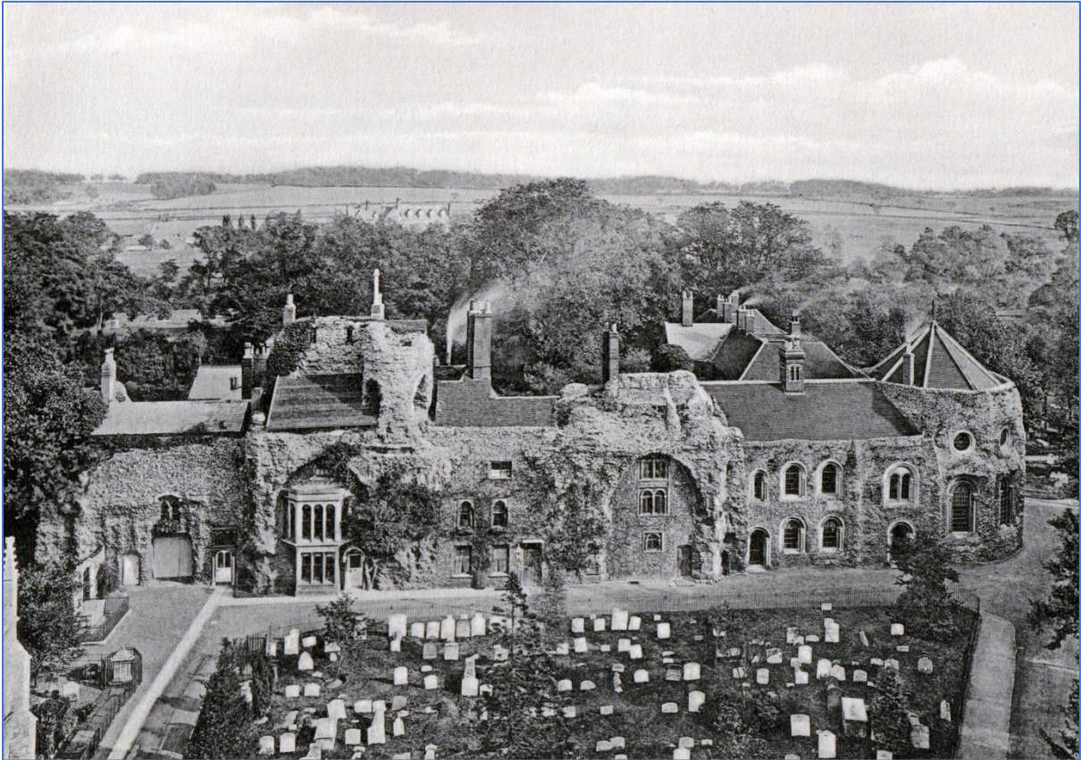
Figure 150. An early 20 th century view of the west front from the top of the Norman Tower clearly showing the density of the burials in the Great Churchyard.
