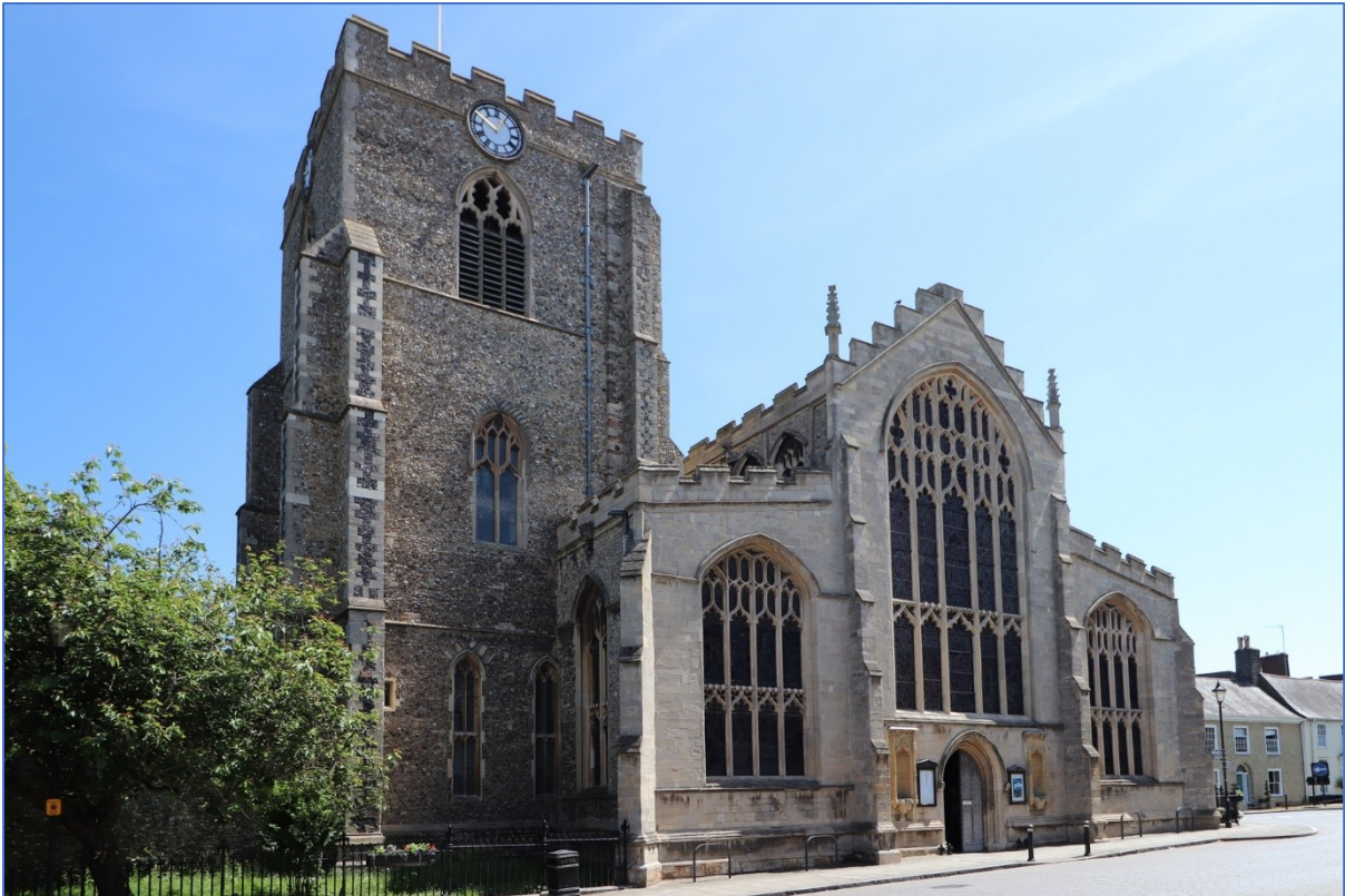
Figure 134: St Mary's church, looking westwards, showing the offset northern tower and the traces of the precinct wall extending to the north of the tower.
