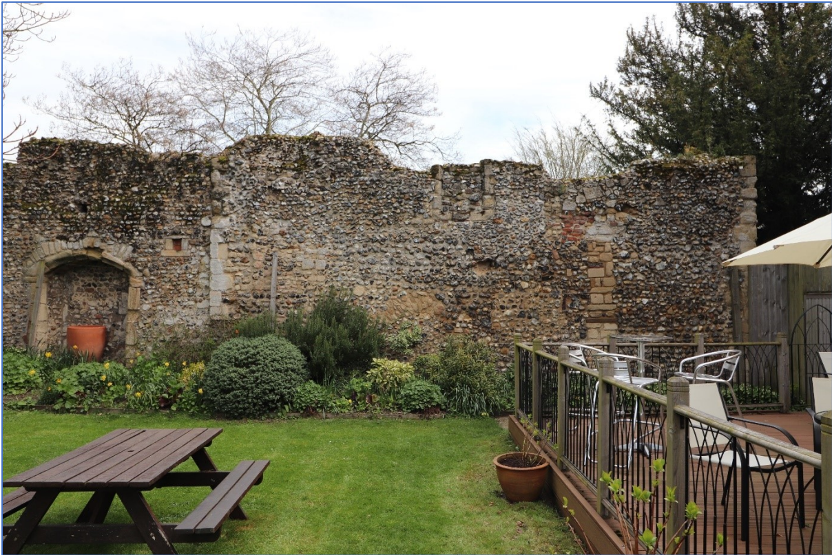
Figure 129: The eastern wall of the Cathedral Garth, looking east, showing the preserved gable end of a medieval building, with a blocked doorway to the north..
