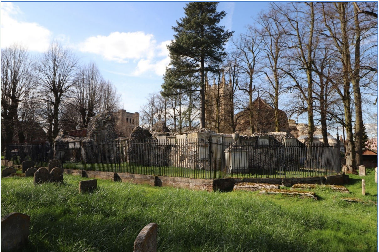
Figure 131: The cordoned-off ruins of the Chapel of the Charnel, looking north.
