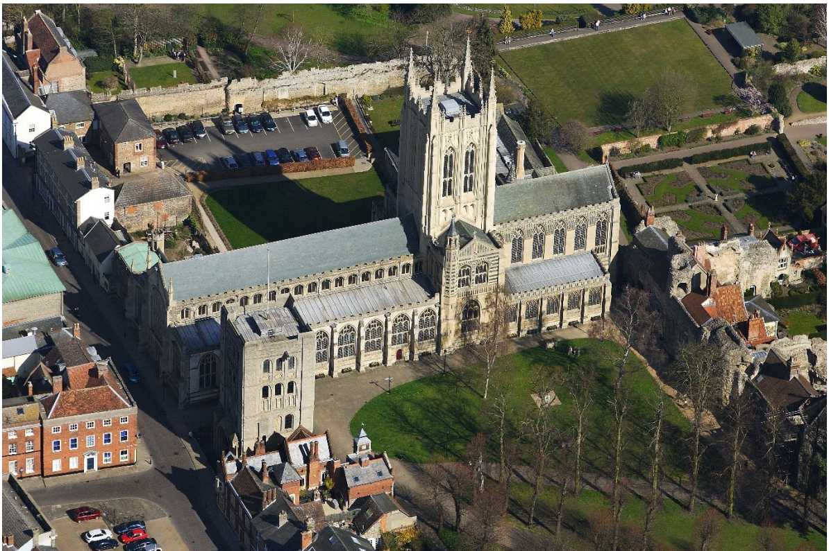
Figure 85: Aerial photograph of St Edmundsbury Cathedral (formerly St James' church) from the south, showing its relationship with the Norman Tower and the west front of the abbey church. (© Mike Page, reproduced with permission)
