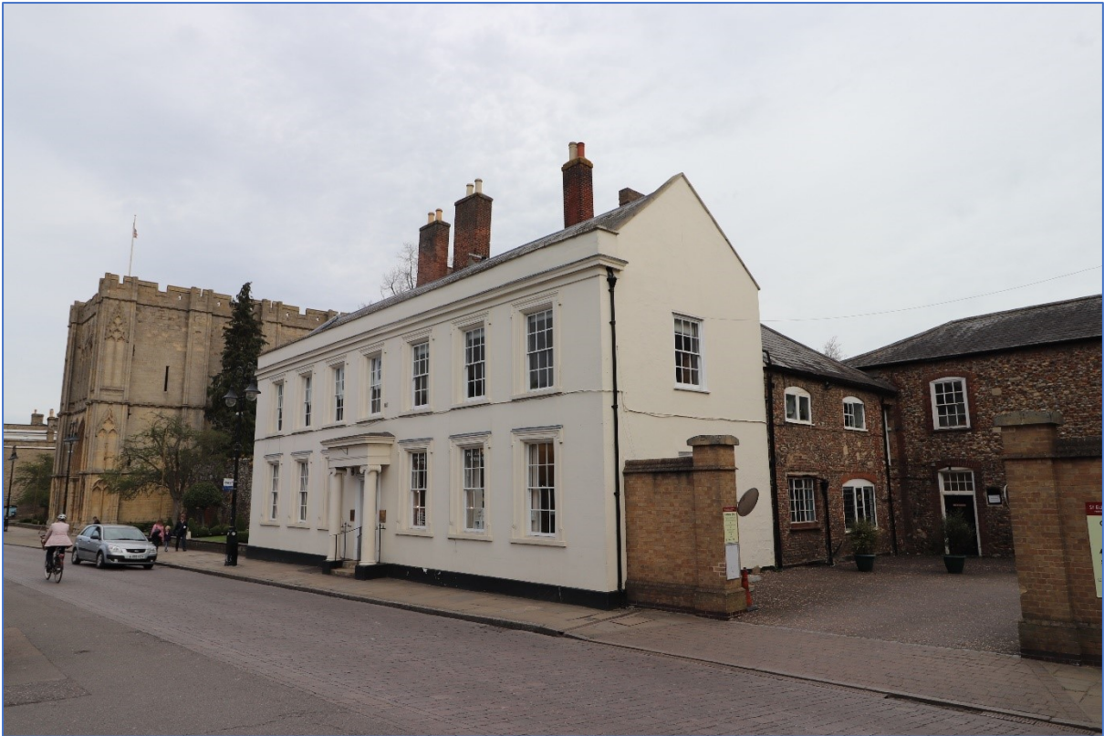
Figure 145: Abbey House looking north-east, with the Abbey Gate beyond and extensions to the rear.
