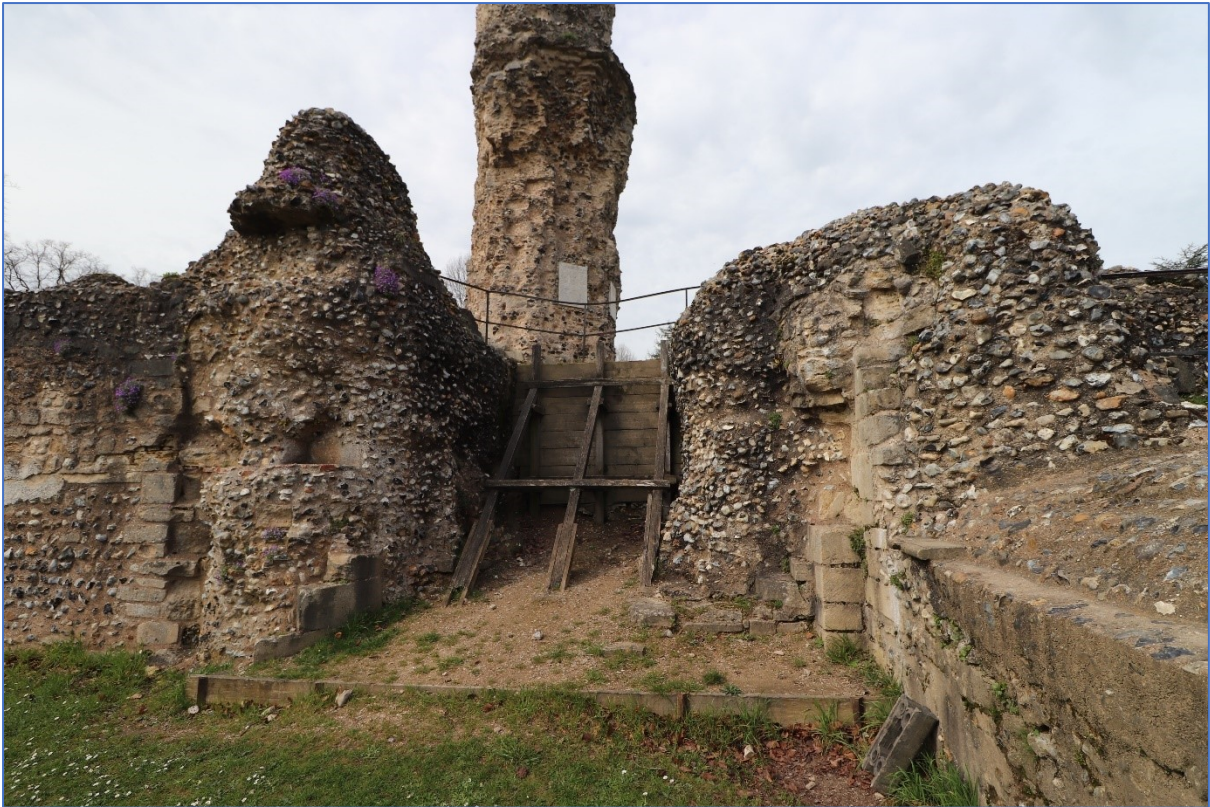
Figure 98: View of the position of the staircase leading from the north transept to the crypt, looking west, showing the wooden shuttering now used to support the backfilled passage..
