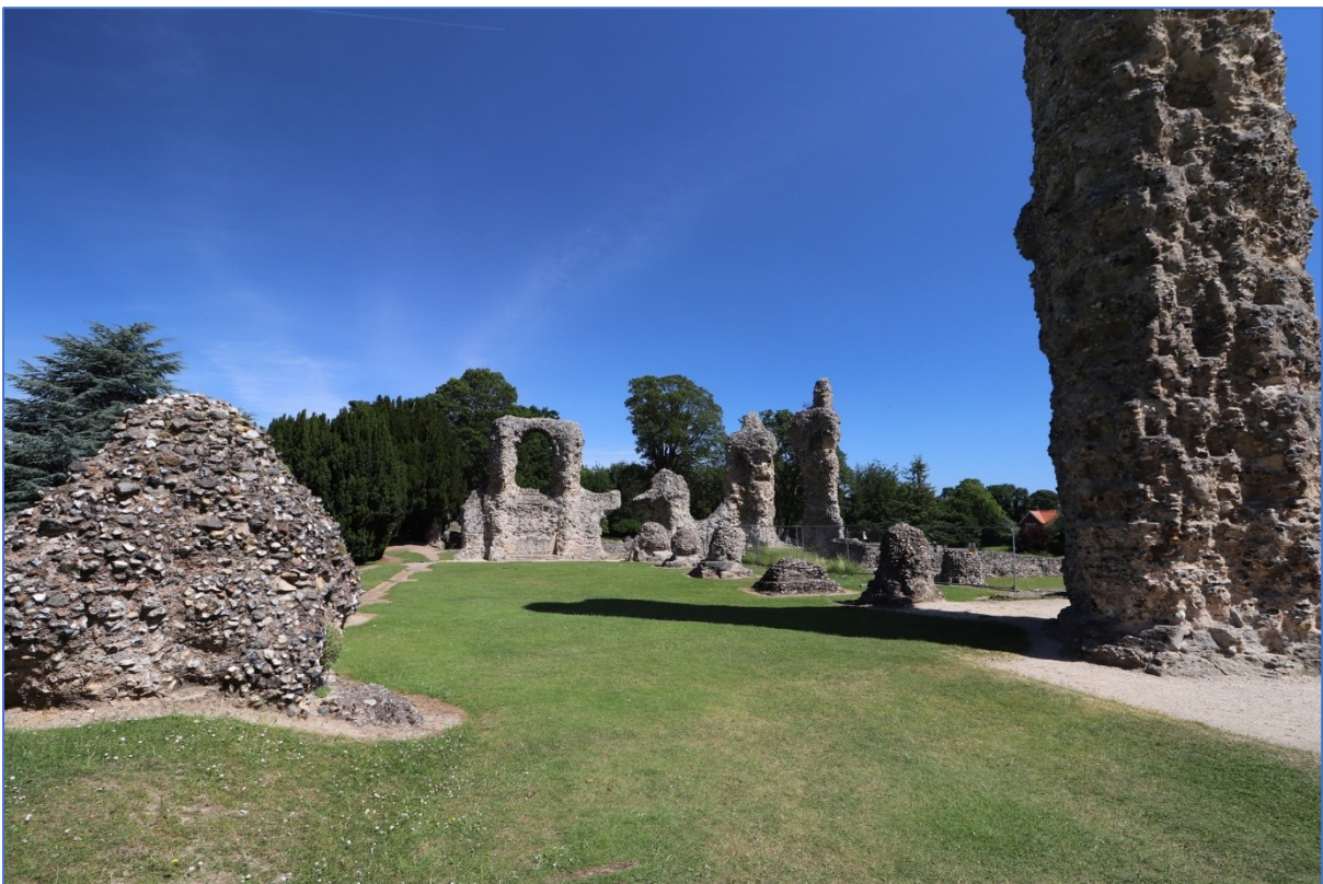
Figure 102: The north transept, looking north, showing the piers of the eastern aisle of the transept and the remnants of the cloistral buildings beyond.
