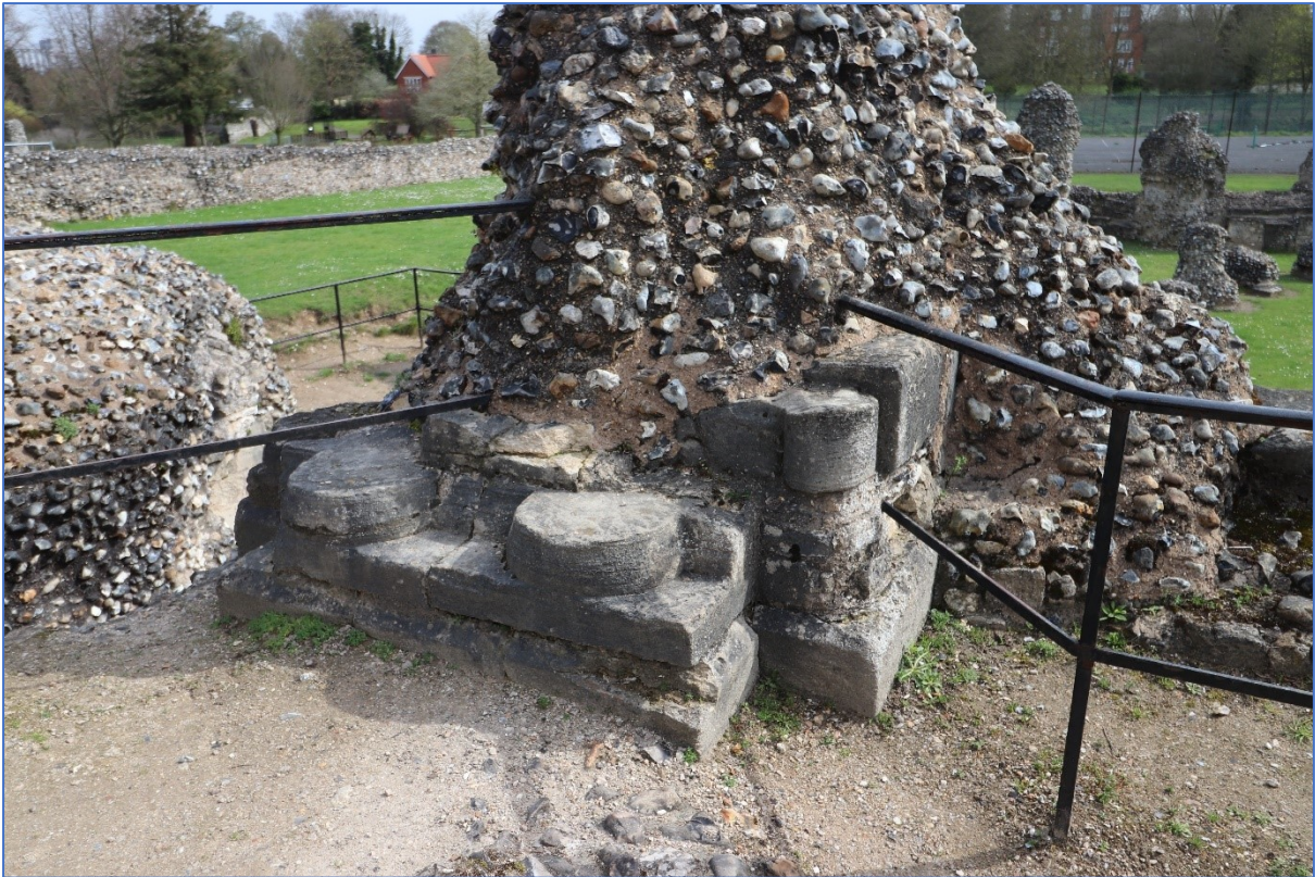
Figure 99: Close-up view of the base of the north-western presbytery pier, intended to support the original crossing of the abbey church before its enlargement.
