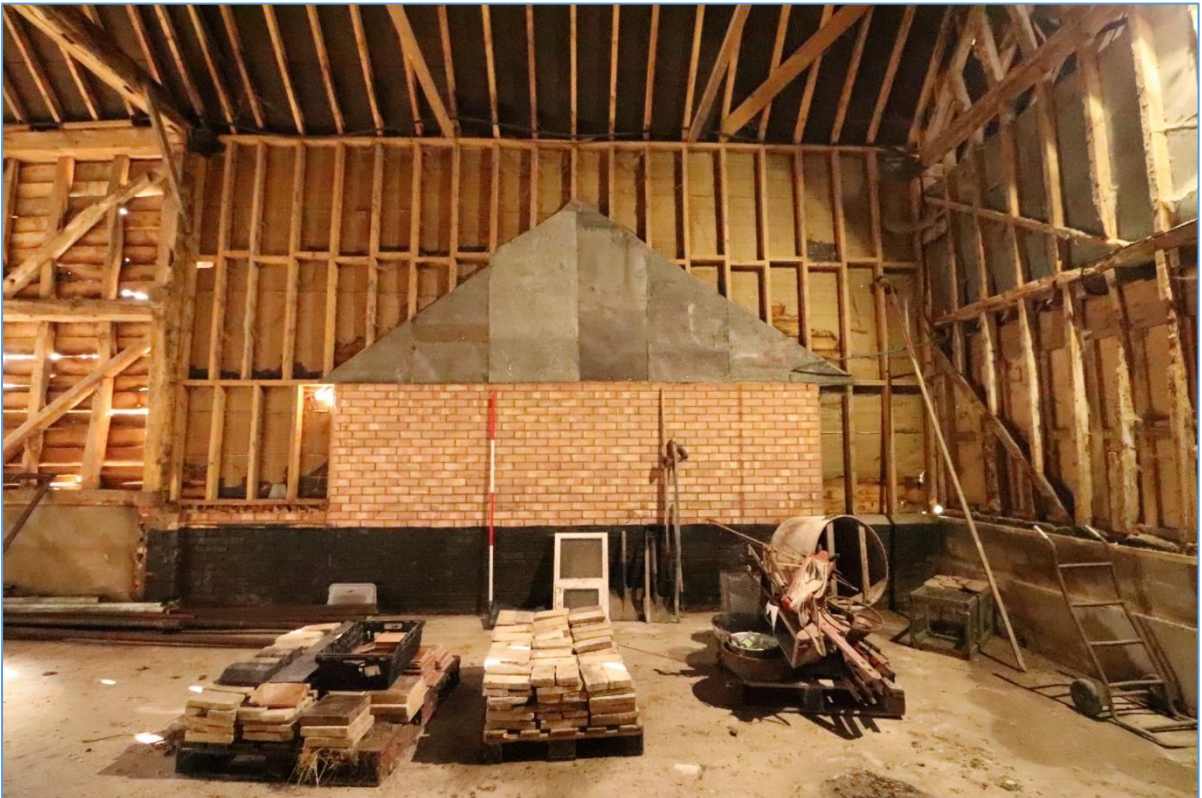
Plate 54. Interior of Building E, looking west.
