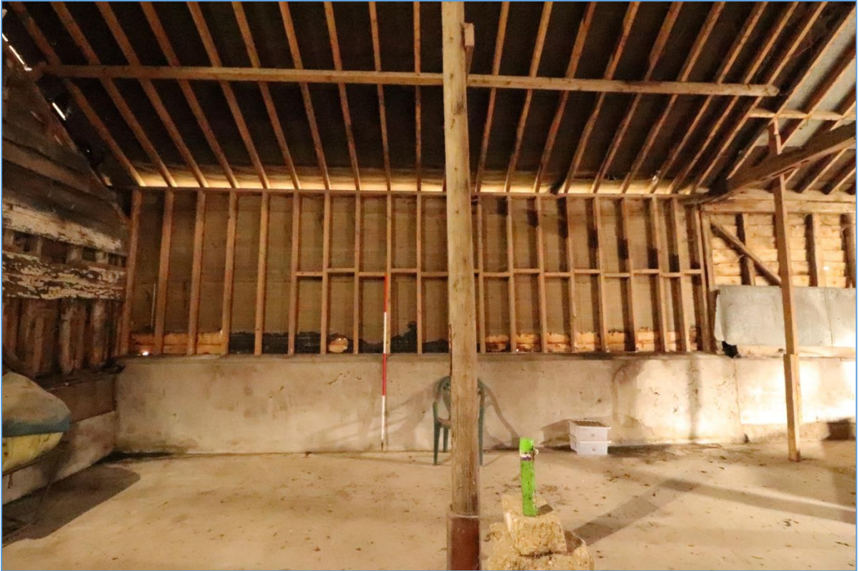
Plate 53. Interior of Building E, looking east.
