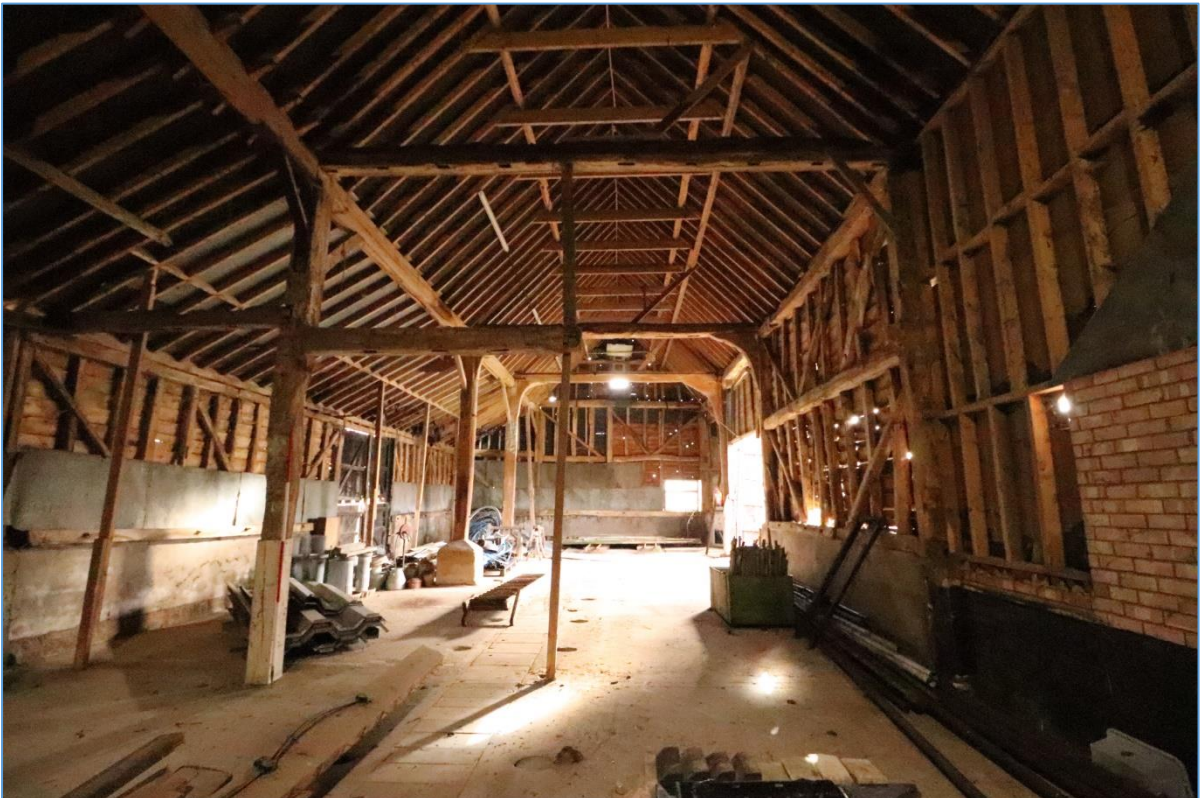
Plate 12. The interior of Building A, looking south.
