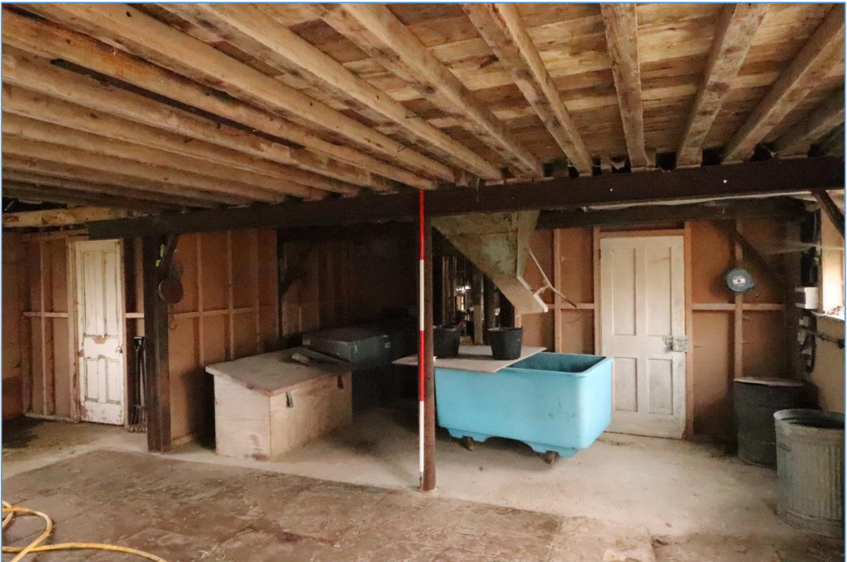
Plate 30. Interior of the southern bay of Building B, looking south-east.
