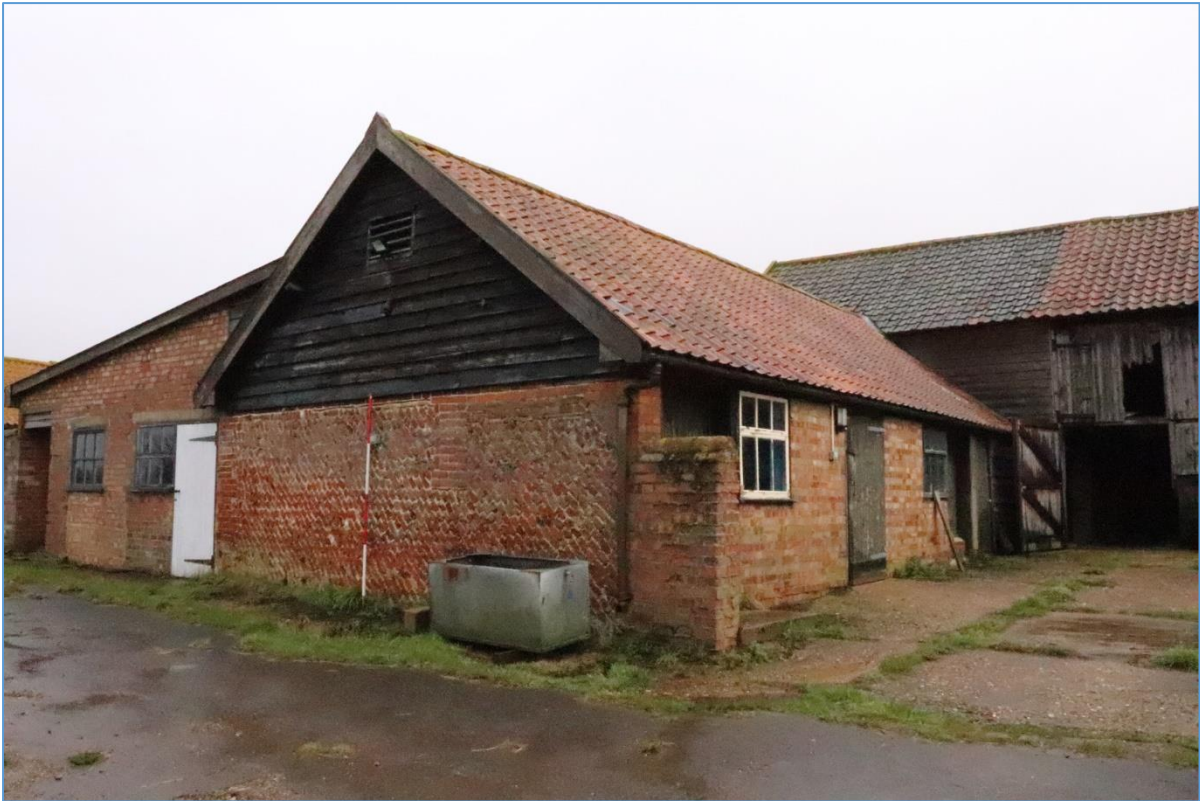
Plate 39. The western elevation of Building D, looking north-east.
