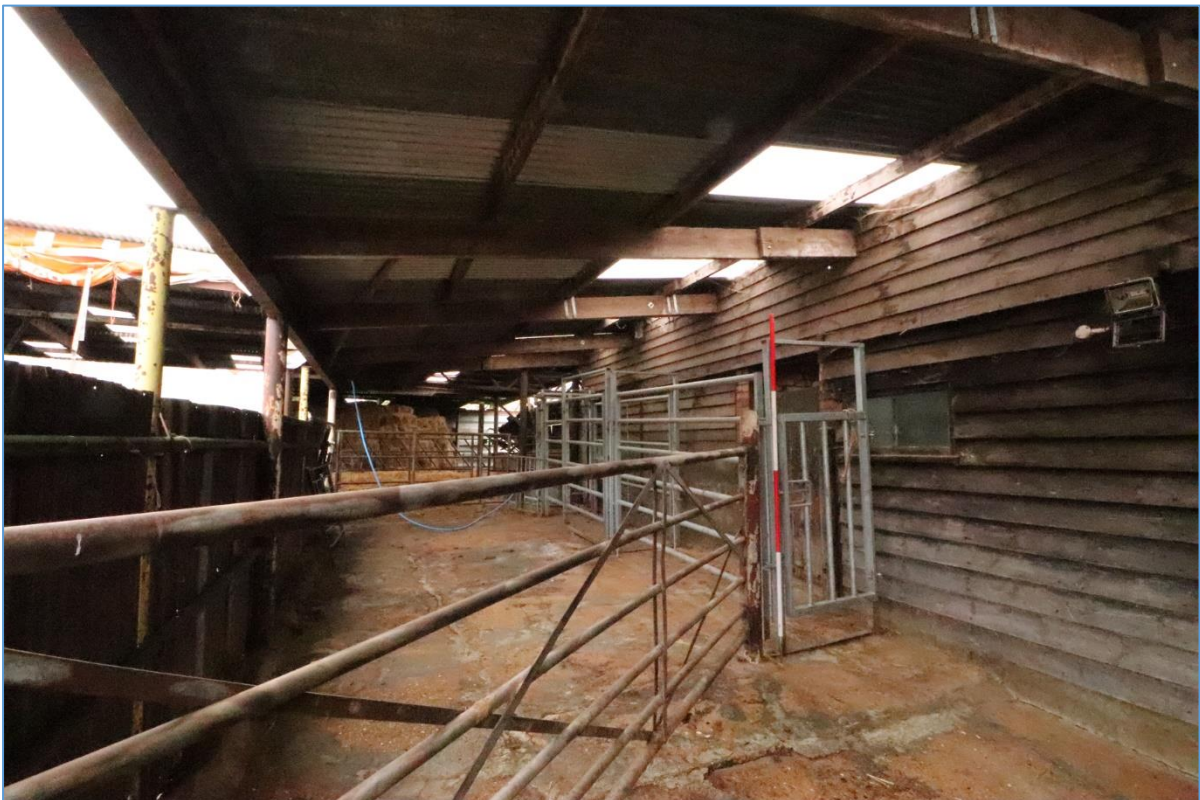
Plate 44: Interior of Building D, looking east.
