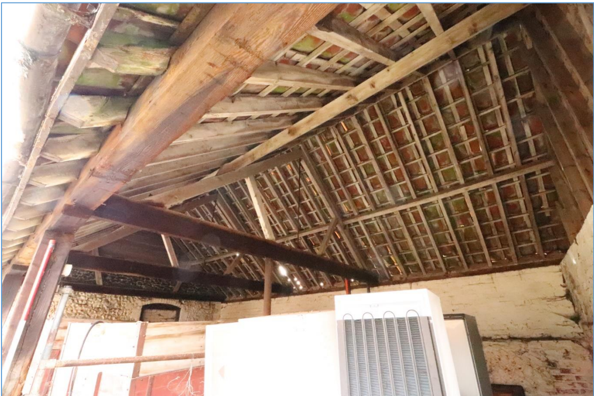
Plate 60. Interior of the northern part of Building F, looking south-west.
