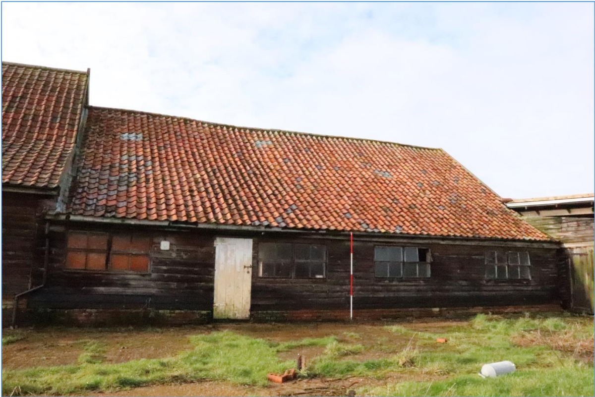
Plate 21. The eastern elevation of Building B, looking west.
