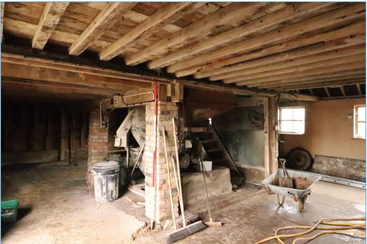
Plate 28. Interior of the northern bay of Building B, looking north-east.
