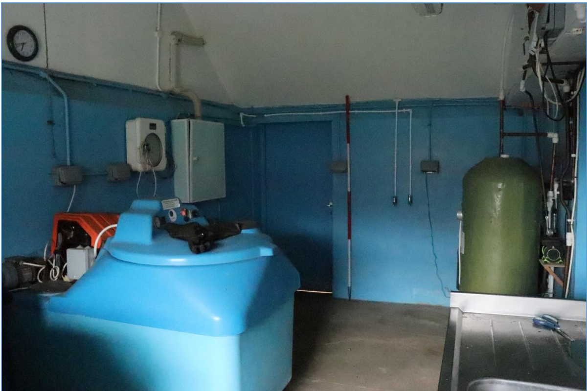
Plate 46. Interior of the milk treatment room of Building D, looking north-west.
