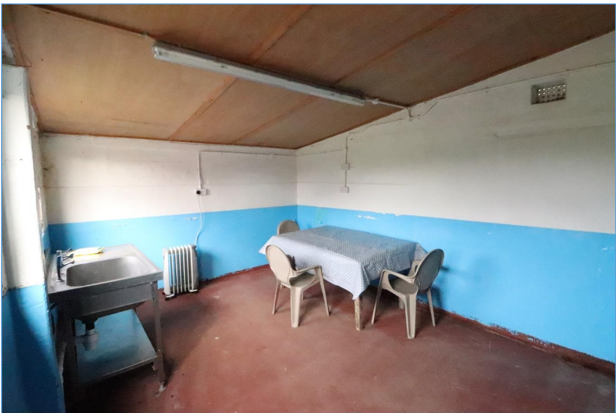
Plate 50. Interior of the former dairy in Building D, looking north-east.
