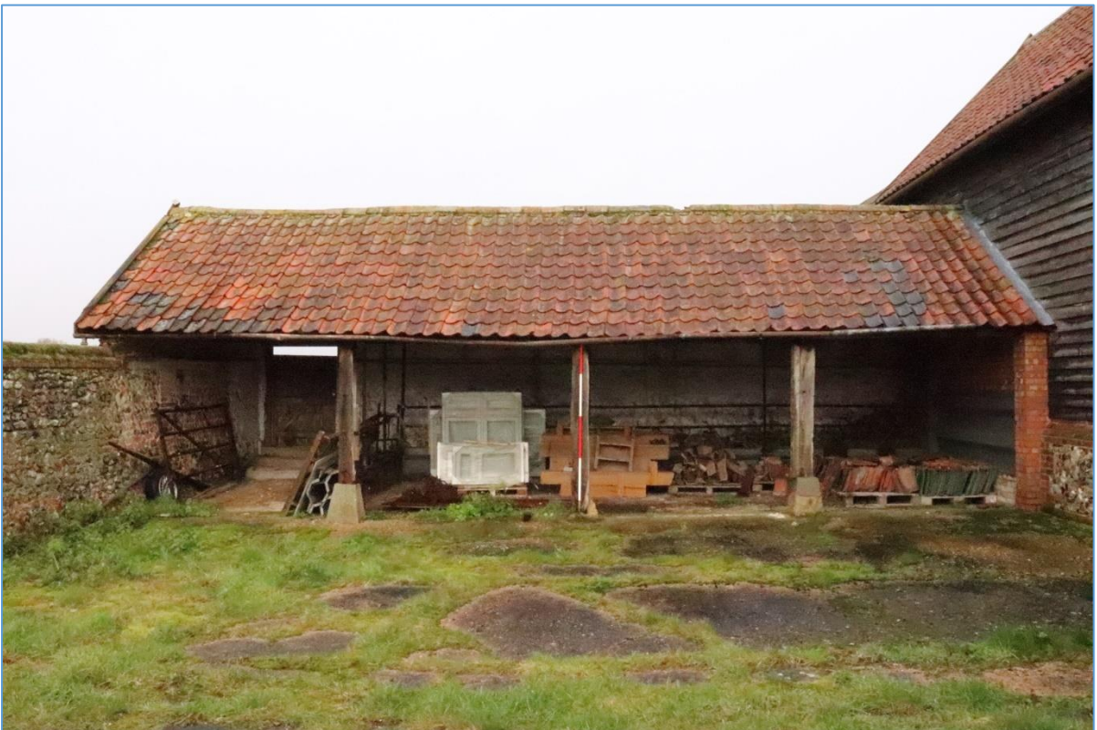
Plate 34. The southern elevation of Building C, looking north.
