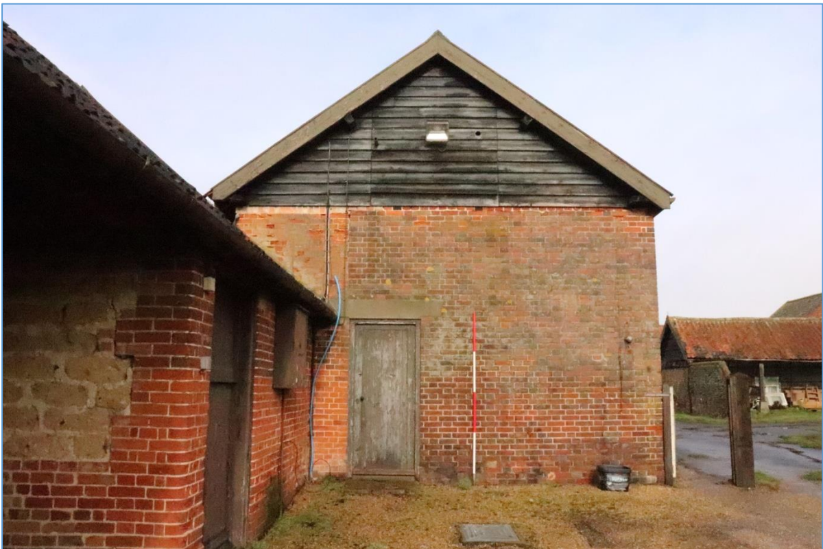
Plate 58 The southern elevation of Building F, looking north.
