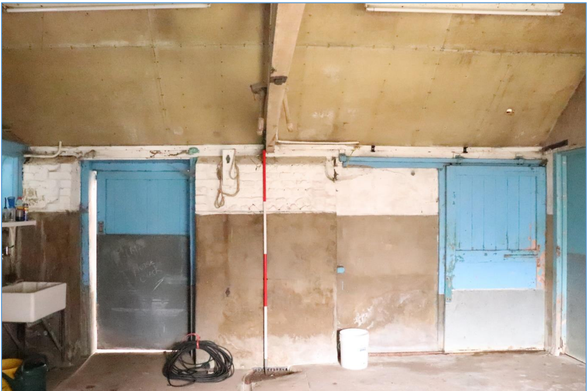
Plate 48. Interior of the former milking parlour in Building D, looking north.
