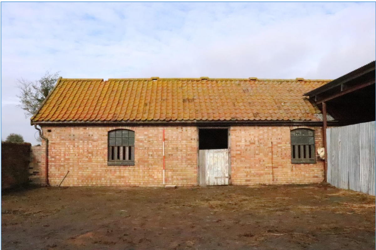
Plate 70. The southern elevation of Building G, looking north.
