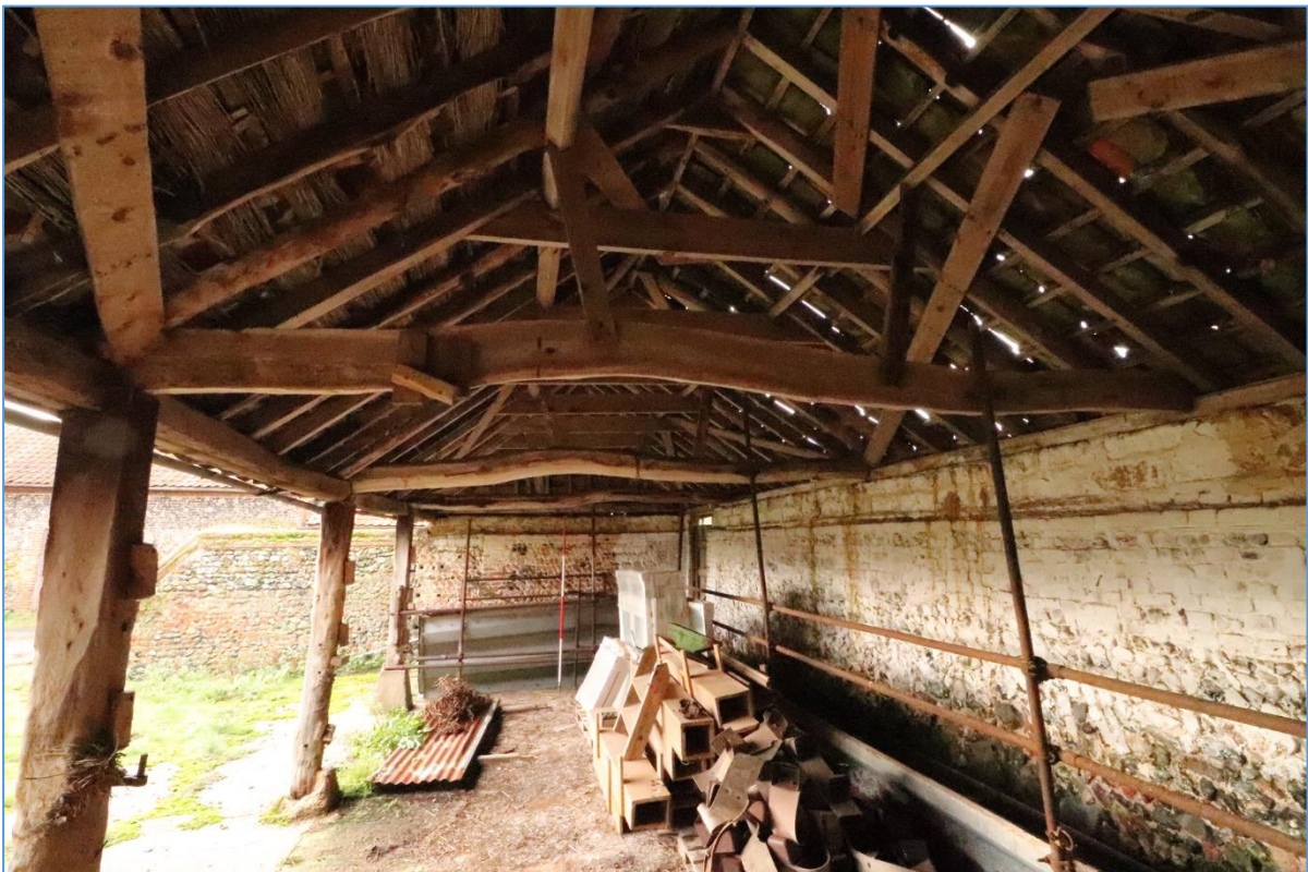
Plate 38. Interior of Building C, looking west.
