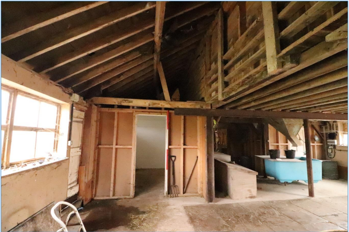
Plate 31. Interior of the eastern aisle of Building B, looking south.
