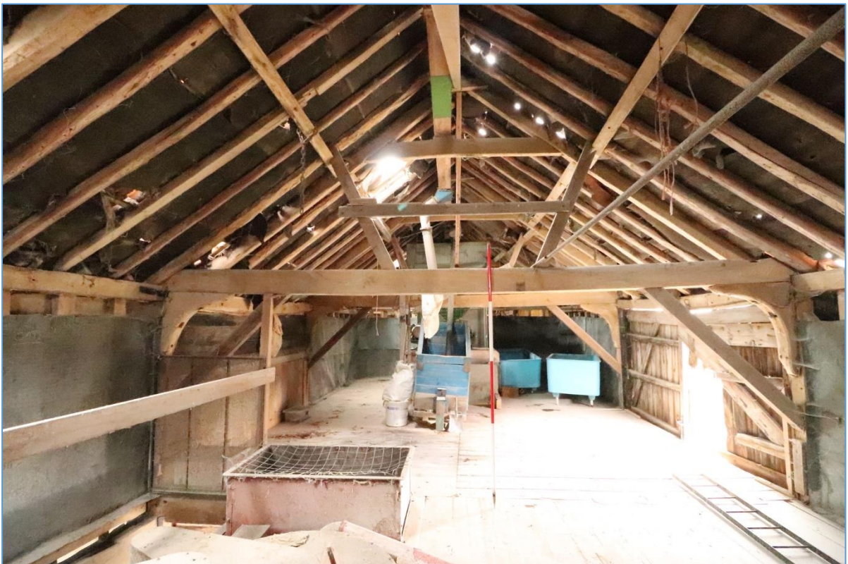
Plate 32. Interior of the first floor of Building B, looking south.
