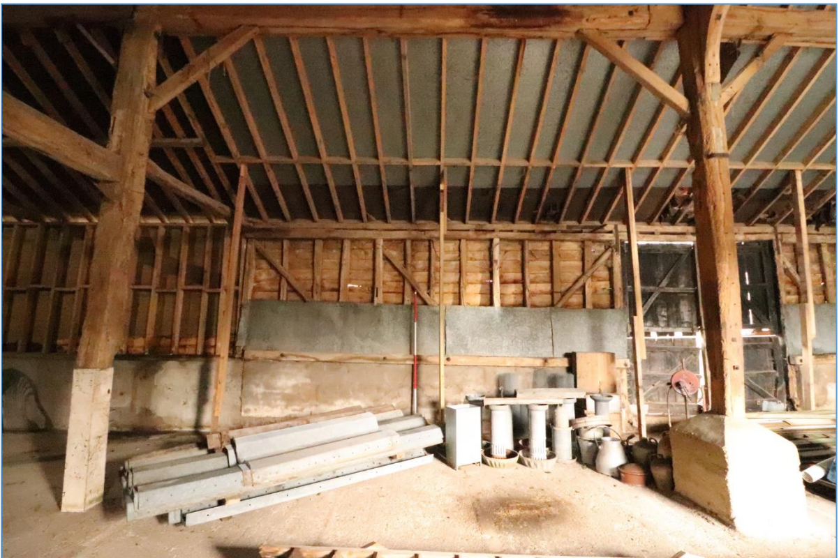
Plate 18. Interior of the northern bay of Building A, looking east.
