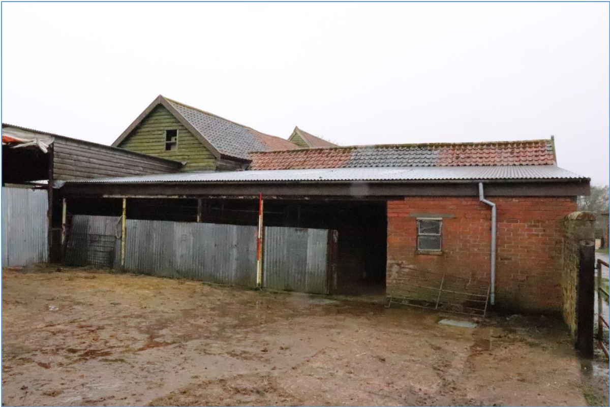
Plate 43: The northern elevation of Building D, looking south-east.
