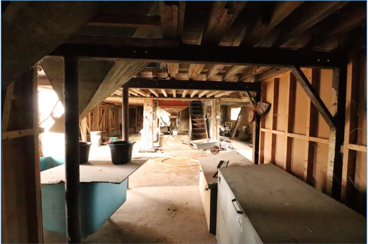
Plate 23. Interior of Building B, looking north.
