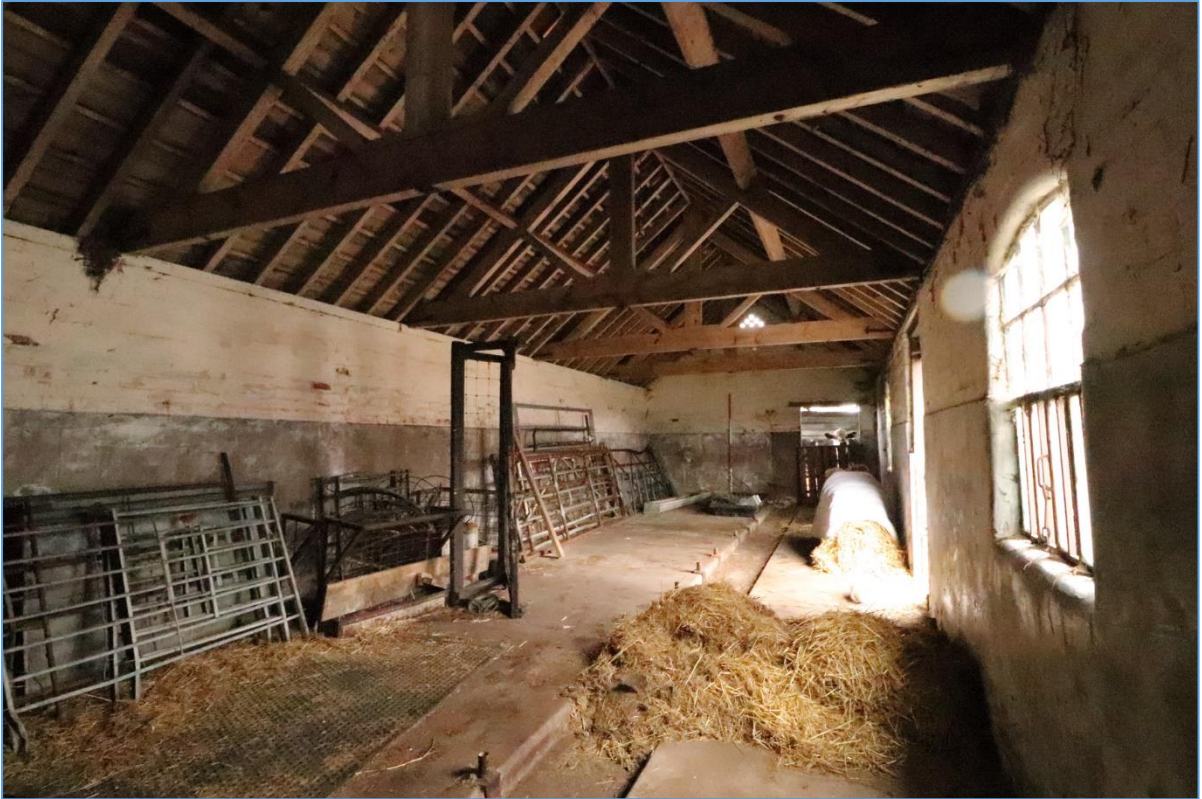
Plate 73. Interior of Building G, looking east.
