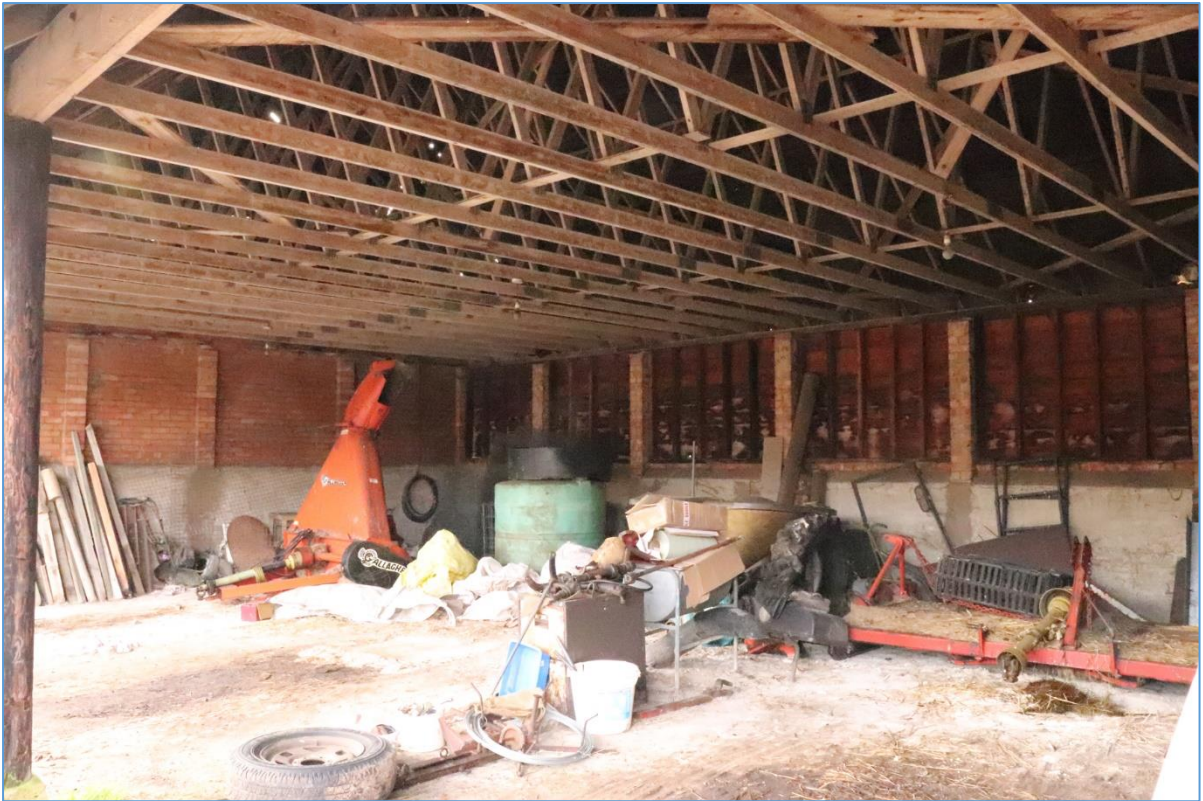
Plate 77. Interior of Building H, looking south-west.
