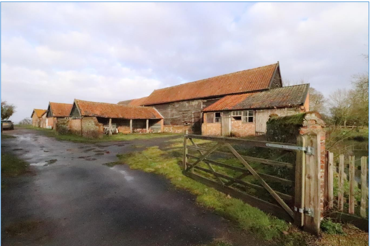
Plate 2. General view of the farm complex, looking north-east.
