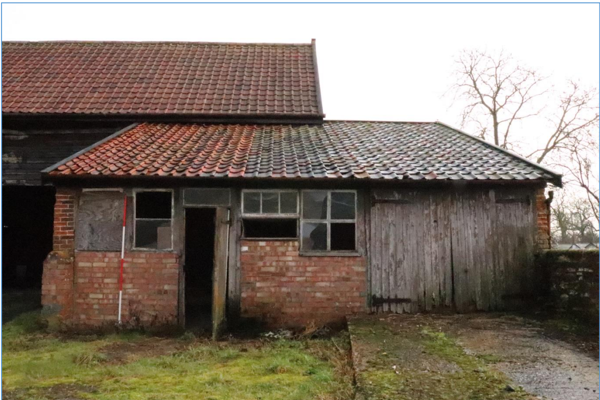
Plate 8. The western elevation of Building A's southern-western lean-to, looking east.
