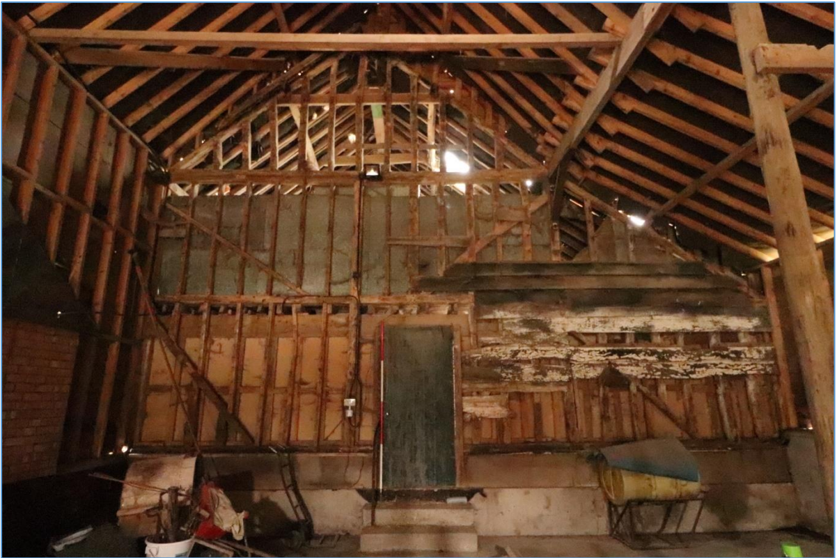
Plate 55. Interior of Building E, looking north.
