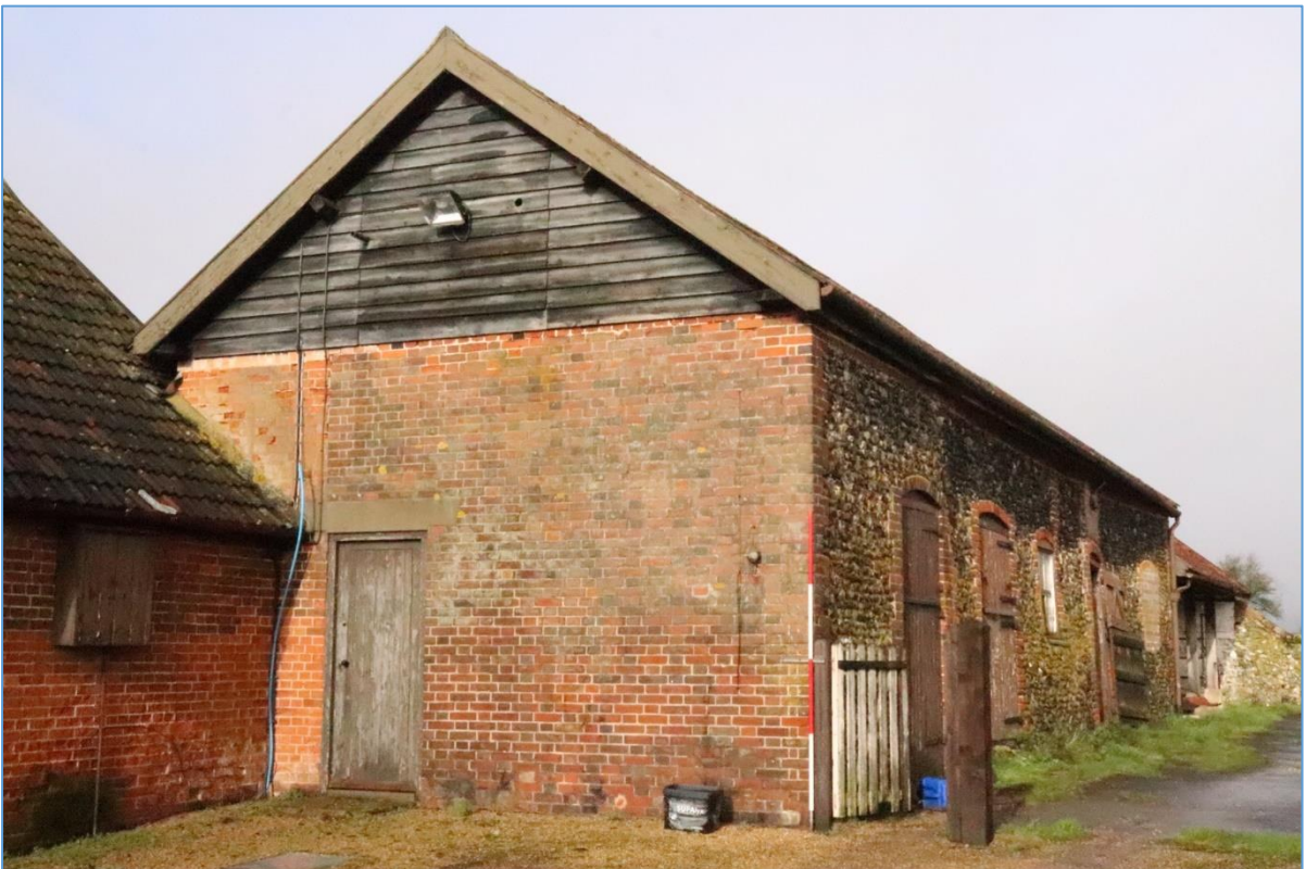
Plate 56. The southern elevation of Building F, looking north-west.
