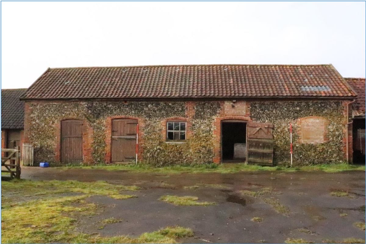
Plate 57. The eastern elevation of Building F, looking west.
