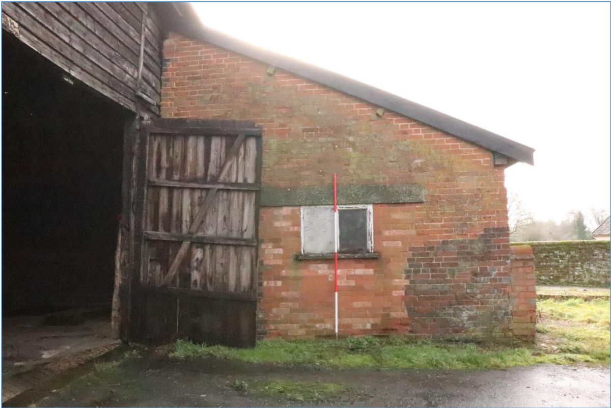
Plate 7. The northern elevation of Building A's southern-western lean-to, looking south.
