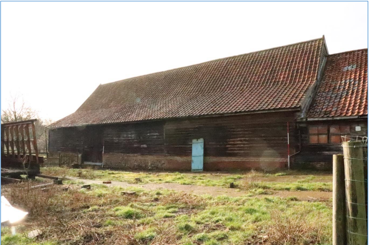
Plate 52. The eastern elevation of Building E and Building A, looking south-west.
