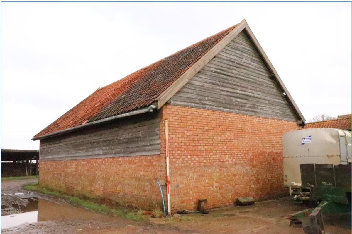
Plate 76. The western and southern elevations of Building H, looking north-east.
