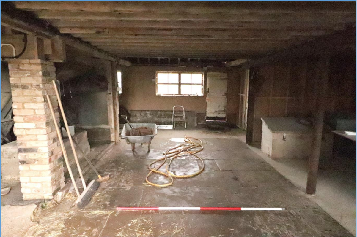
Plate 29. Interior of the central bay of Building B, looking east.
