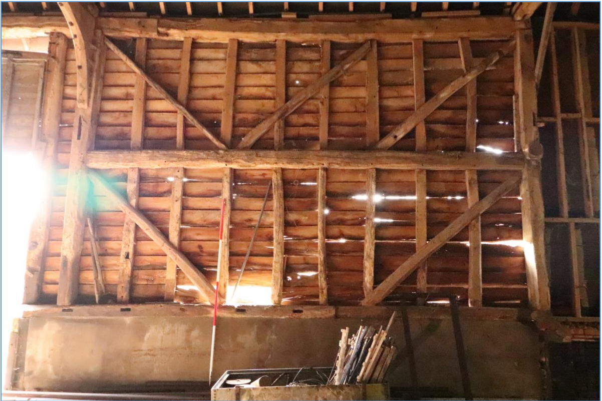
Plate 19. Interior of the northern bay of Building A, looking west.
