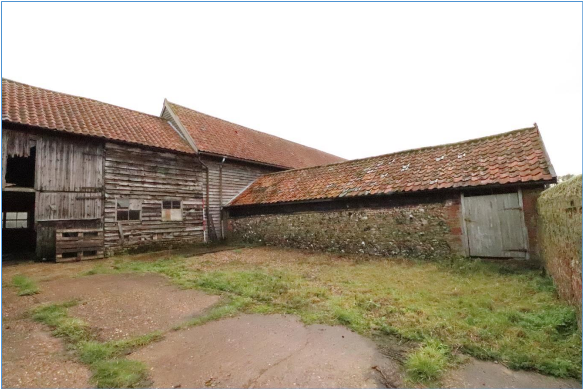
Plate 37. The northern elevation of Building C, looking south-east.
