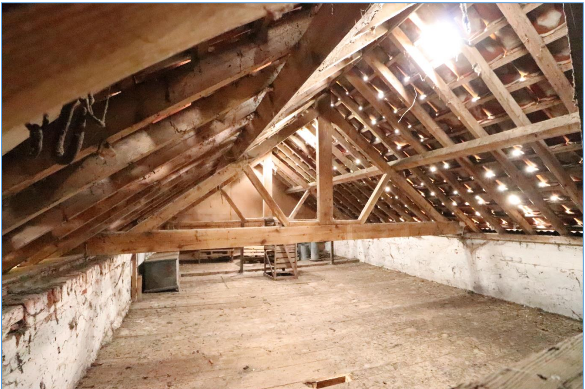
Plate 68. Interior of the first-floor of Building F, looking south.
