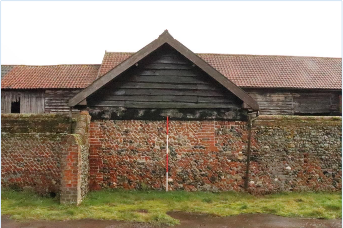
Plate 35. . The western elevation of Building C, looking east.
