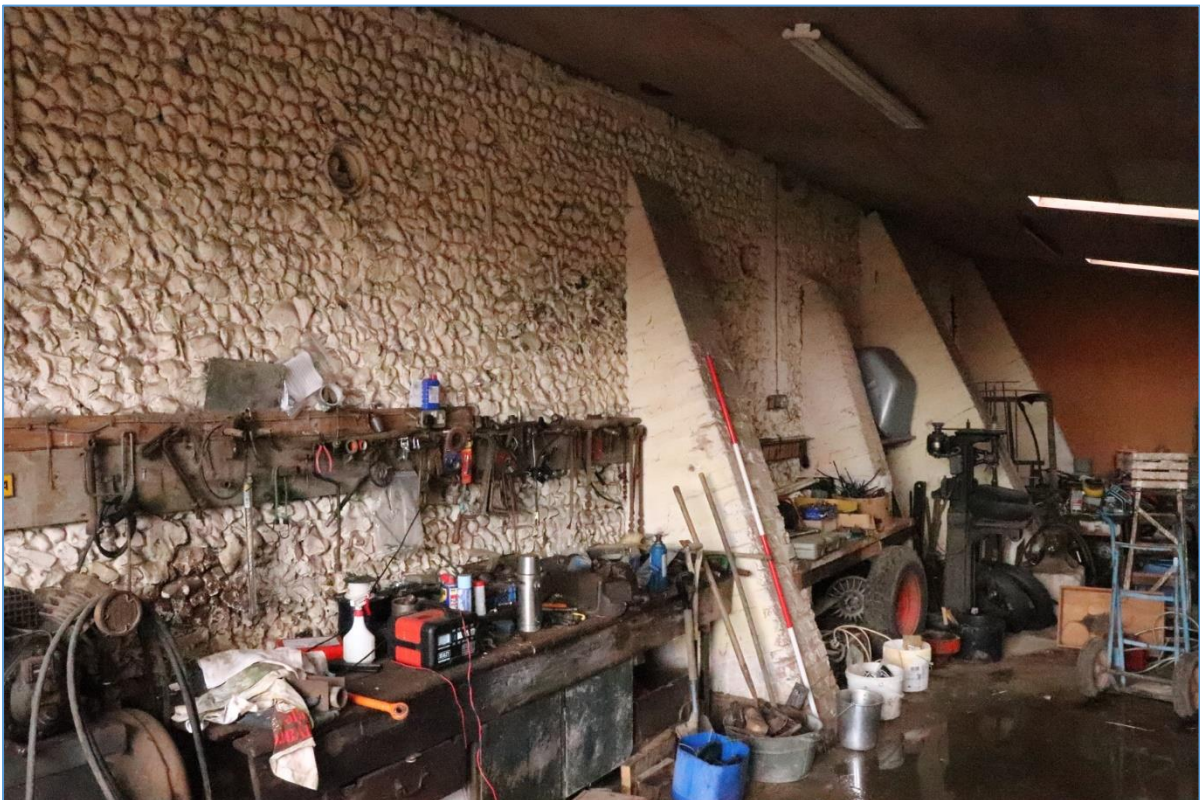
Plate 64. Interior of Building F's lean-to extension, looking south-east.
