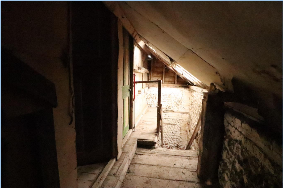
Plate 69. Interior of the first-floor of Building F, looking south.
