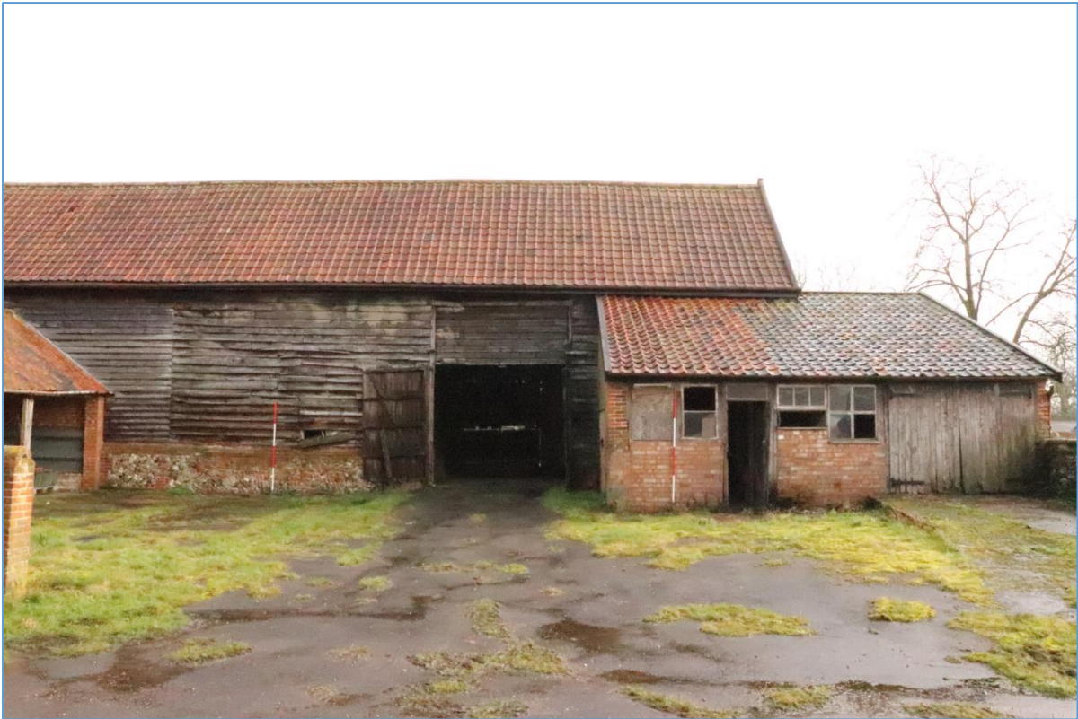
Plate 5. The western elevation of Building A, looking east.
