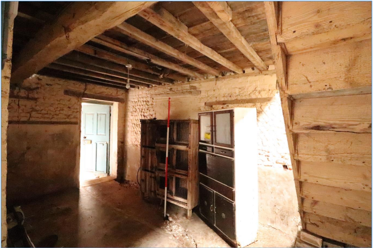
Plate 67. Interior of Building F, northern end, looking north-west.
