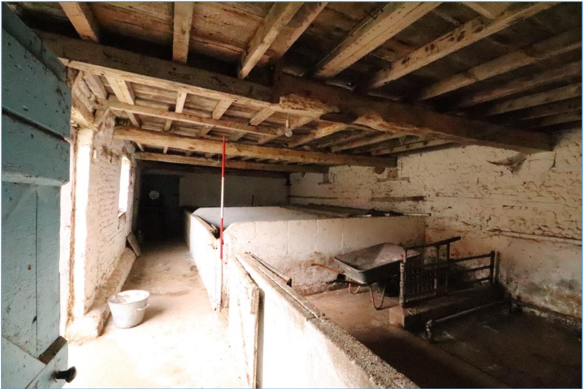
Plate 65. Interior of Building F, looking south.
