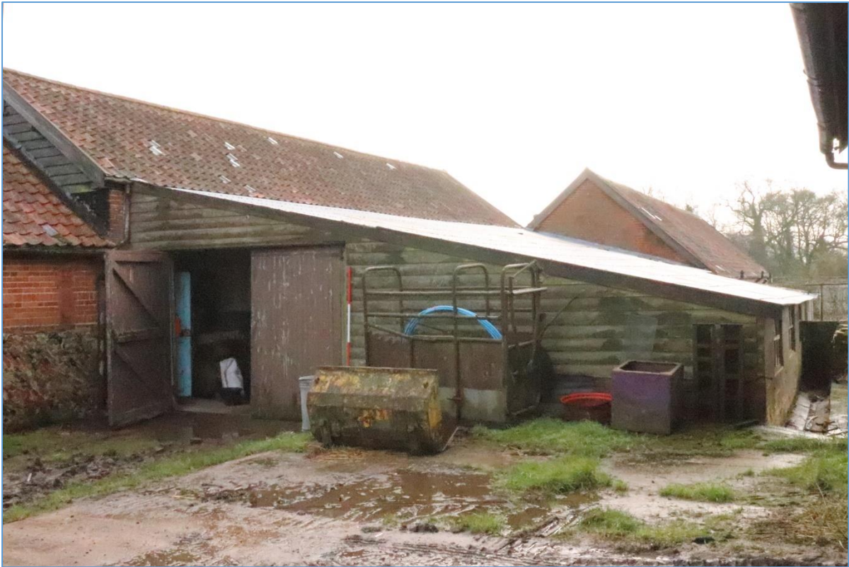
Plate 63. The northern elevation of Building F's lean-to extension, looking south.
