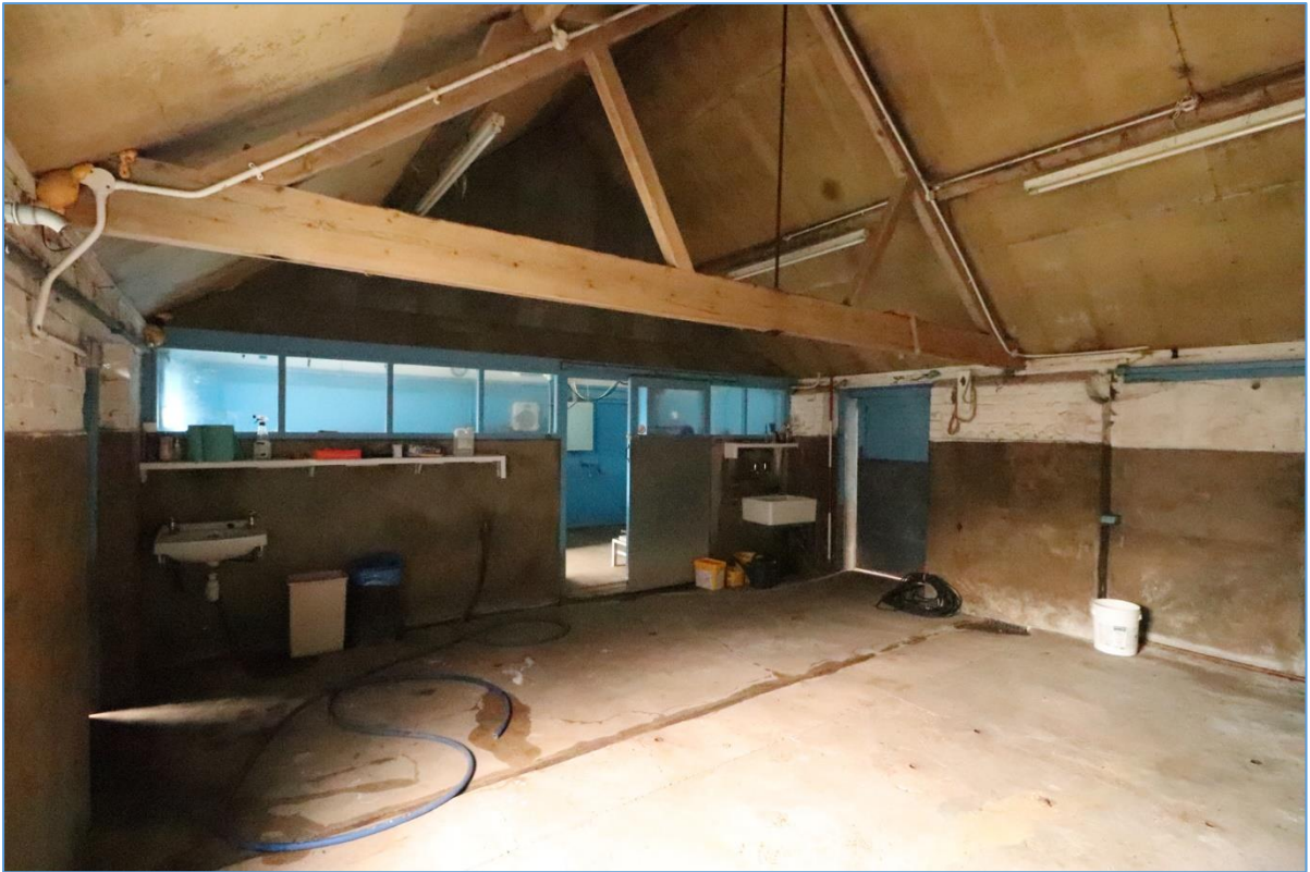
Plate 47. Interior of the former milking parlour in Building D, looking north-west.
