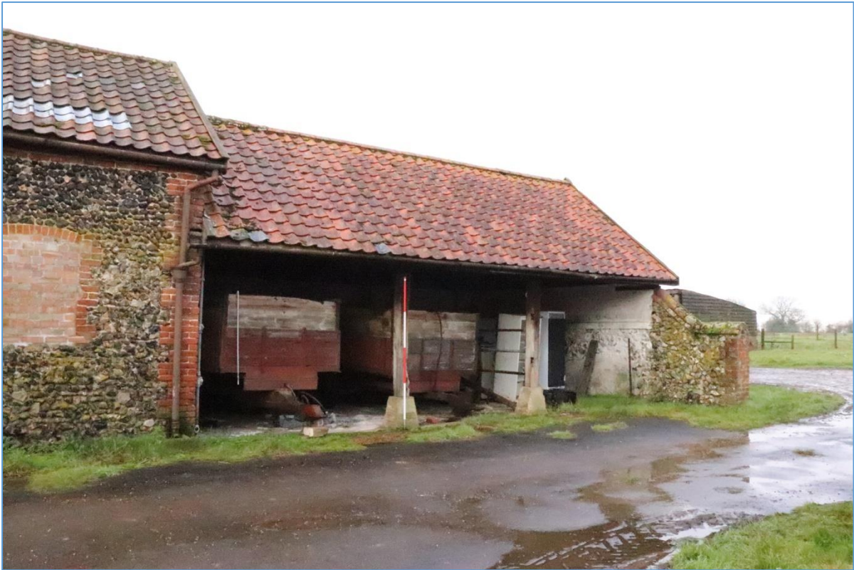
Plate 59. The eastern elevation of Building F, looking north-west.
