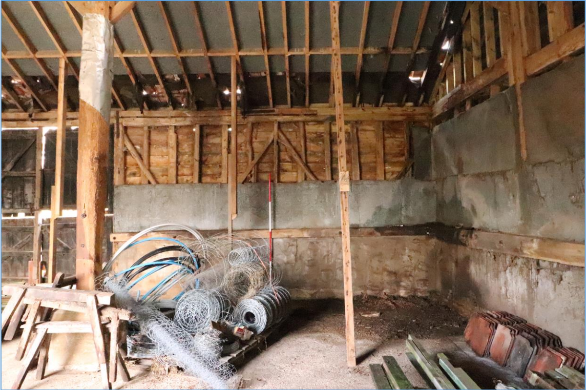
Plate 15. Interior of the southern bay of Building A, looking east.
