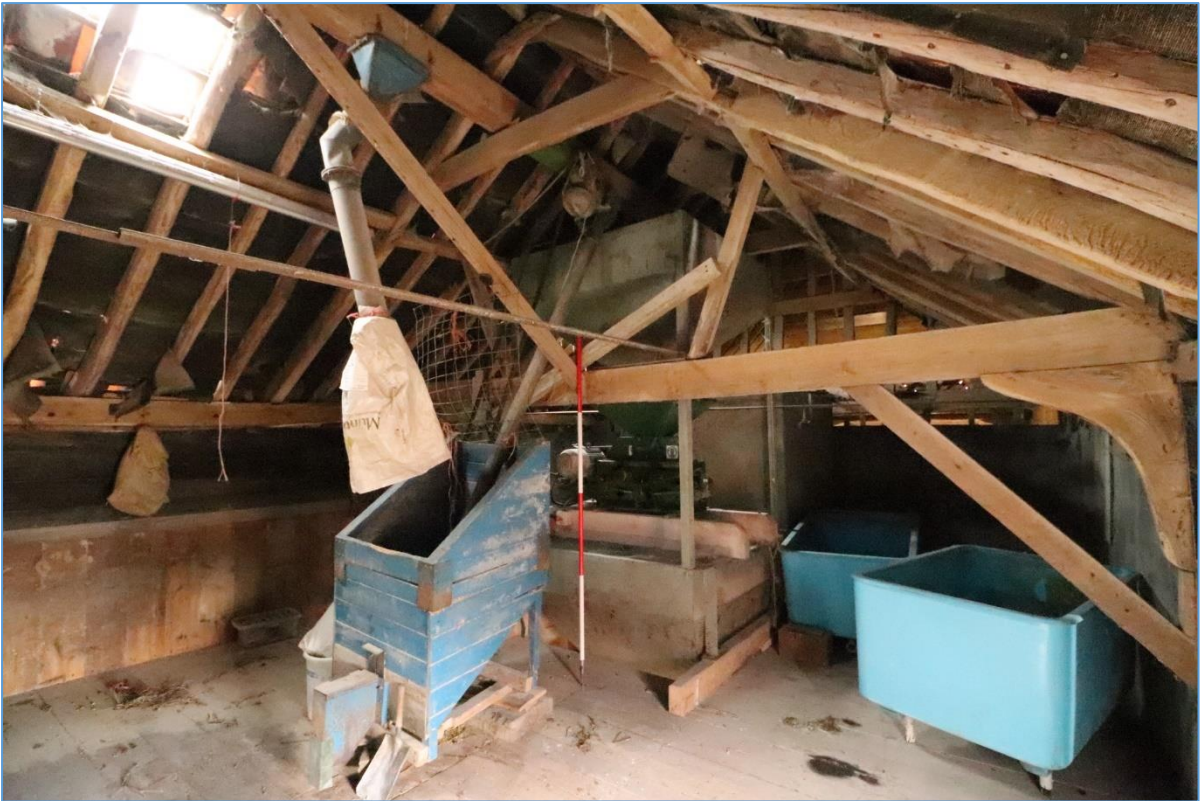
Plate 33. Interior of the first floor of Building B, looking south-east.
