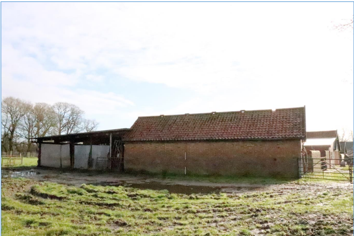
Plate 72. The northern elevation of Building G, looking south-east.
