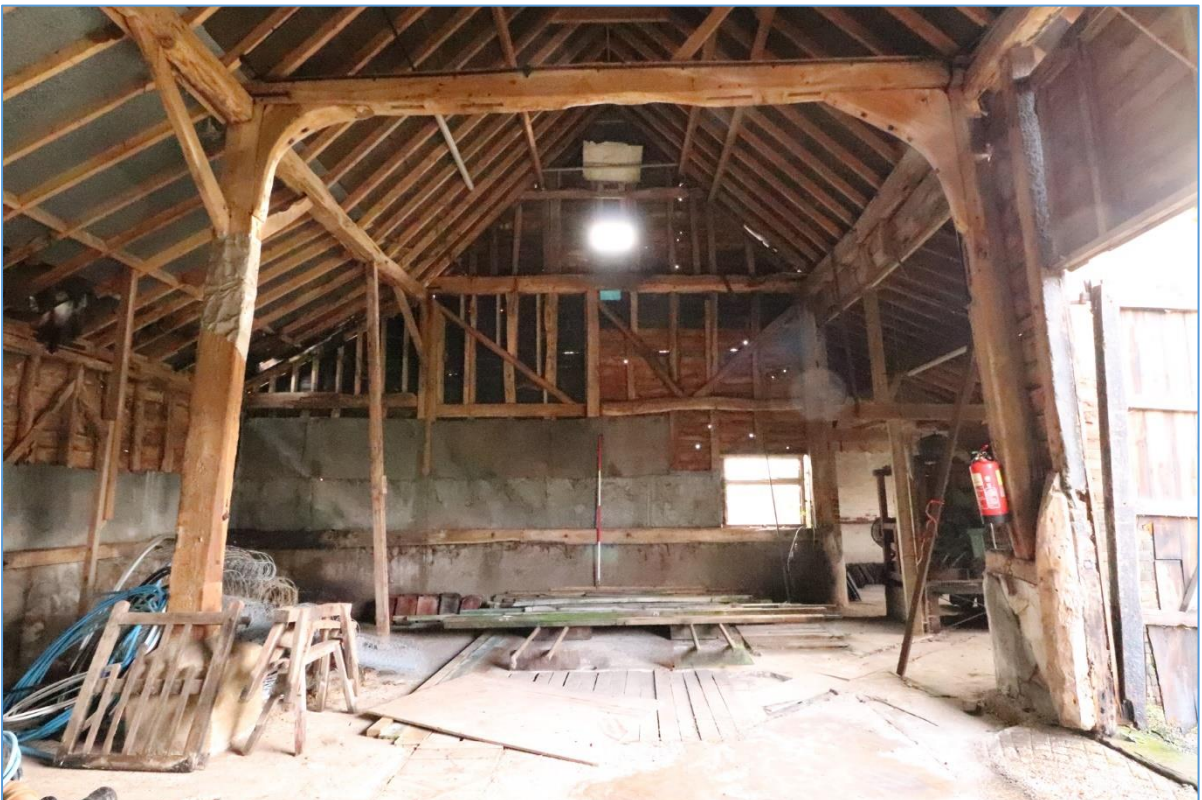
Plate 14. The interior of the southern bay of Building A, looking south.
