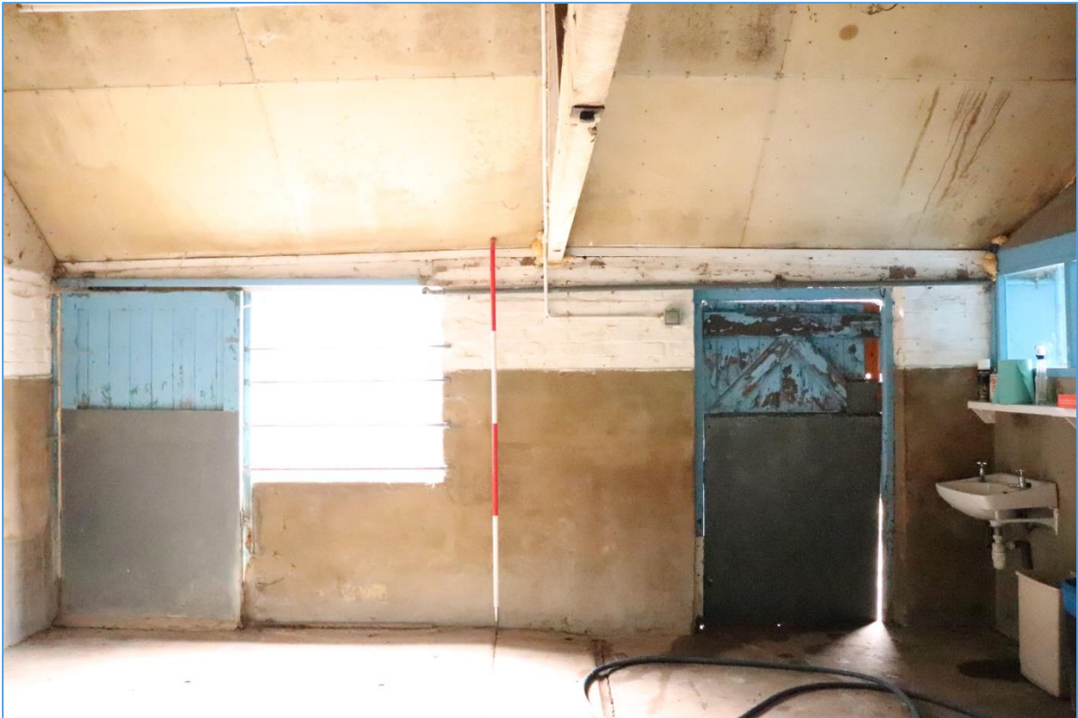
Plate 49. Interior of the former milking parlour in Building D, looking south.
