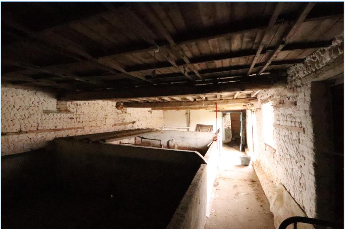
Plate 66. Interior of Building F, looking north.
