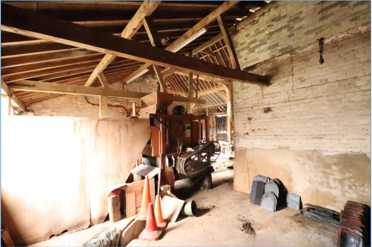
Plate 11. The interior of Building A's south-western lean-to, looking north-east.
