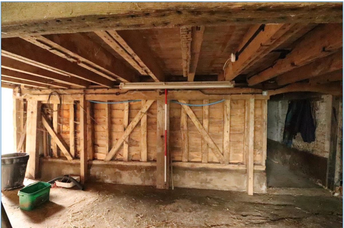
Plate 24. Interior of the northern bay of Building B, looking west.
