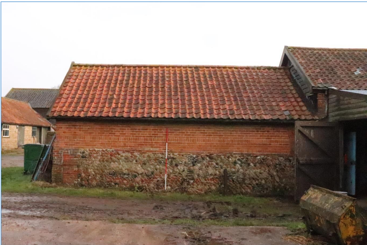
Plate 62. The western elevation of Building F, looking east.
