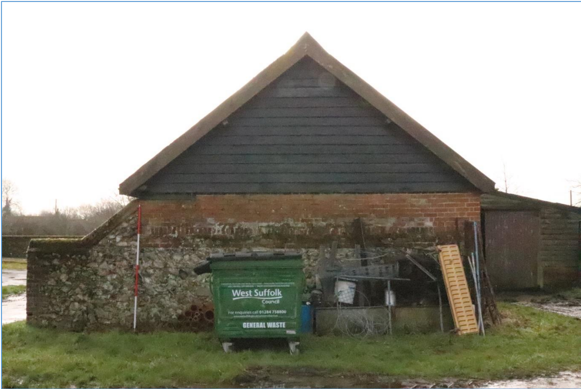
Plate 61. The northern elevation of Building F, looking south.
