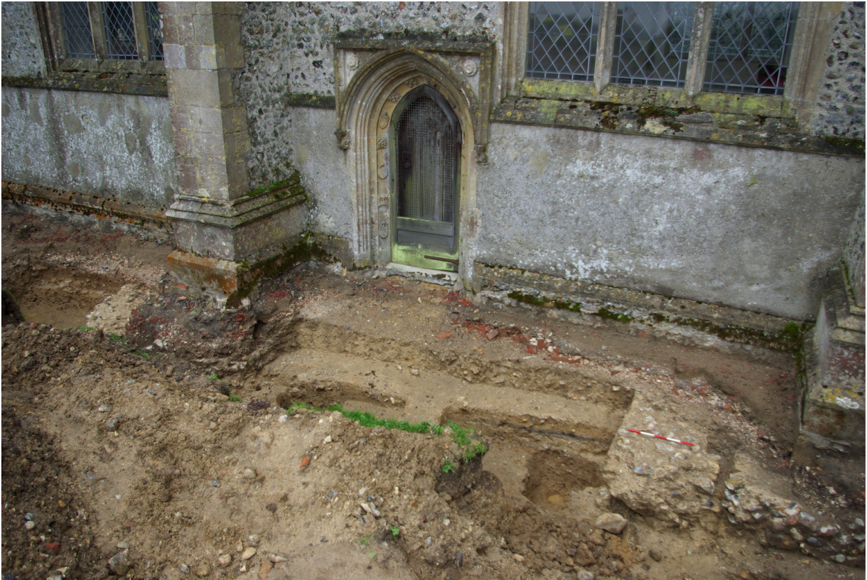
Plate 1: Walls 57 (to left) and 11 with construction and demolition layers, looking S, 0.5m scale
