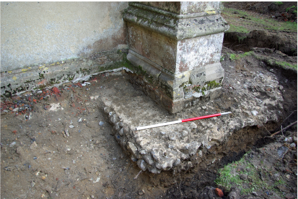
Plate 6: S transept SW buttress with footing 76, looking SE, 1m scale
