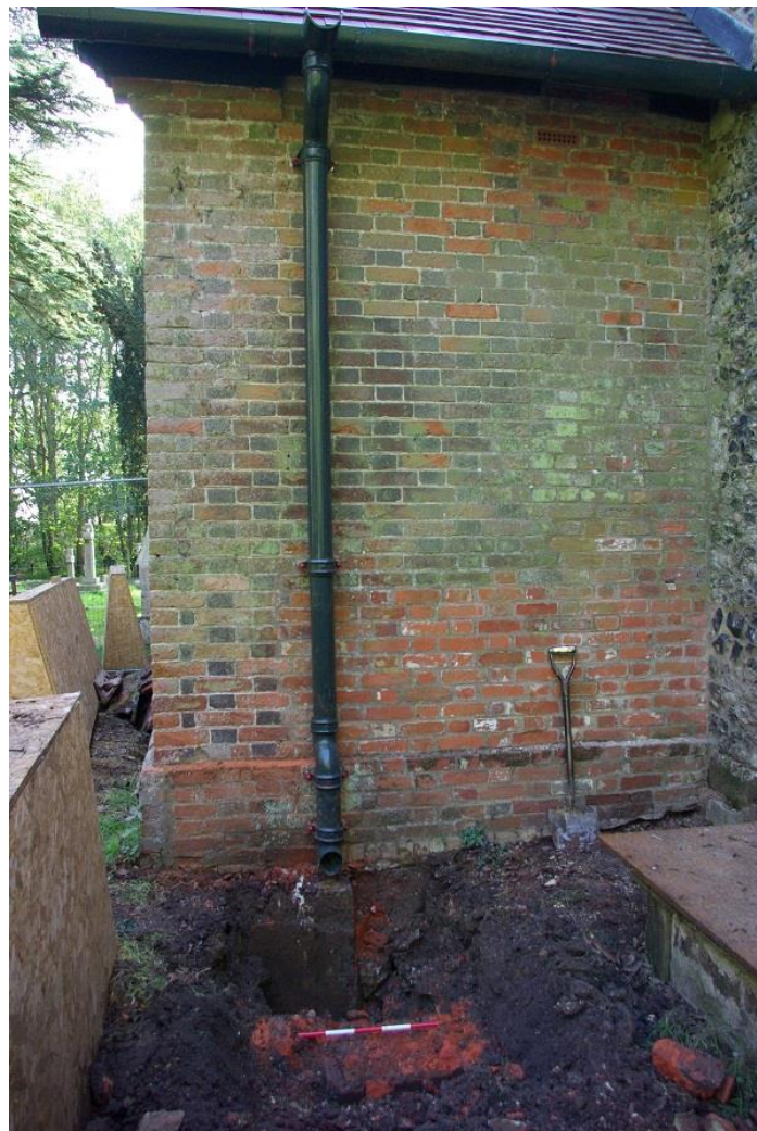
Plate 5: Gully trench 5 with brick wall 6 (0.50m scale), looking S and new brickwork in chancel wall visible
