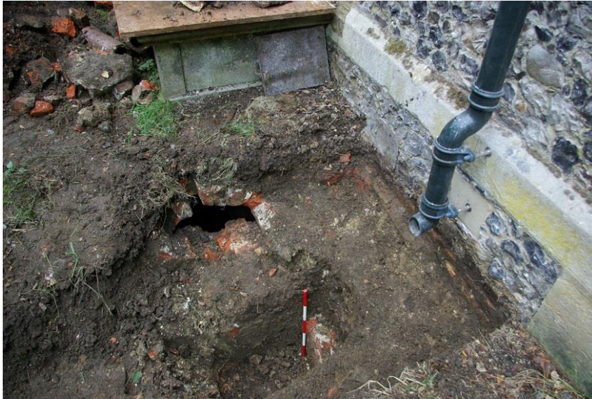
Plate 4: Gully trench 4 with brick feature 15 (0.5m scale) and showing damage to vaulted structure 16, looking SSW
