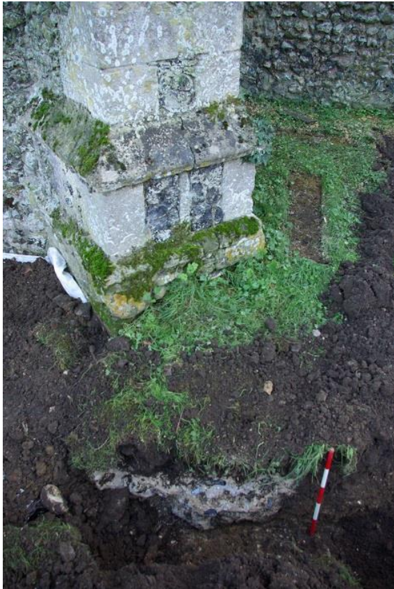
Plate 3: NW nave corner buttress and footing [17], looking S, 0.5m scale
