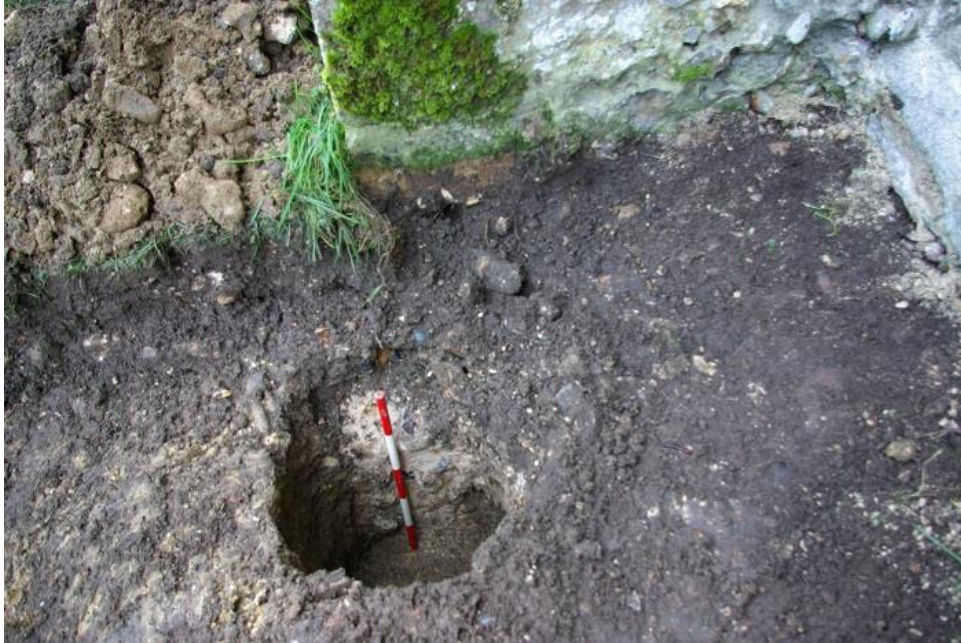
Plate 6: N nave buttress footing, [8], looking E, 0.5m scale
