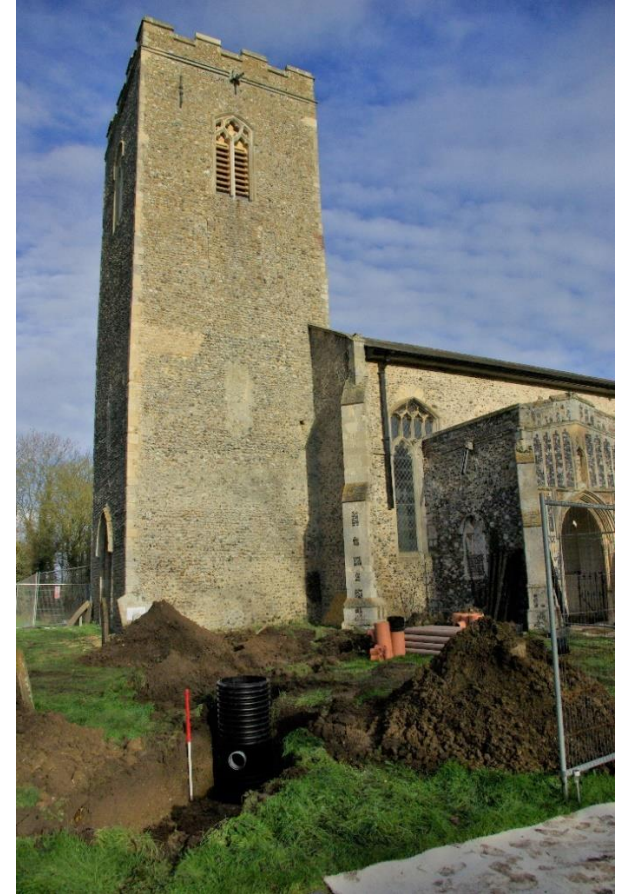
Plate 10: Soakaway trench [14], looking NNE,..... 1m scale
