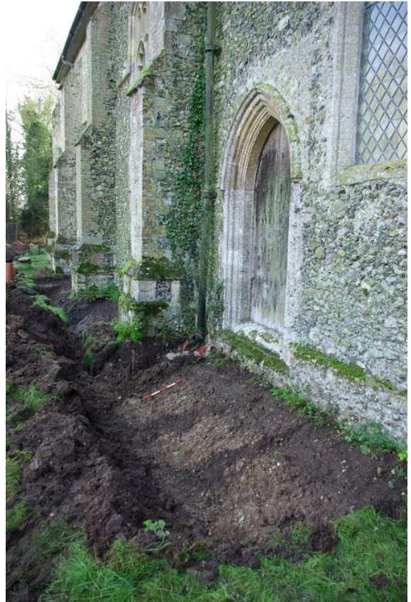
Plate 4: N nave, drain trench [1], looking E, 0.5m scale
