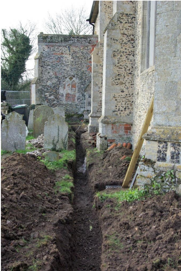
Plate 8: Drain [9], S of nave, looking W
