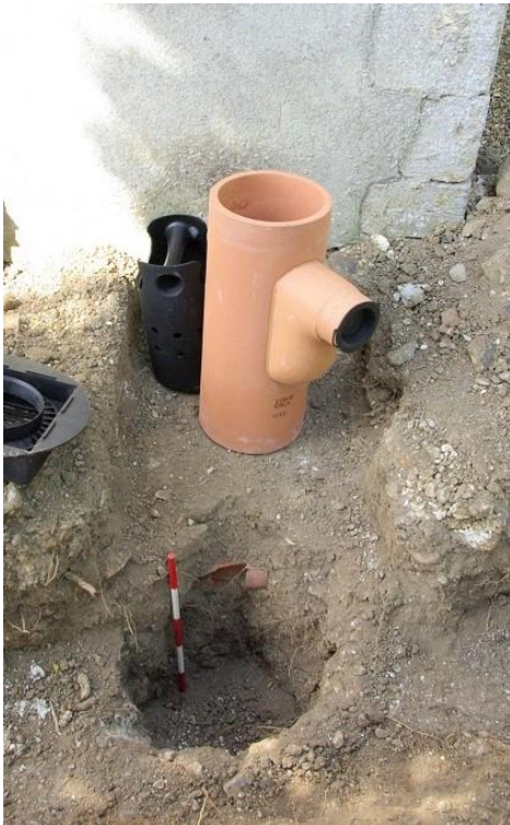
Plate 19: Trench 68, looking N, 0.5m scale
