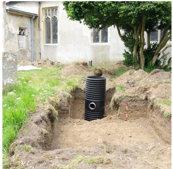
Plate 20: Trench 6, looking NW, 0.5m scale
