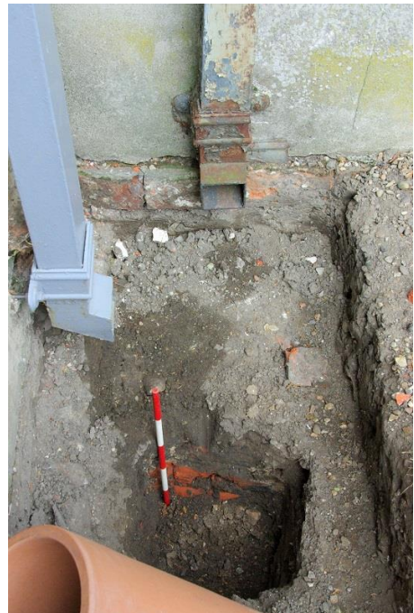
Plate 22: Trench 70, looking N, 0.5m scale
