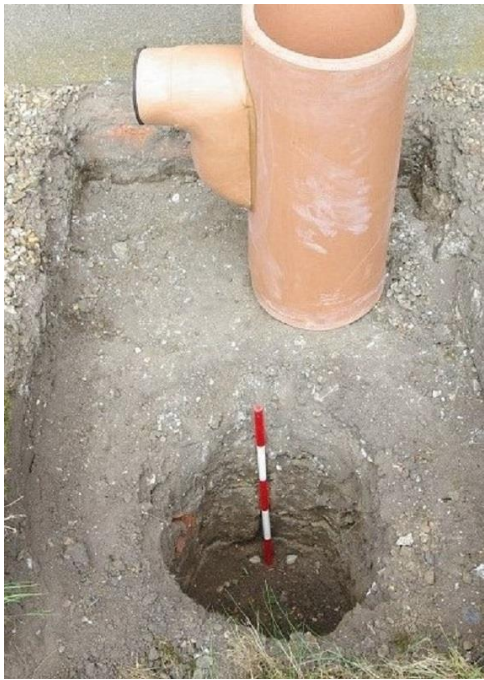
Plate 21 Trench 69, looking N, 0.5m scale
