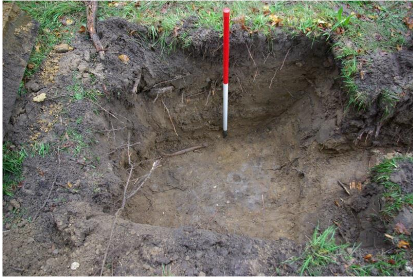
Plate 4: Trench 1 (soakaway), looking S, 1m scale
