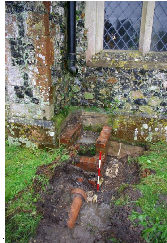
Plate 5: Trench 2, existing brick gully in situ , looking S. 0.5m scale
