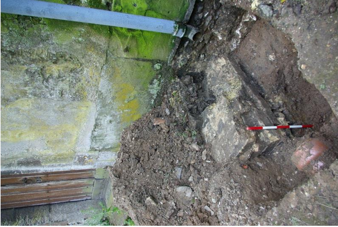
Plate 7: Trench 30, footing [31], looking S, 0.5m scale
