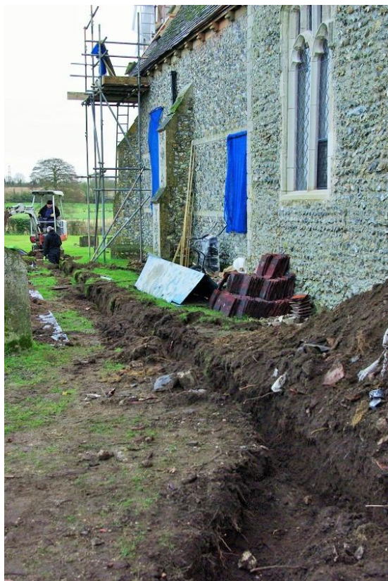
Plate 1: Drain trench N of church, looking E
