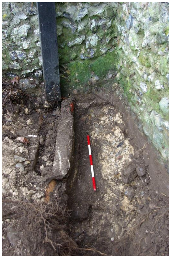
Plate 2: Trench [1], footing [2], looking S, 0.5m scale
