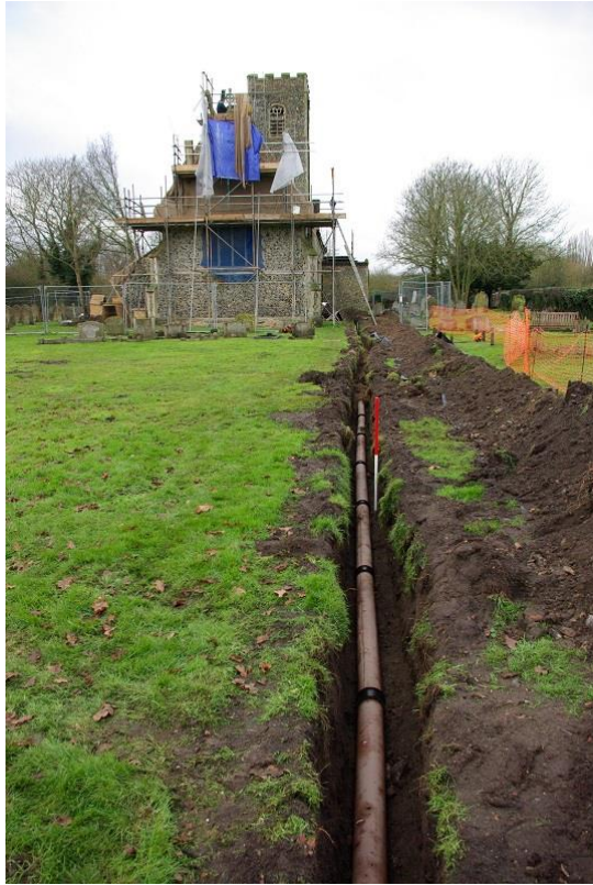
Plate 6: Drain E of church, looking W, 1m scale
