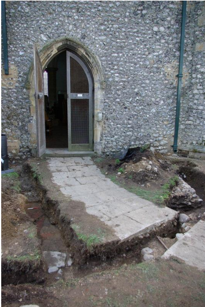
Plate 1: Wall [2]/[15], floor [12], looking S, 0.2m scale
