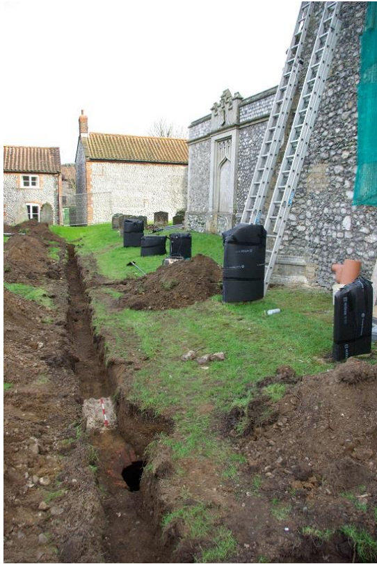
Plate 6: Wall [6], sunken churchyard path behind, looking E, 0.5m scale
