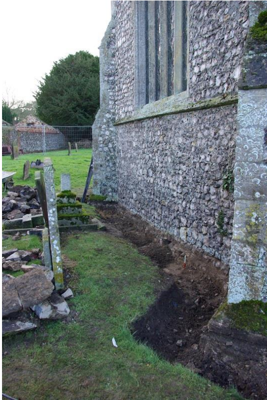
Plate 14: Chancel footing, looking SSE, 0.2m scale
