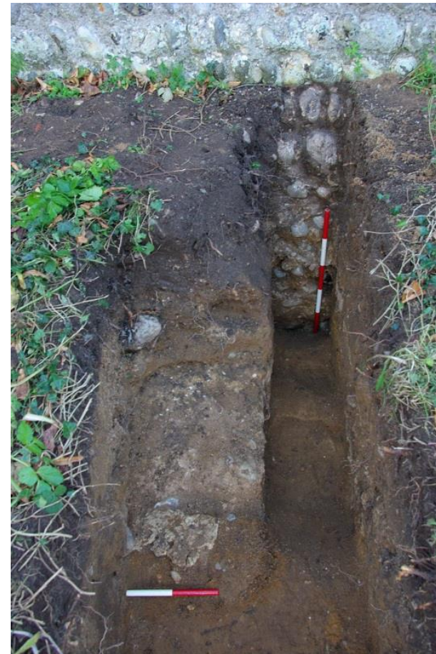
Plate 3: Opening-up trench 2; mortar [17] with underlying sand [18], N aisle footing exposed, looking S, 0.5m and 0.2m scales
