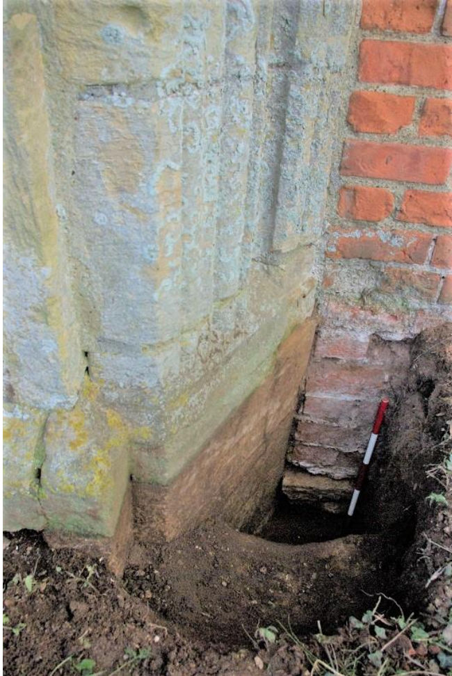
Plate 13: Former threshold at blocked W door, looking E, 0.5m scale
