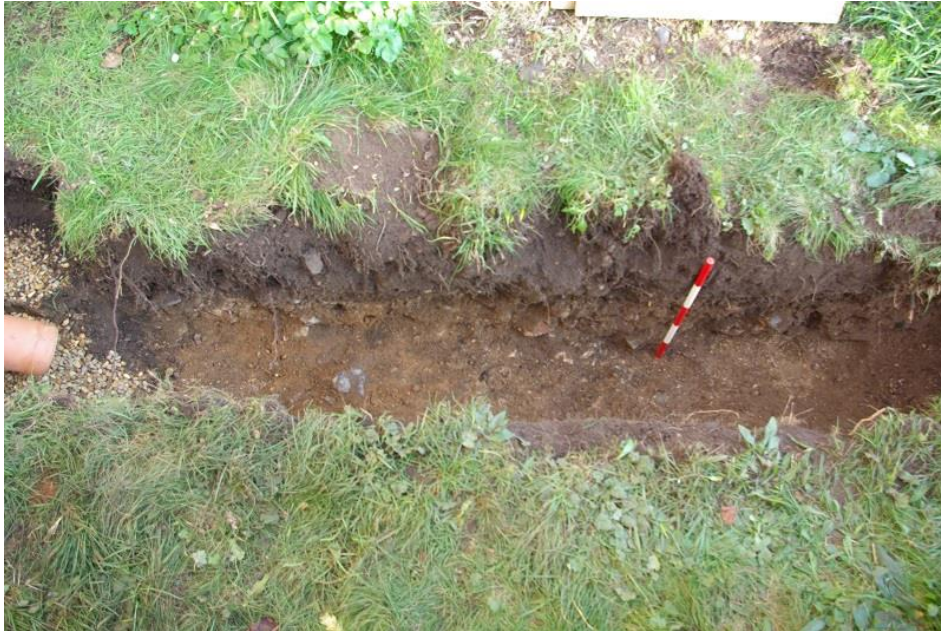
Plate 8: Drain trench S of trench 46; orange sand overlaid by mortar (left) rubble [67] (central) looking E, 0.5m scale
