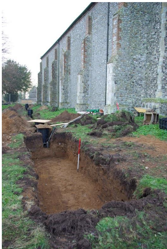
Plate 10: Trench 45; looking E, 1m scale
