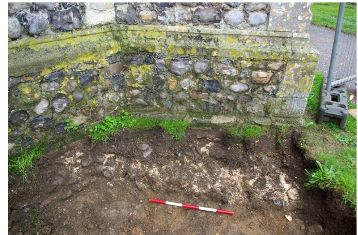
Plate 9: Trench 20, butress and tower footings, looking WSW, 0.5m scale
