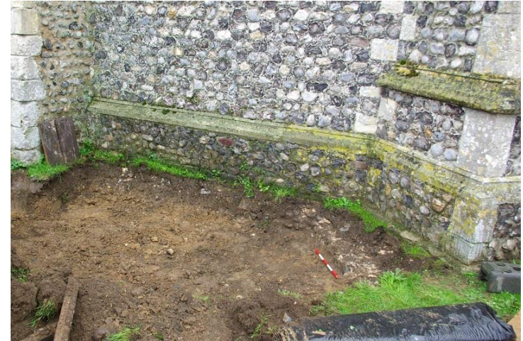
Plate 8: Trench 20, butress footing, looking SSE, 0.5m scale
